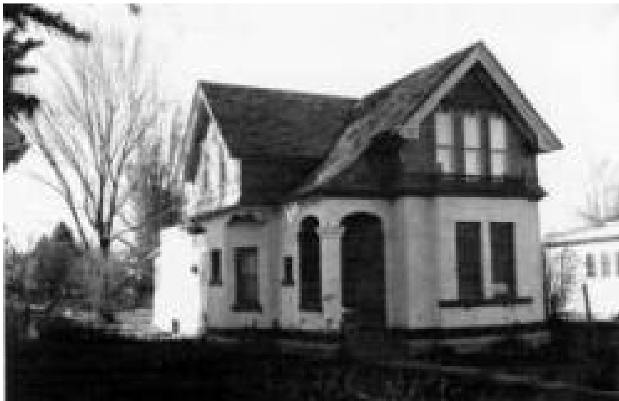
Figure 9: South side (left) and east façade, camera facing northwest. Photo taken by Larimer County Assessor, 1967. Shows brick portion of house painted white. Wall on south side west of bay is unclear, but might be the south porch shown in the 1948 photo. To the west is the wood back porch that was removed in 1978. Otherwise materials and details match house today. Original archived at Local History Archive, Fort Collins Museum of Discovery. Available online at http://database.history.fcgov.com/cdm/search/?collection=ph&searchterm=121+n+grant .
