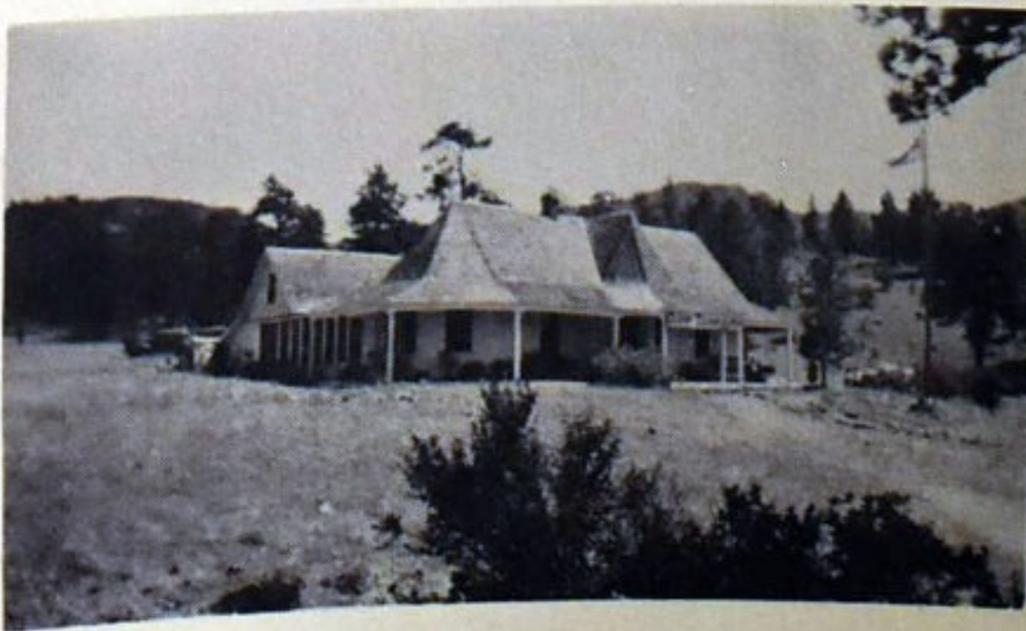
Figure 8: Photo from the 1950 Camp Dunraven brochure. Note that the north wall of the enclosed rear porch is flush with the north wall of the main house. (City of Greeley Museums, Hazel E. Johnson Research Center)
