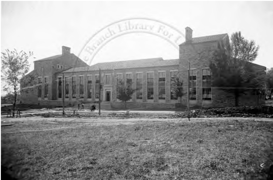
Figure 2: The 1921 Hellems Arts and Sciences Building was the first University of Colorado building designed by Charles Klauder in the "Colorado Style" after adoption of Klauder's campus master plan in 1918. Photograph dated May 1922. Boulder Historical Society Collection, Carnegie Library for Local History, BHS 240-2-30.
