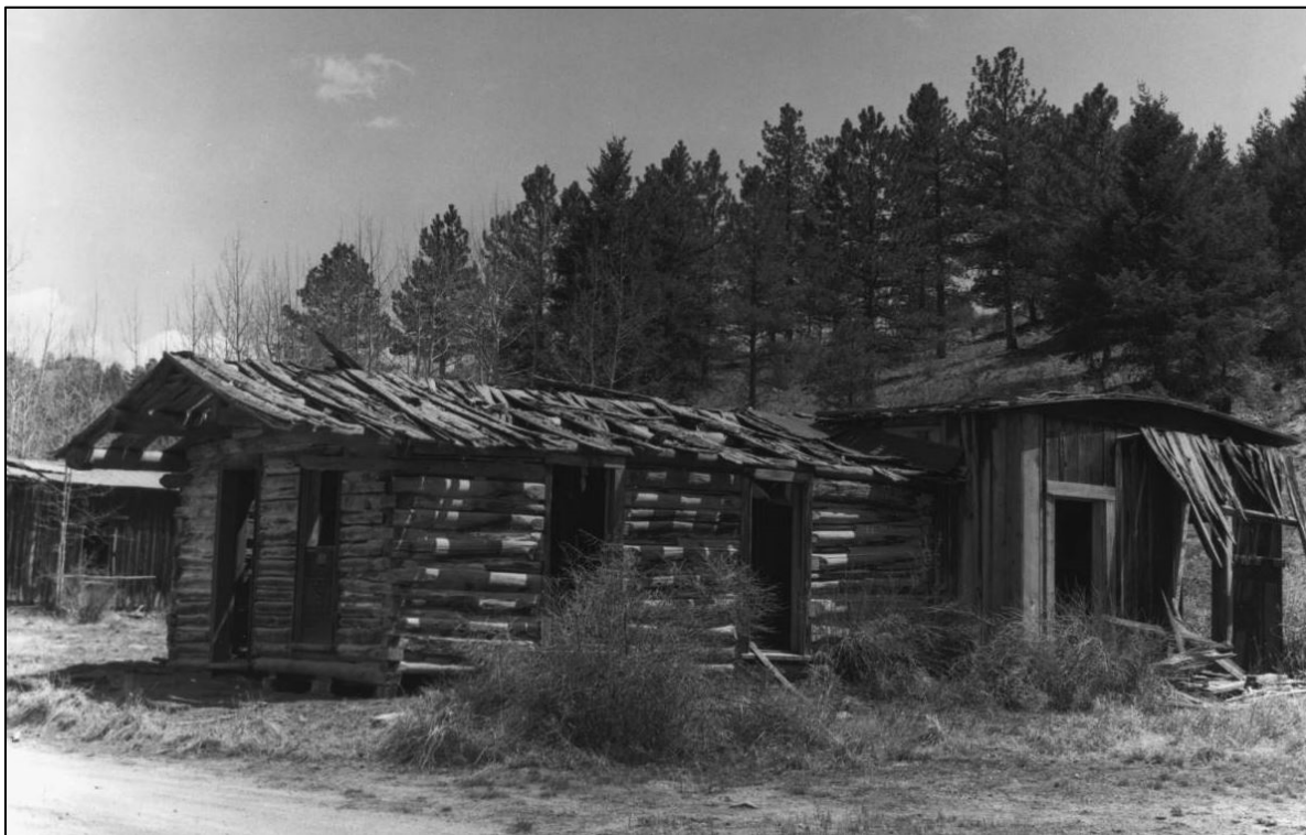
Figure 5. Local historian Dick Dixon took this view of the deteriorated building in 1975 (view southeast). Courtesy of Western History and Genealogy Department, Denver Public Library, Denver, Colorado, photograph number X-13917, May 1975.
