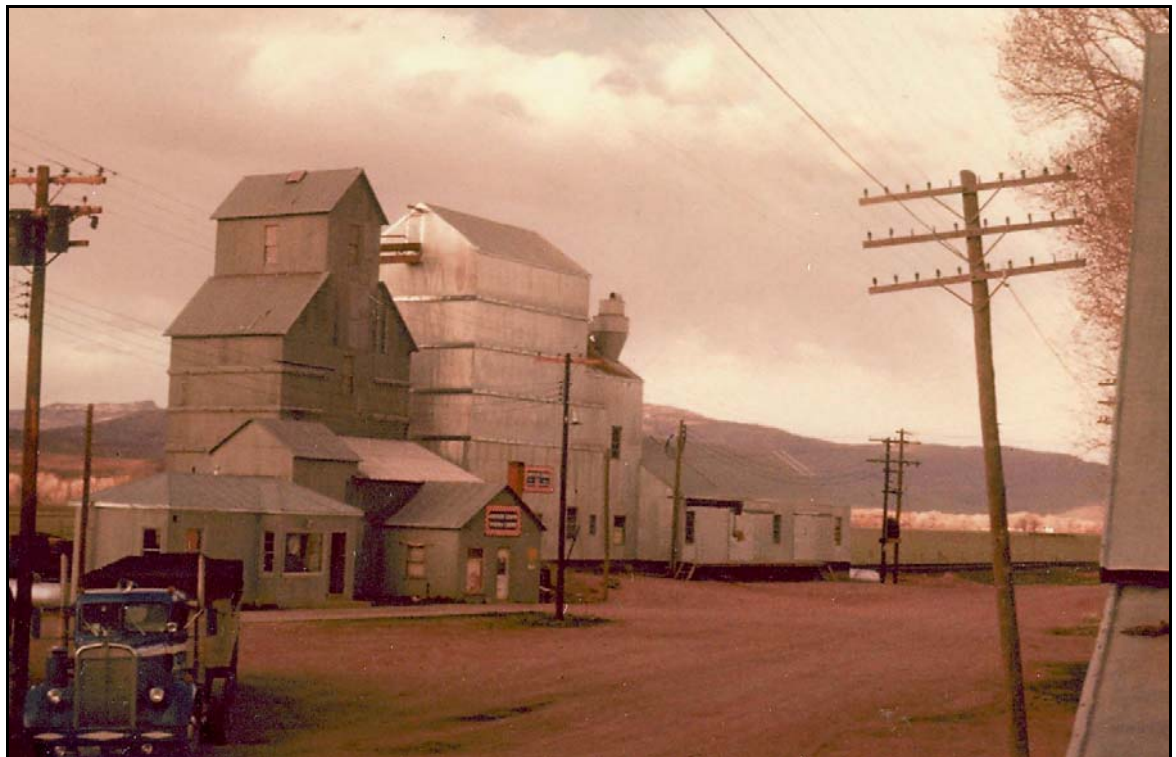
Hayden Grain Elevator shortly after construction of the pellet mill and half of the processing plant, camera facing northeast, circa 1955. (Courtesy: Tammie Delaney personal files, Hayden, CO)
