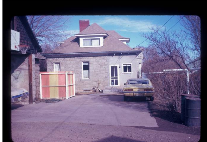
Fig 11 – West-facing (rear) of house after resurfacing of backyard with concrete, 1967.
