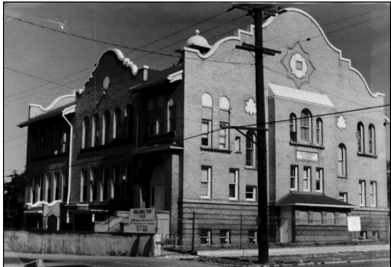
The 1902 Byers-Alameda School exhibits the distinctive curvilinear gable parapets that characterize the Mission style. Unlike the Columbian School, the Byers-Alameda uses the rectangular plan typical of school designs of the early twentieth century. (Source: Office of Archaeology and Historic Preservation, Colorado Historical Society)
