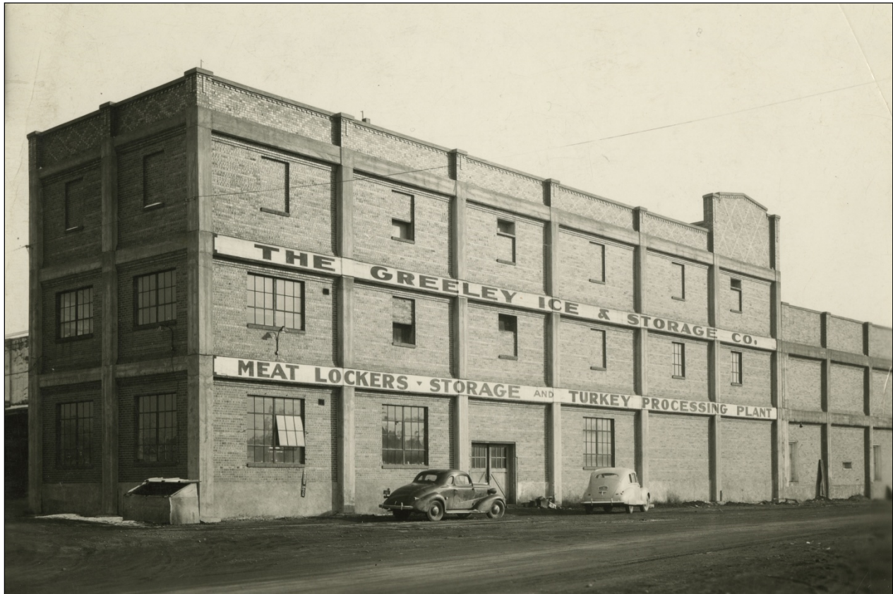
Figure 7. The three-story 1930 portion of the building is to the left with the 1939 two-story portion at the far right in this ca. 1940-50 view to the southeast. Note the factory-style windows with movable awning panels. The "ICE" sign on the elevator tower is not yet present. Courtesy of City of Greeley Museum, Greeley, Colorado, image number 1981.64.0002.
