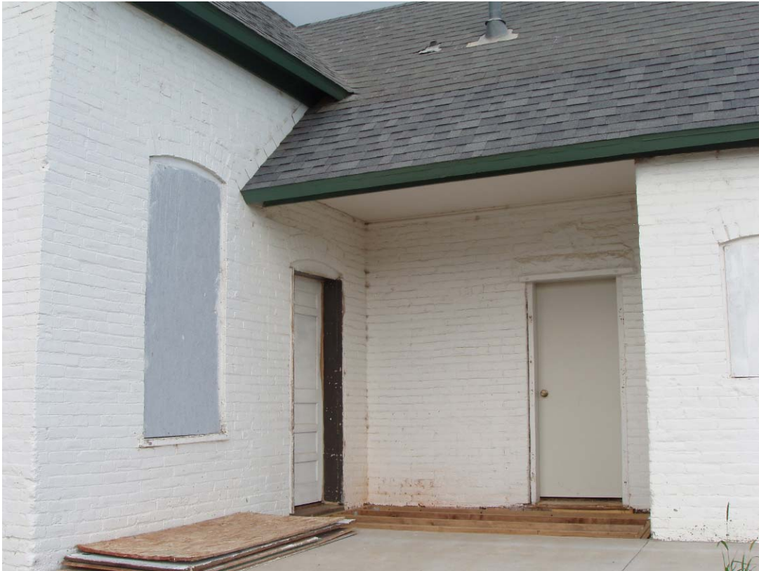
Fig. 14 2011 Southeast Porch, during restoration
