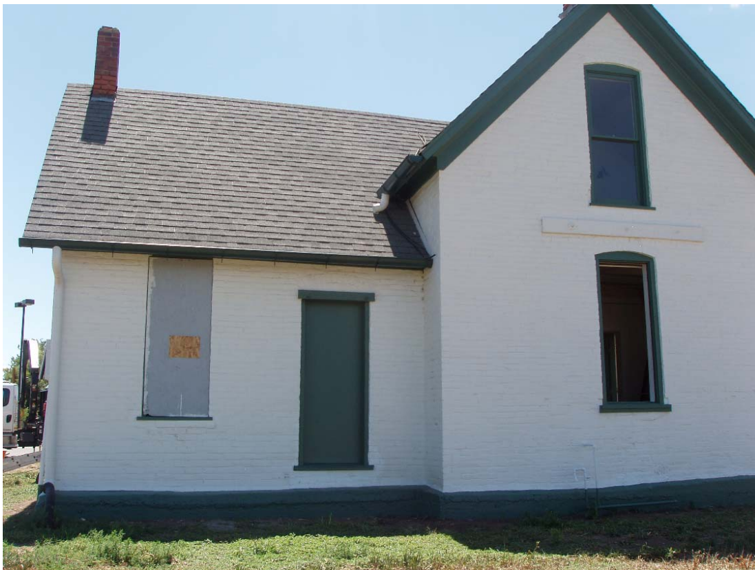
Fig. 15 2011 Northwest-facing side, during restoration
