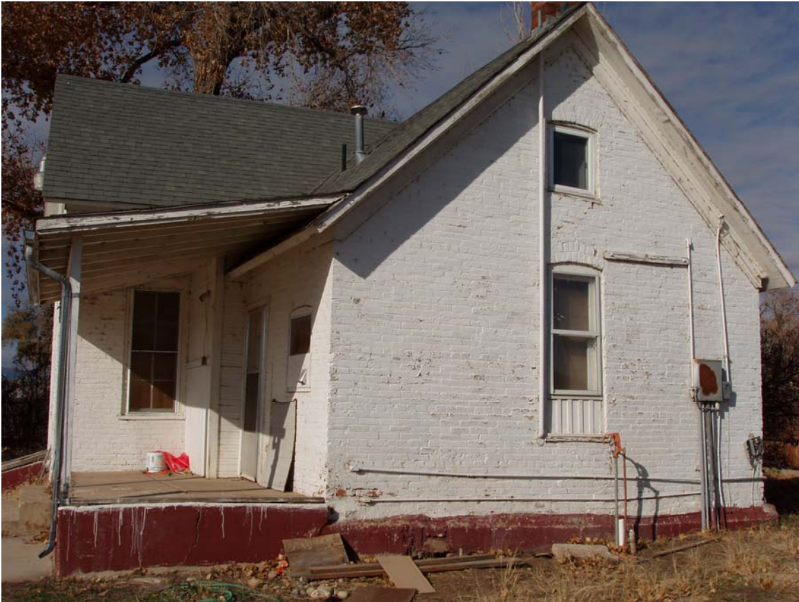
Fig. 8 2009 Northeast Façade, prior to restoration
