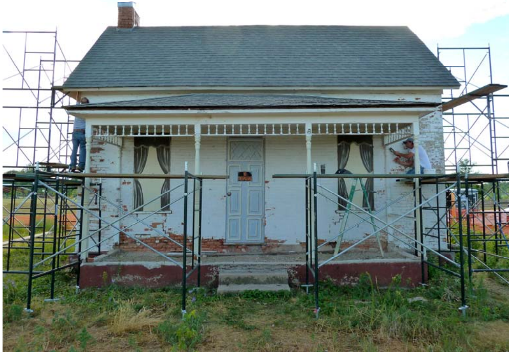
Fig. 12 2010 Southwest Façade, during restoration
