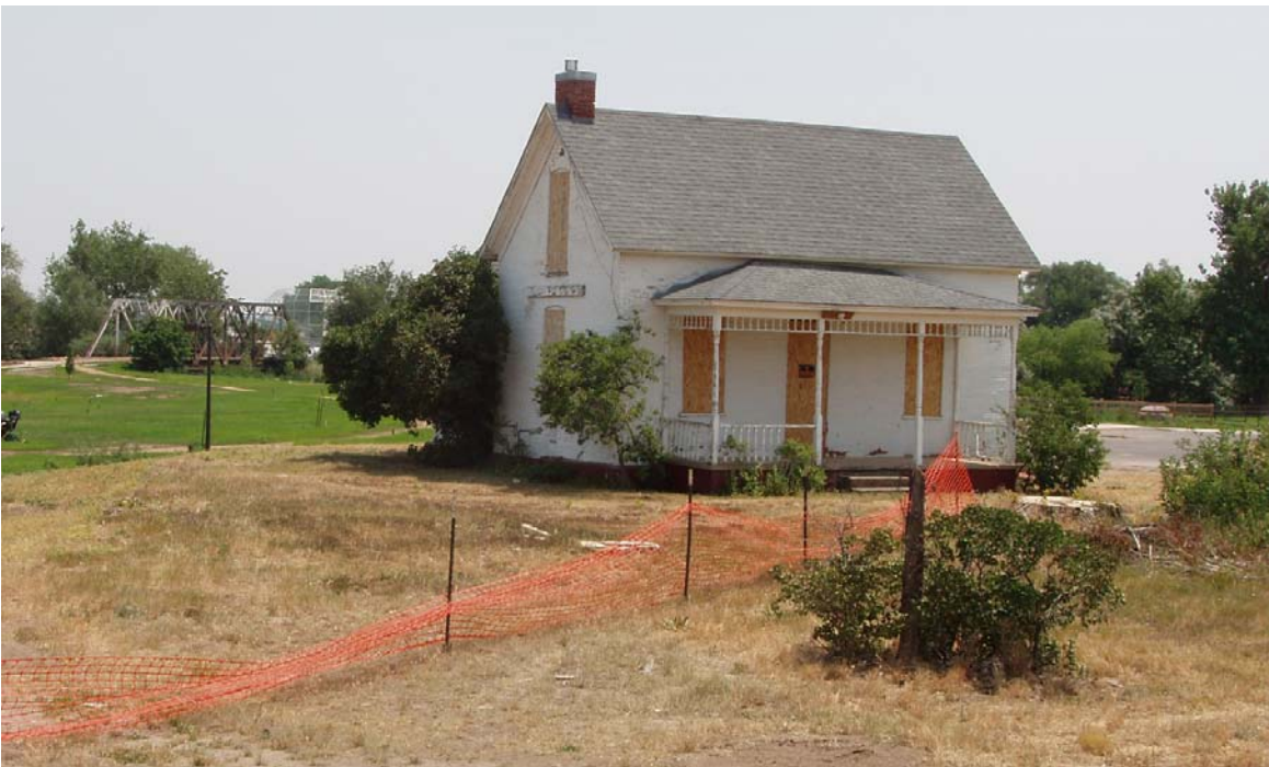
Fig. 9 2009 Southwest (main) Façade, prior to restoration
