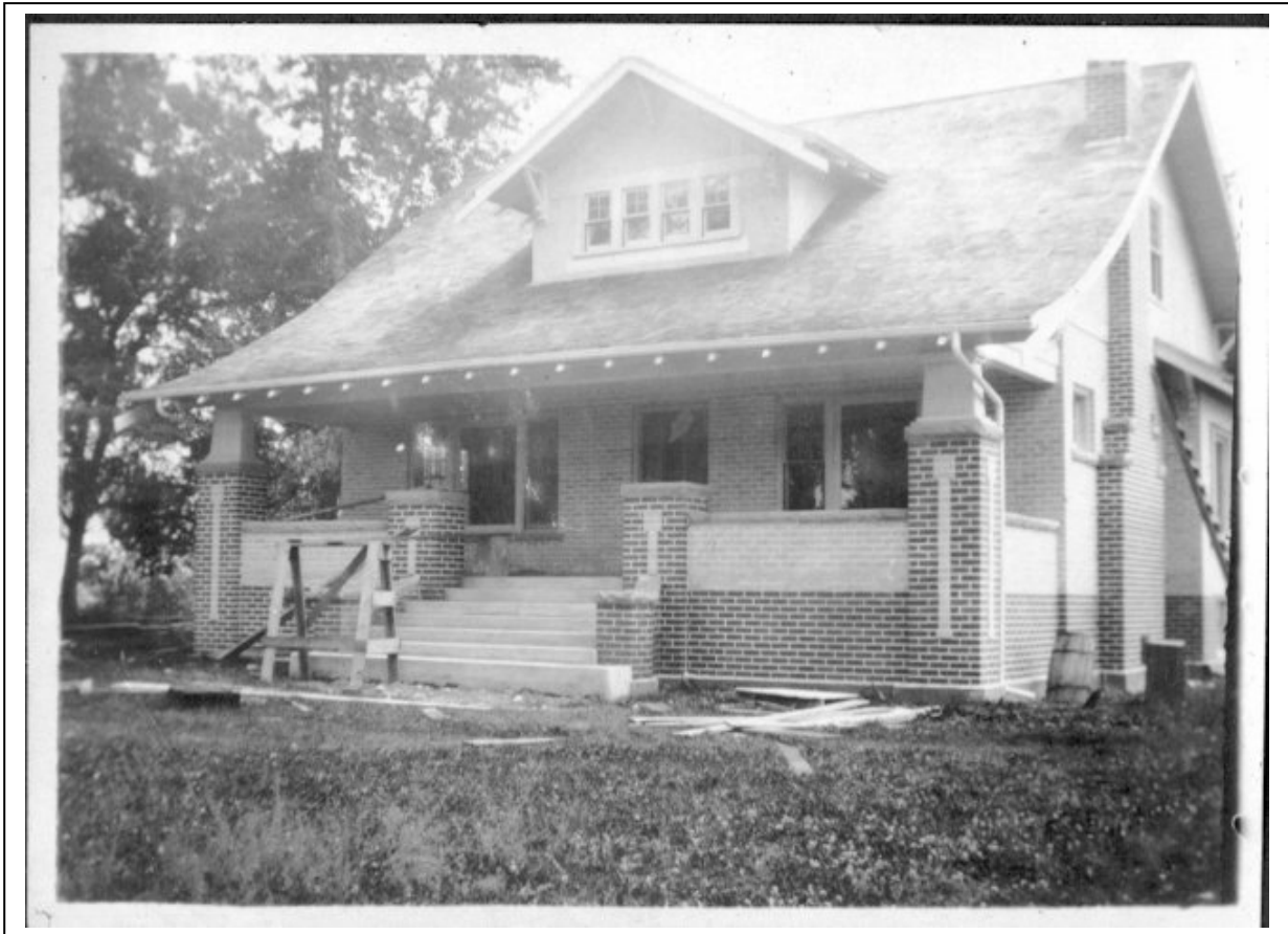
Gustav and Annie Swanson Farmhouse Under Construction - 1918
