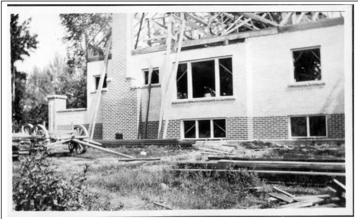
Swanson Farmhouse Under Construction - 1918
