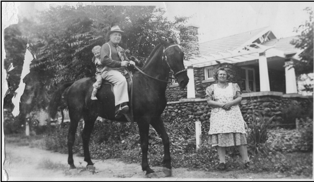
Figure 8: East-facing side of house, camera facing west, with Samuel Albina on horse along with friends, ca. 1950s.
