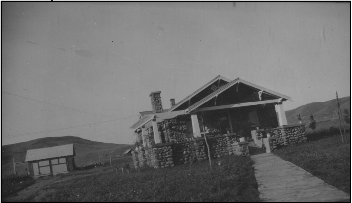
Figure 1: North-facing side of property with house outbuilding, camera facing south, ca. 1929.
