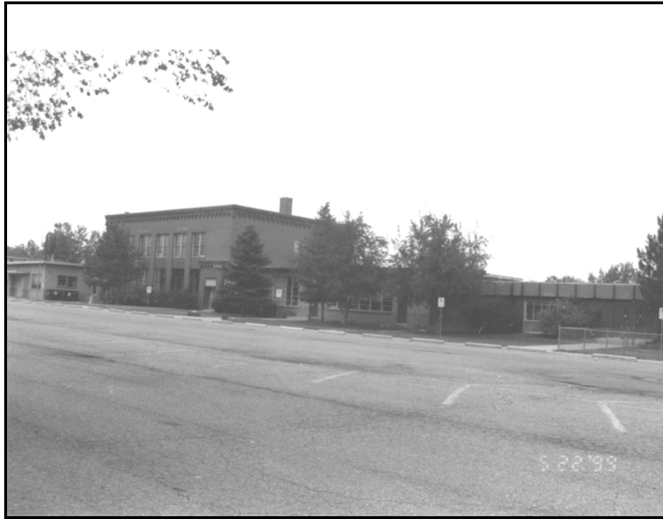
Figure 8: Overview of Fruitdale School and additions. Photo taken by Robert J. Olson, May 22, 1999, in the files of the Office of Archaeology and Historic Preservation, Denver, Colorado
