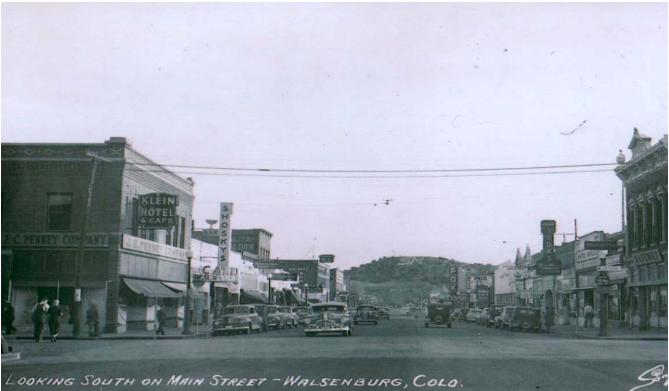
Photo H-1: J.C. Penney, ca. 1940, looking south on Main Street.
