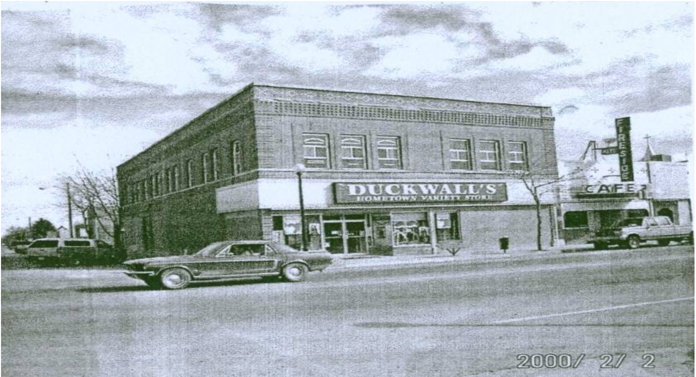
Photo H-5: Duckwall, entire building with offices on second floor, 2000.
