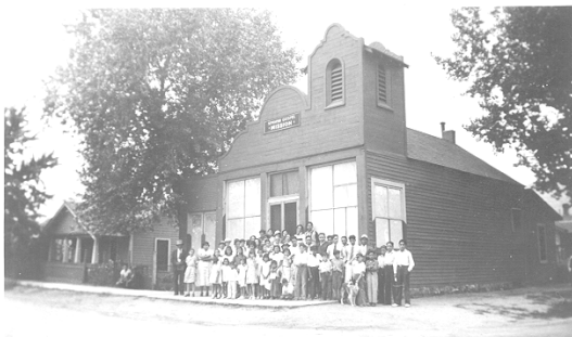
H4. c.1939 photo showing partial completion of renovation project, including the bell tower and curvilinear parapet.
