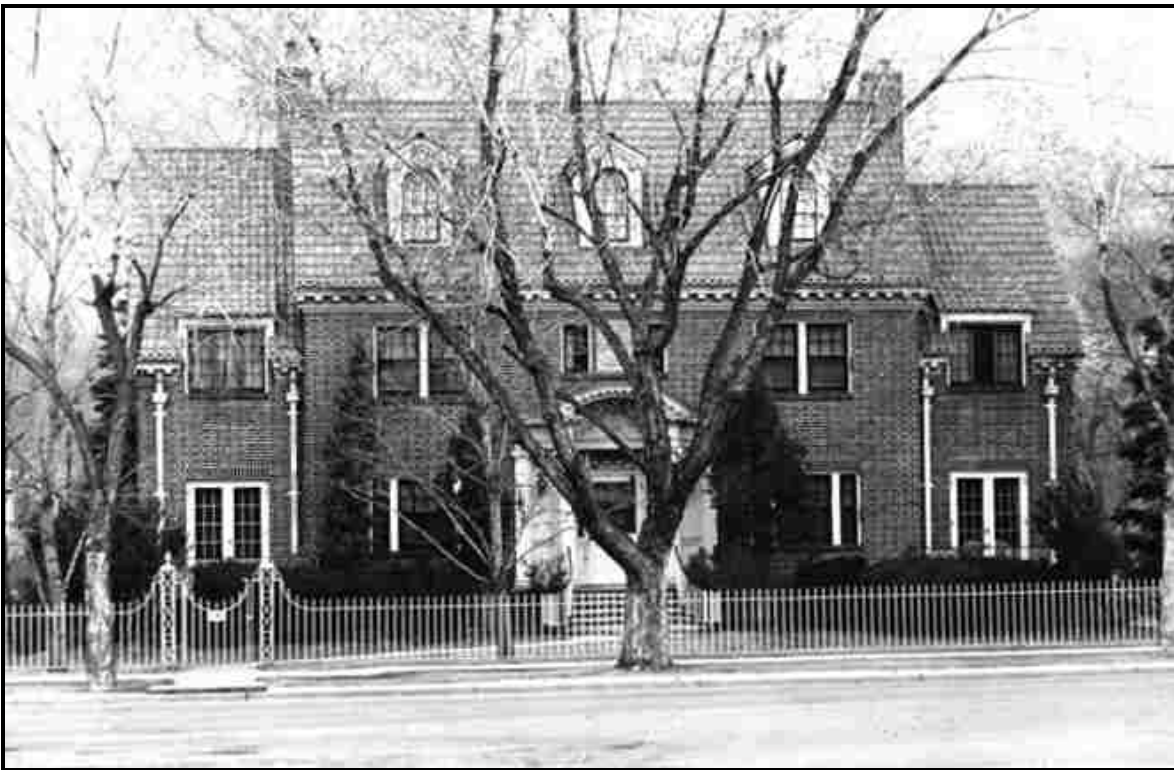
Figure 2. The Ida Rice House was owned by Edgar L. Study, a Kansas oilman, at the time this photograph was taken in 1959. SOURCE: Pikes Peak Regional Library, Special Collections, Myron Wood photograph, call number 002-1345-di-72, March 1959.
