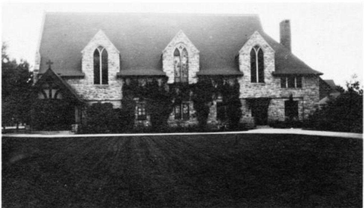
H0002. View of west elevation of 1884-95 portion of the building prior to 1925 addition
