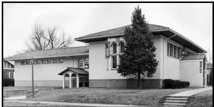
Figure 4. The Park Hill Library received a new entry and a large rear addition in the early 1960s. Photo circa 1963. Source: Western History/Genealogy Department, Denver Public Library
