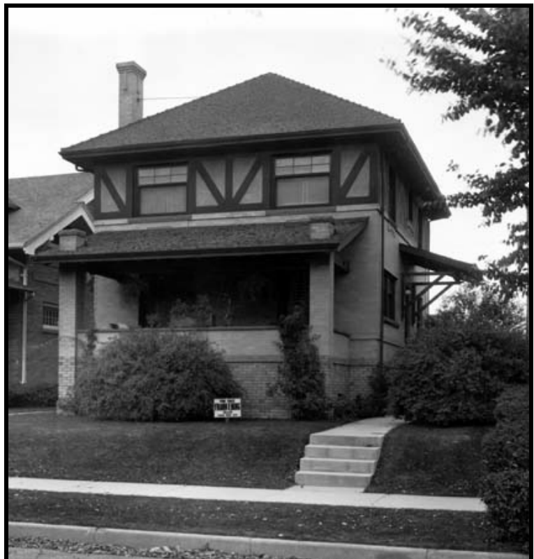
Figure 11. The two-story house at 2308 Birch exhibits the form of the residential Foursquare-type and Craftsman architectural styling. Built in 1909, this photograph dates from about 1925. Source: Western History/Genealogy Department, Denver Public Library
