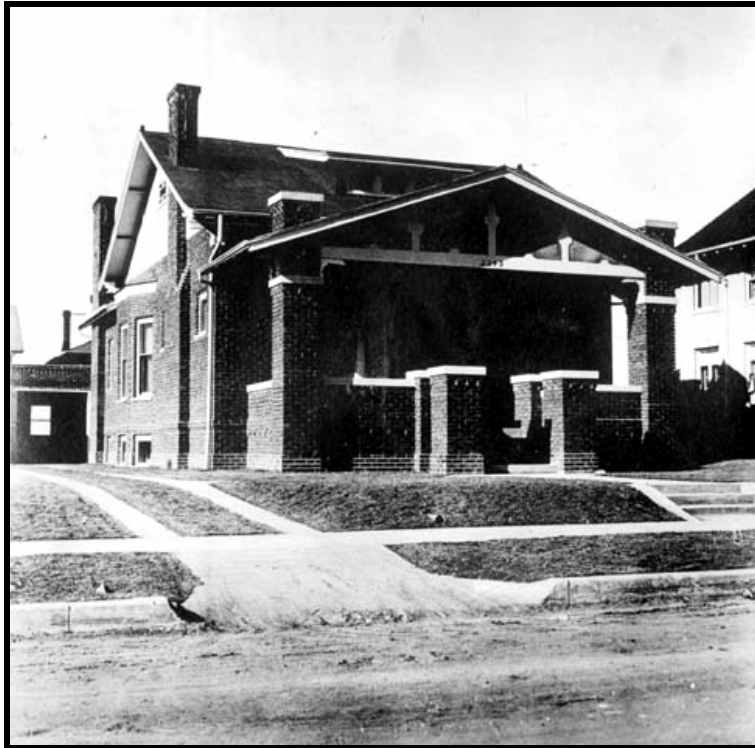
Figure 10. The 1906 Charles Collins House at 2245 Albion typifies the Bungalow-type found throughout Park Hill. Brick porch columns extending through the porch roof is a common feature in Park Hill, and is sometimes referred to as a "Park Hill Porch." Photograph circa 1910. Source: Western History/Genealogy Department, Denver Public Library.
