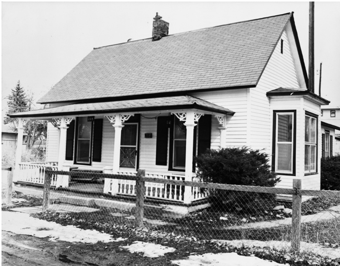
2. ca. 1960s – Looking Northeast at the West Side
