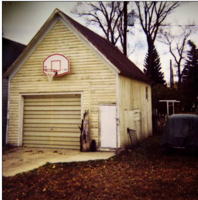
Figure 6. The barn/garage at the southwest corner of the property is shown in this 1997 Assessor photograph (view southwest). Courtesy of Chaffee County Assessor, Salida, Colorado, 23 October 1997 photograph.
