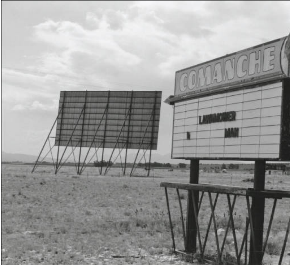
Figure 5. This ca. 1990s southeast view from County Road 306 shows the attraction board/marquee sign, screen tower, and projection booth/snack bar/restroom building (right edge beneath the sign). Lawnmower Man , a science fiction film, was released in 1992. Courtesy of Thomas J. Noel, image AUR-950, Denver Public Library, Denver, Colorado.
