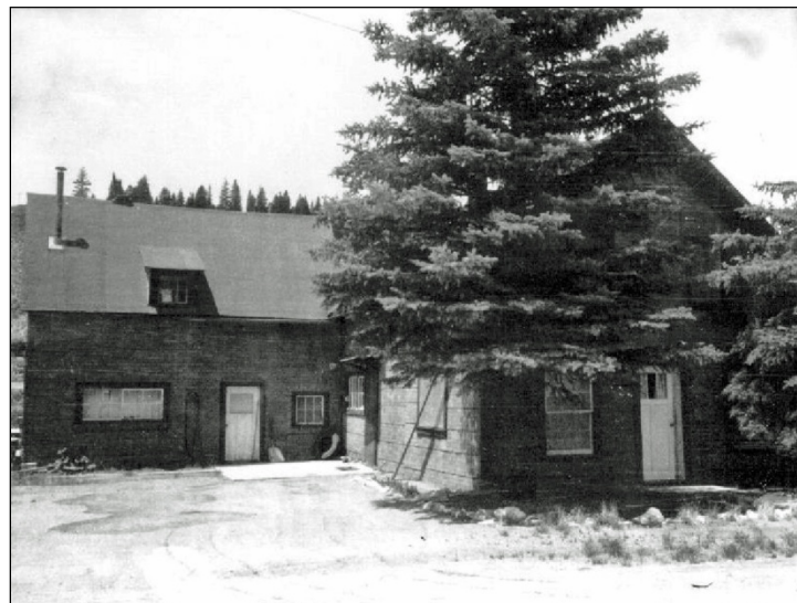
Figure 9. The hotel building was clad with rolled asphalt siding resembling brick in 1974 (view west-northwest). Courtesy of History Colorado, survey form photograph, 5CF.155, 1974.
