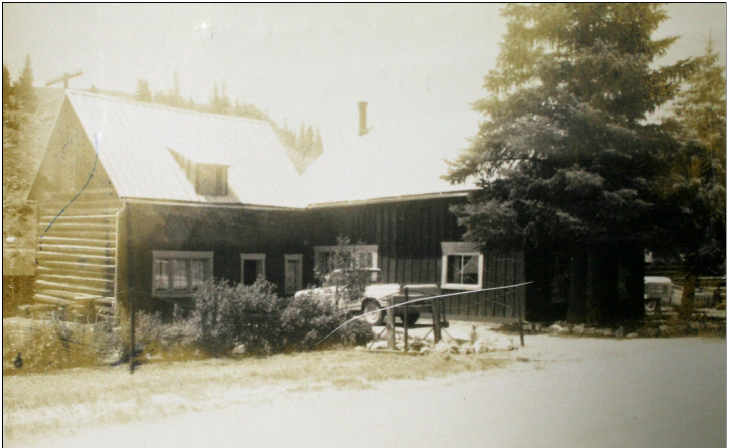
Figure 11. This undated Assessor photograph (view northwest) shows the hotel building in the late 1970s or 1980s. Courtesy Chaffee County Assessor, appraisal card, Salida, Colorado.
