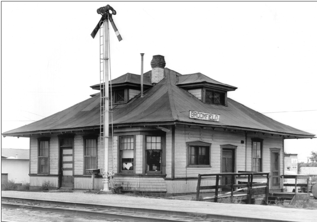
Figure 15. The Broomfield Depot in 1967 had rolled roofing. The platform constructed of railroad ties (to the right) was still present. Courtesy of Broomfield Depot Museum, Collection 1997.4.2.
