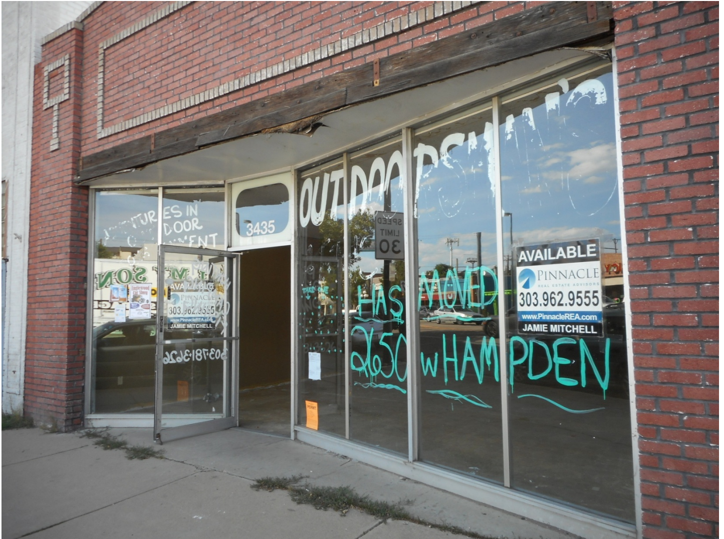
The façade of 3435 South Broadway showing the 1950s-60s aluminum and plate glass storefront prior to restoration in 2015-16. Photo: Diane Tomasso, 2015.
