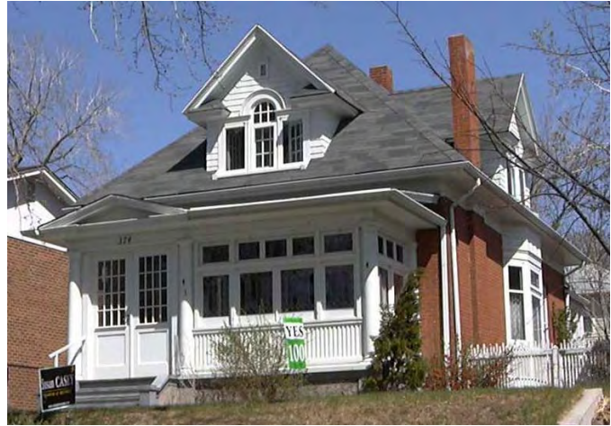
This High Style Classic Cottage in Denver exhibits facade and side dormers, Palladian-style dormer windows, multiple bay windows and a pediment over the entry stairs.
