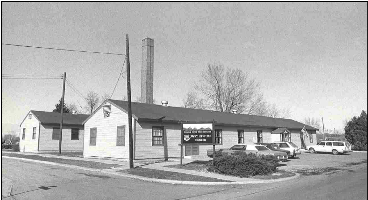
Figure 10. Between 1983 and 1994, the Lowry Heritage Center occupied Building 880, shown here in a 1980s view. SOURCE: Aurora History Museum, photographic collection.
