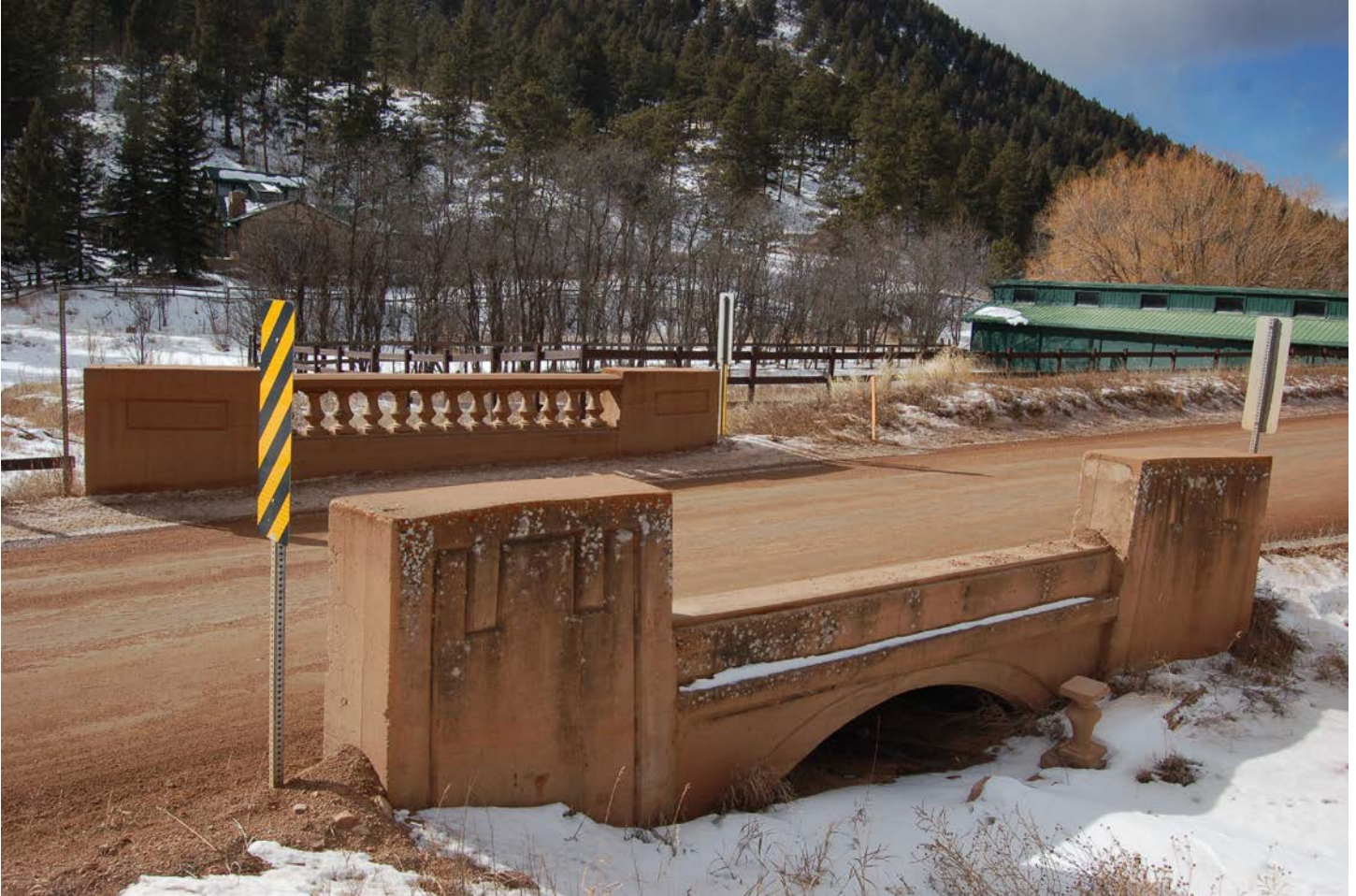
Photo 5 of 10: Easternly exterior, looking northwest.
