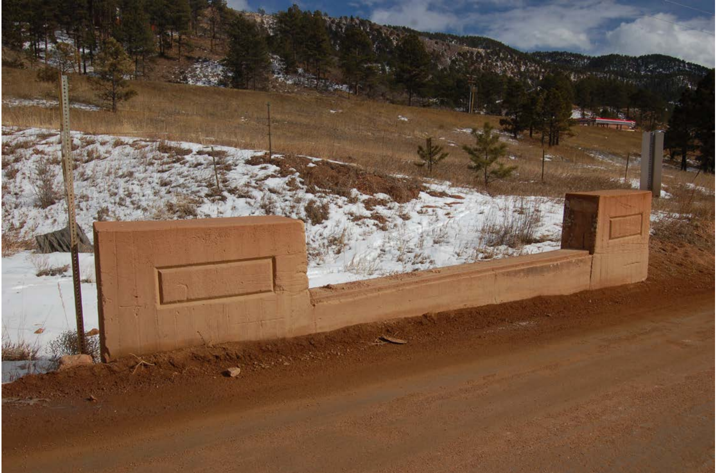
Photo 8 of 10: Easternly interior looking southeast.
