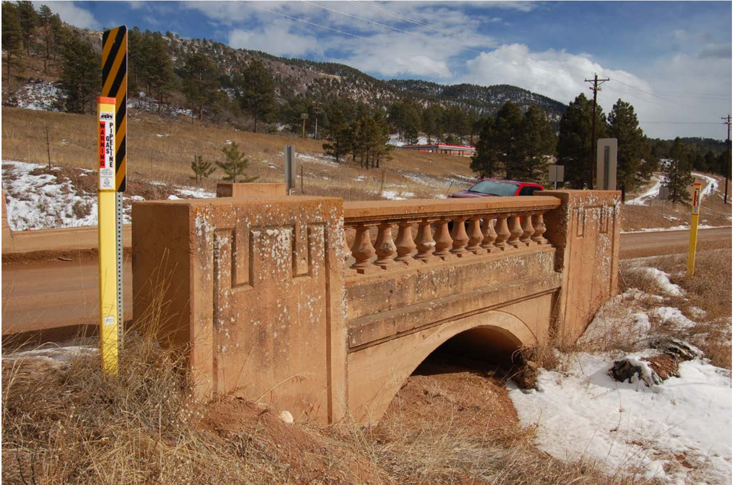
Photo 2 of 10: The westerly exterior, looking southeast.
