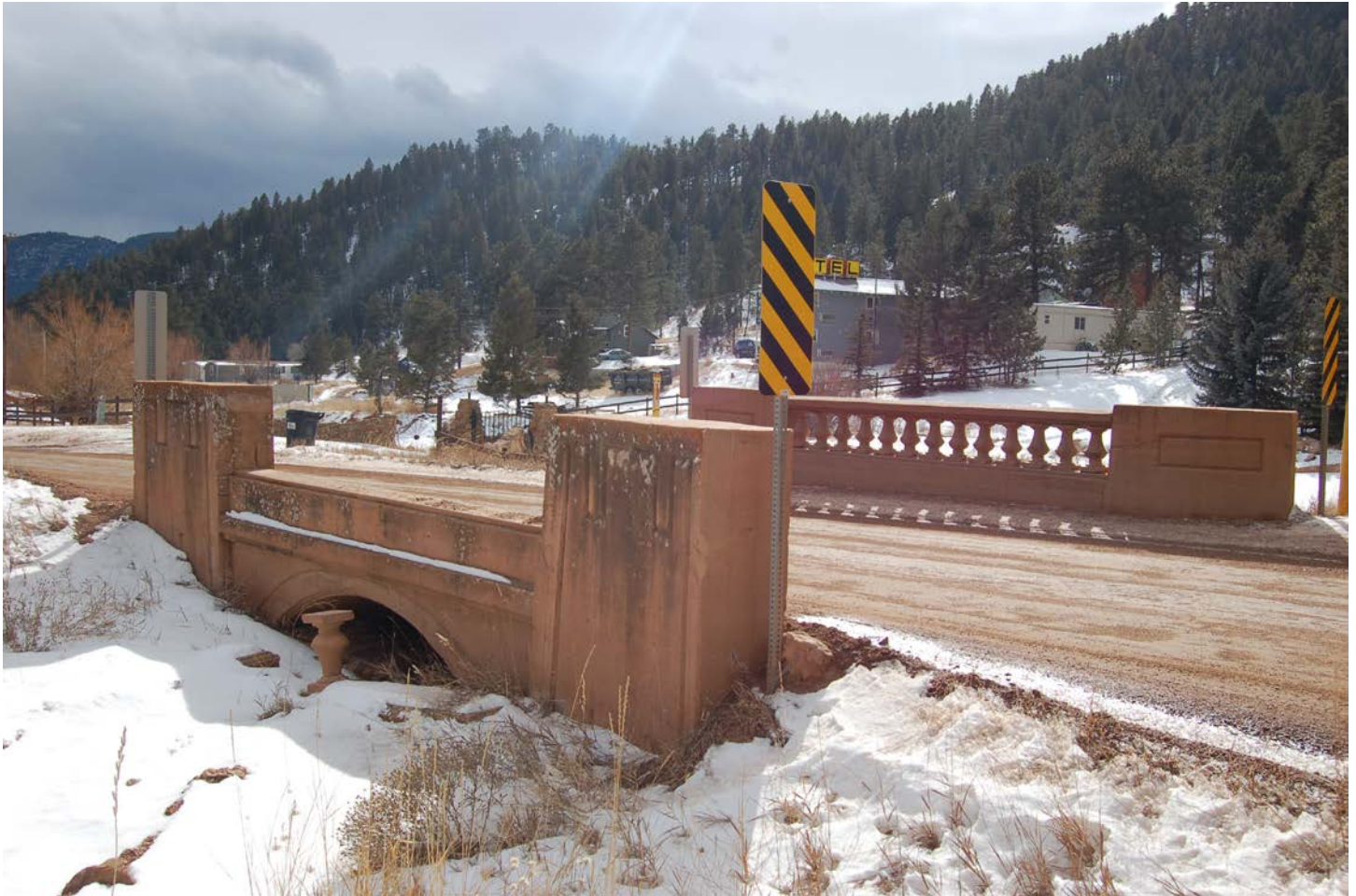
Photo 6 of 10: Easternly exterior, looking southwest.
