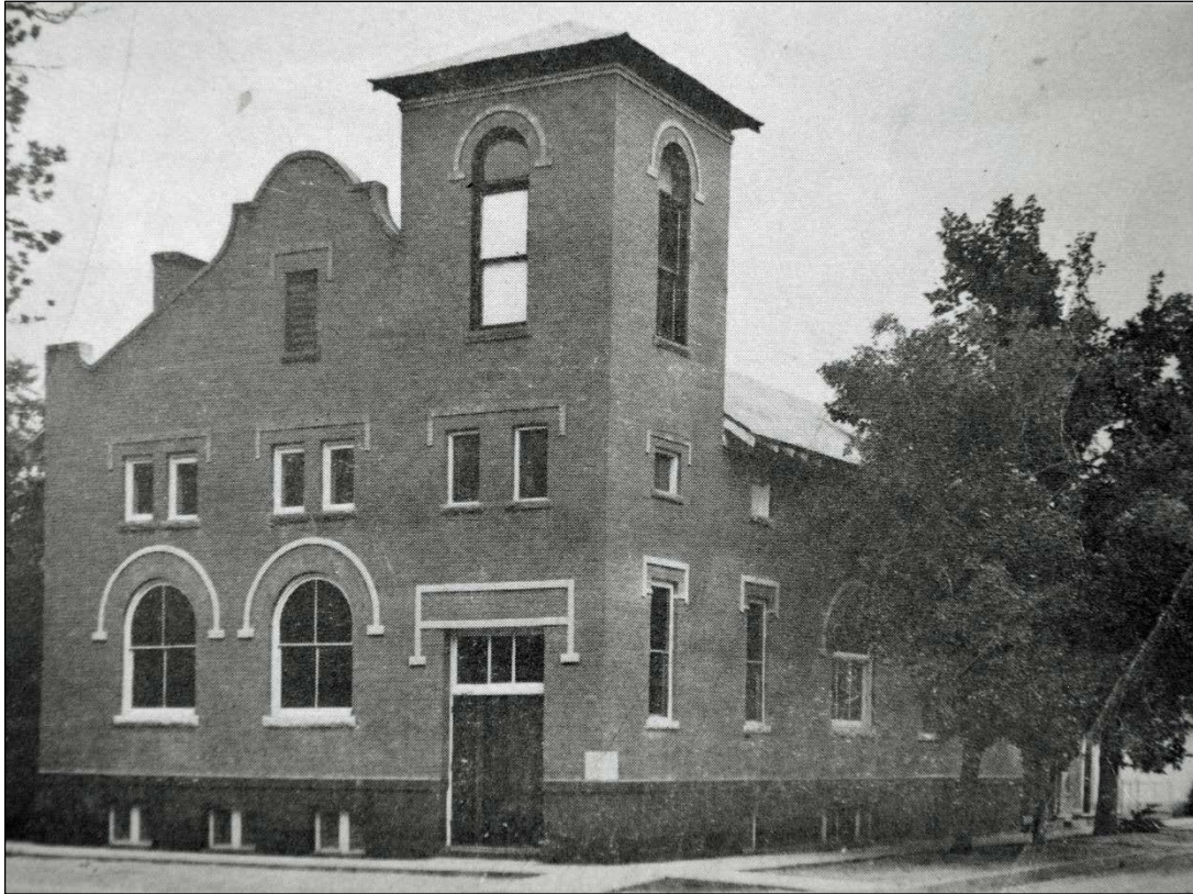
Figure 4. The front and south wall of the church are shown in this 1957 view northeast. The choir loft windows are not bricked in, the third story of the tower holds one-over-one windows, and the basement windows have not been covered. SOURCE: Colorado AME Conference, Souvenir Program (1957).
