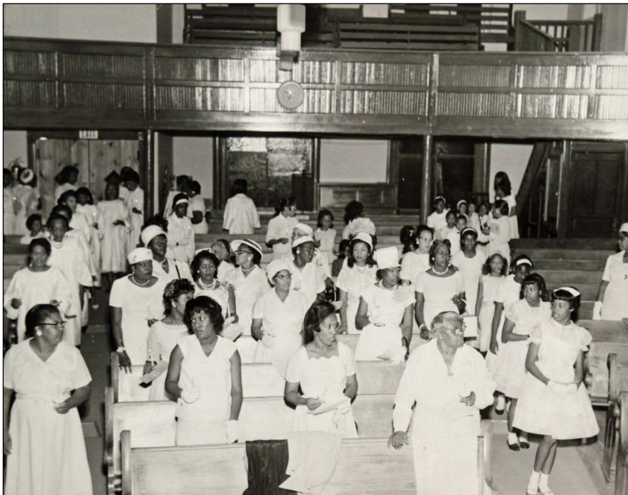
Figure 7. This interior view west of the nave (pre-1959) shows the choir loft still in place in the background. According to a church history, Rev. A.H. Hamilton removed the choir loft during his 1955-59 tenure. SOURCE: First AME Church, photograph collection, Pueblo, Colorado.
