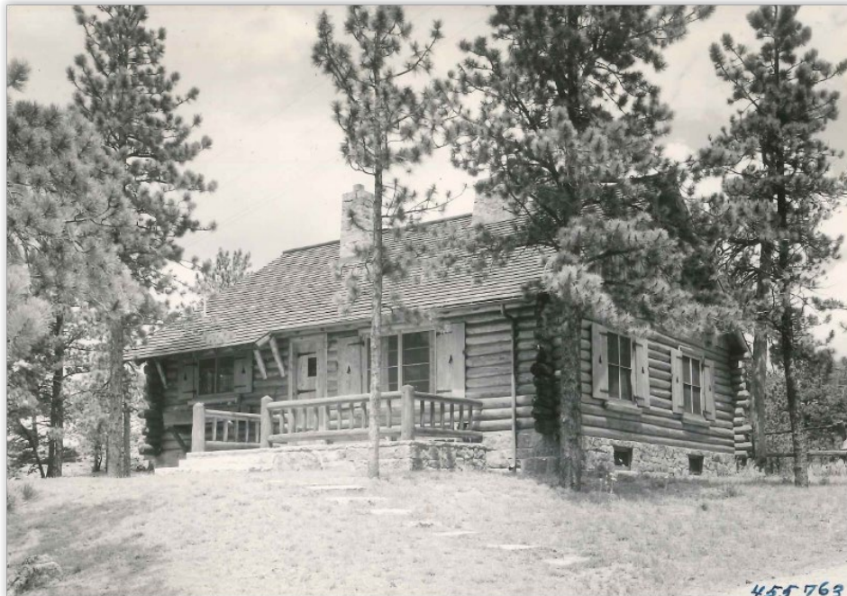
Figure 4: A July 1949 photograph of the Assistant Ranger Dwelling, showing the original front door, kitchen chimney and log front porch railing, all three removed prior to 1967. Source: Roosevelt National Forest Scrapbook, Arapaho and Roosevelt National Forests and Pawnee National Grassland Forest Supervisor's Office, Fort Collins, CO.
