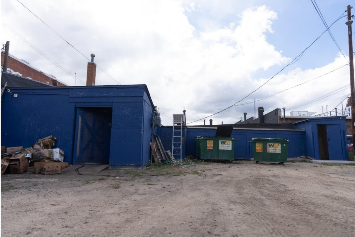
19. Golden Burro, rear parking area facing W, photo by Ned Warner, 9/28/2022 South receiving doors (at left), north receiving doors (at right), outside entry to storage area (center between dumpsters)
