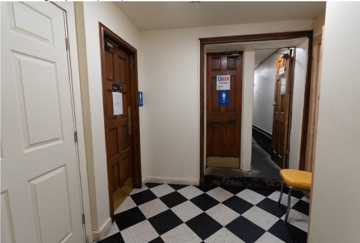
14. Golden Burro, old bathroom entrances facing E, photo by Ned Warner, 9/28/2022 New flooring, mop closet (at left)
