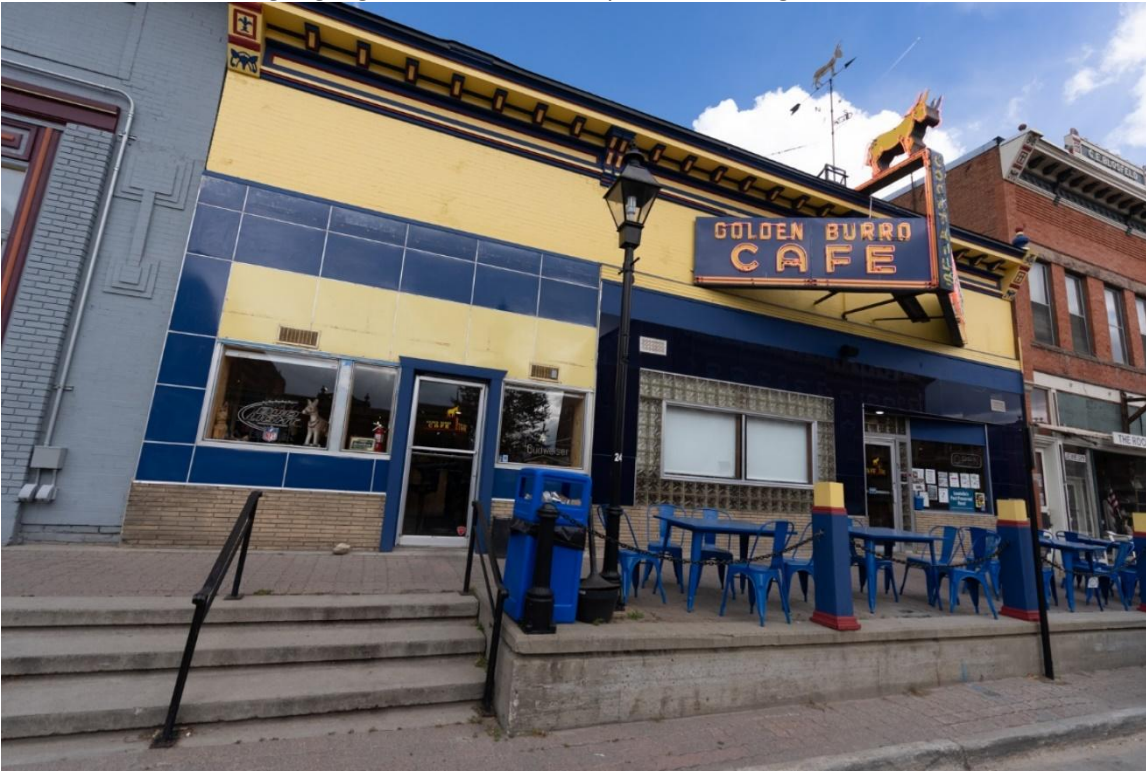
3. Golden Burro Façade, facing ESE, Photo by Ned Warner, 9/28/2022 [Before bollard, awning, signage installation and repair of neon sign]
