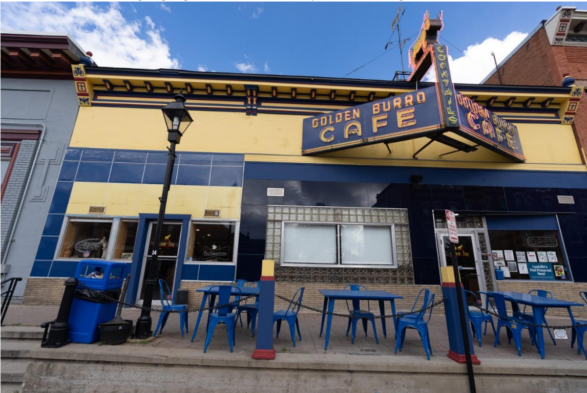
4. Golden Burro Façade, facing E, Photo by Ned Warner, 9/28/2022 [Before bollard, awning, signage installation and repair of neon sign]
