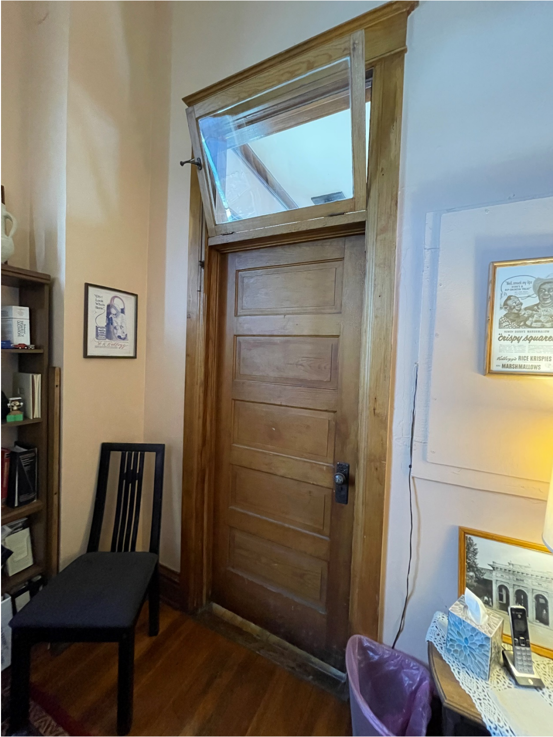
Name of Property: 188 S. Main Street City or Vicinity: Elizabeth, CO County: Elbert County State: Colorado Photographer: Zach Higgins Date Photographed: 18 November 2022
