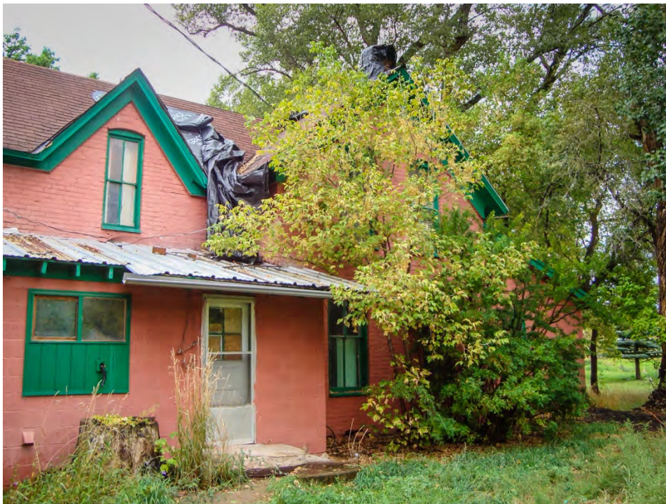
Photo 7 • Northeast Facade, looking southwest. June 2017
