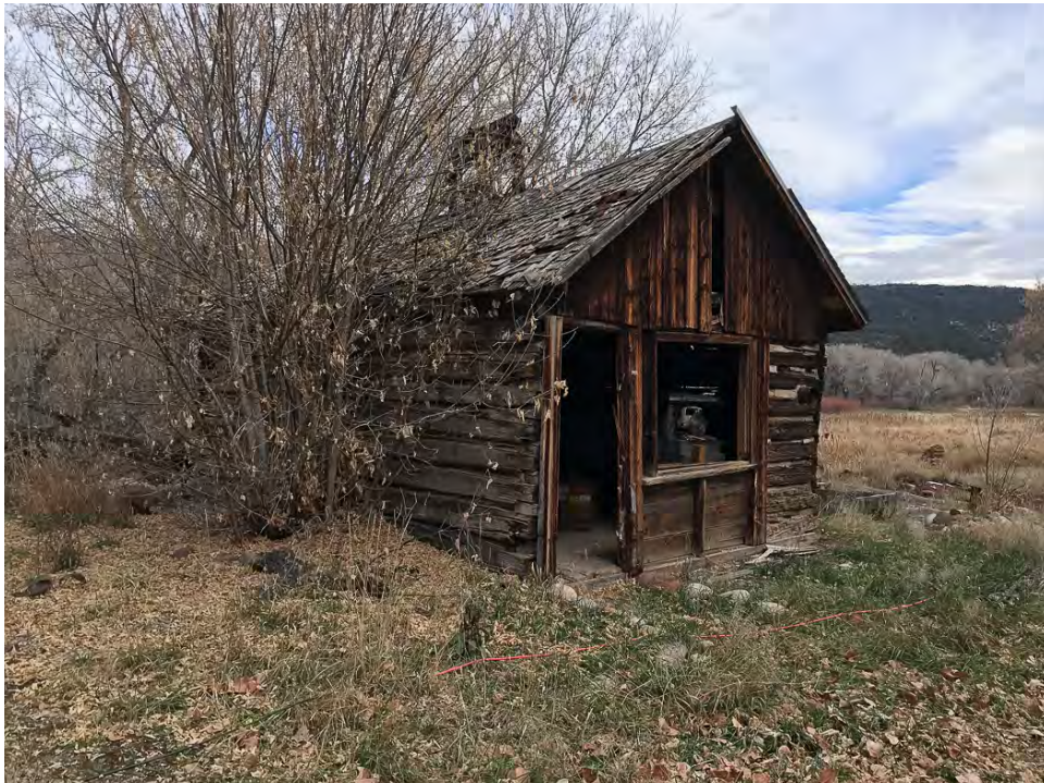
Photo 32 • Log building #2, looking northeast. November 2021
