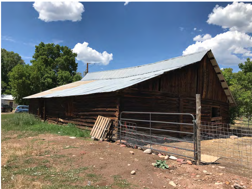
Photo 14 • Log Barn, looking northwest. July 2022
