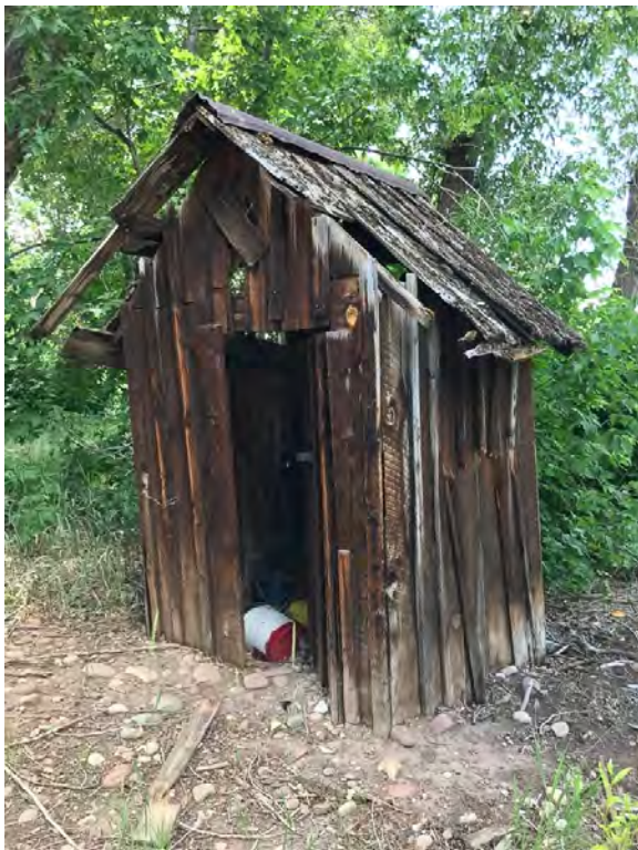
Photo 26 • Privy, southeast facade. Looking northwest, July 2022
