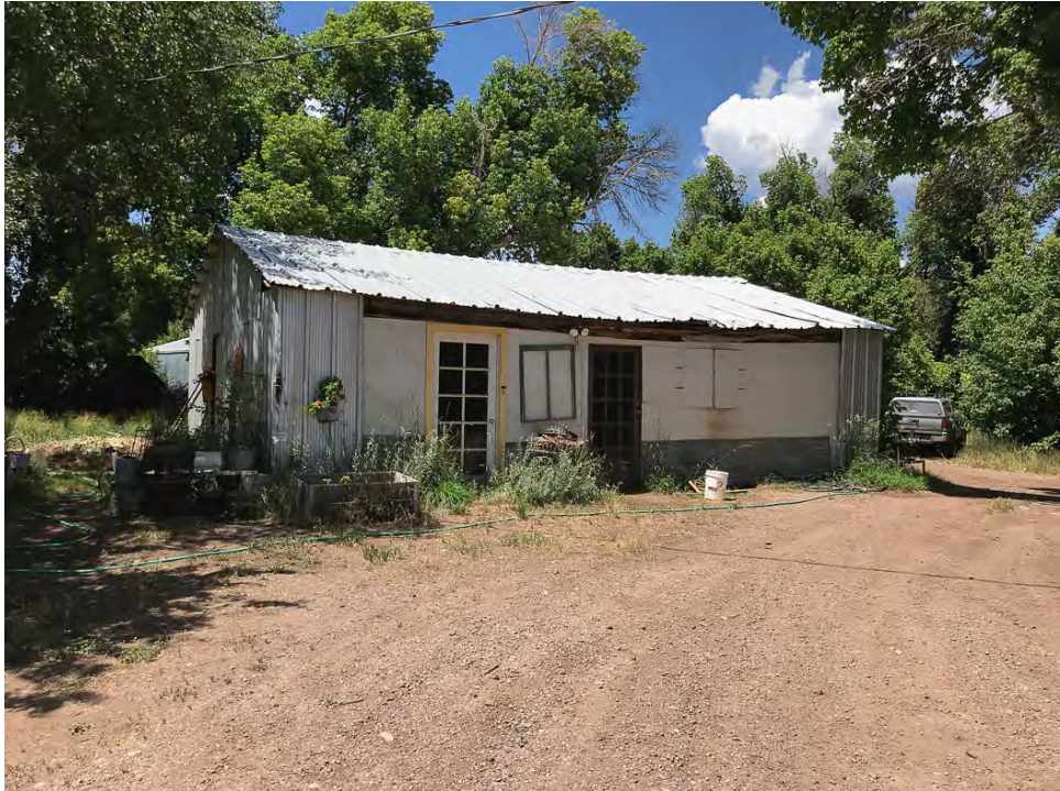
Photo 22 • Low barn aka garage. Southeast facade, looking northwest. July 2022
