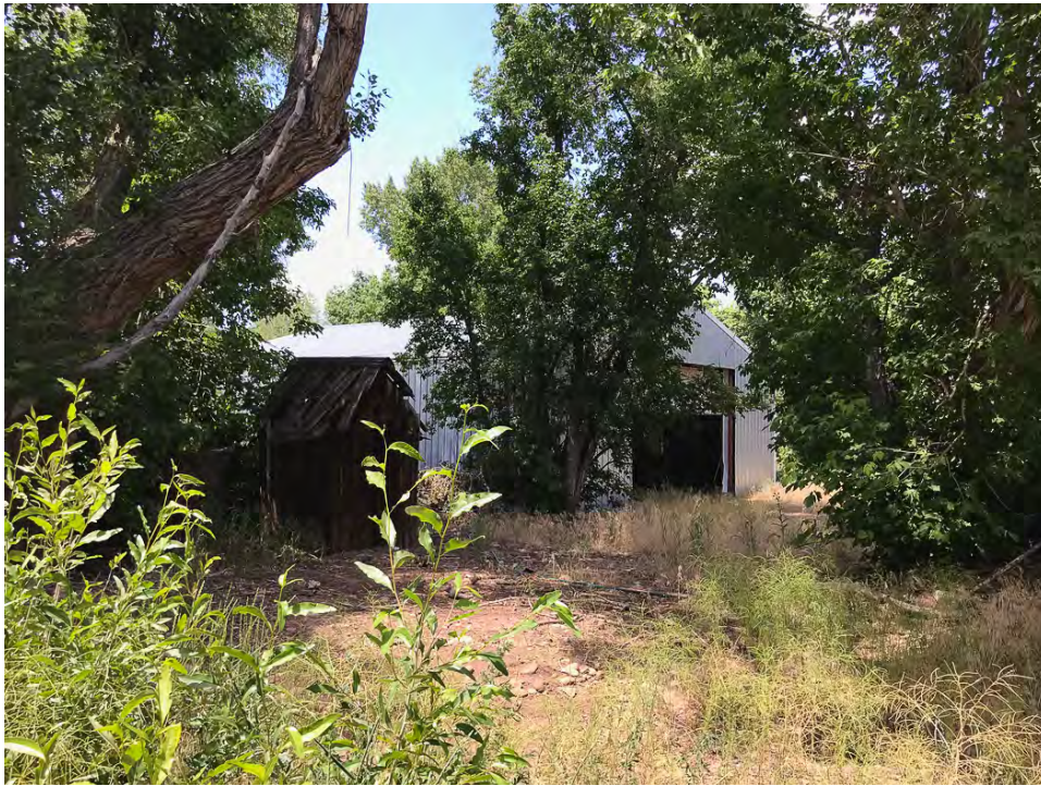
Photo 27 • Metal Barn, southeast facade. Privy in the foreground. Looking northwest, July 2022
