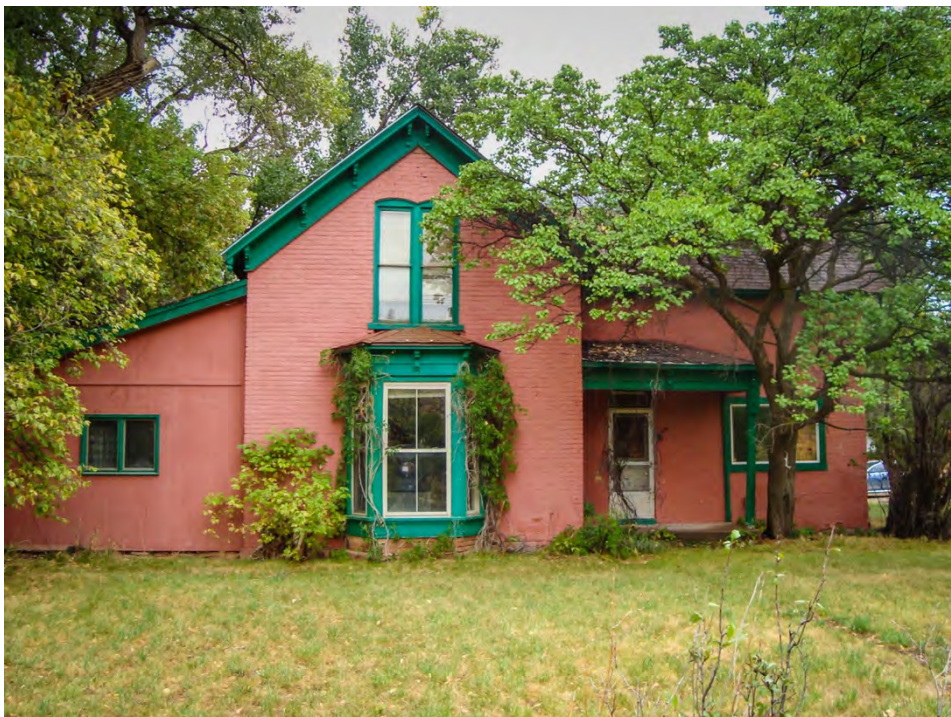
Photo 2 • Southwest Facade, looking northeast. June 2017
