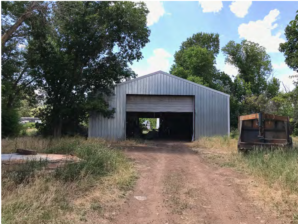
Photo 28 • Metal Barn, southeast facade, looking northwest. July 2022
