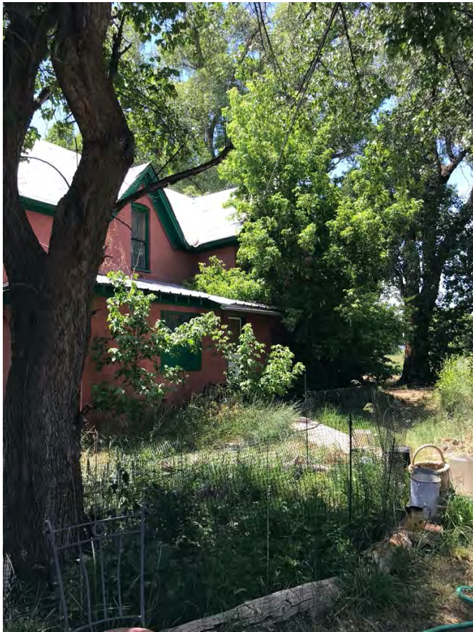
Photo 5 • Northeast Facade, partial, looking southwest. July 2022
