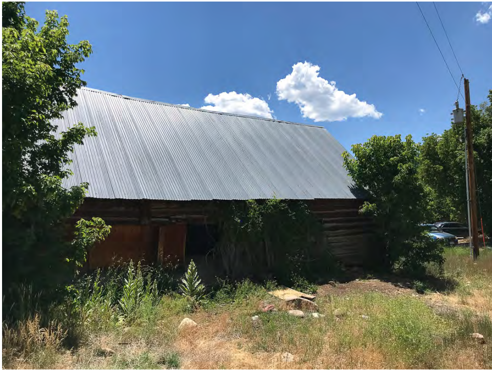
Photo 15 • Log Barn, looking southwest. July 2022
