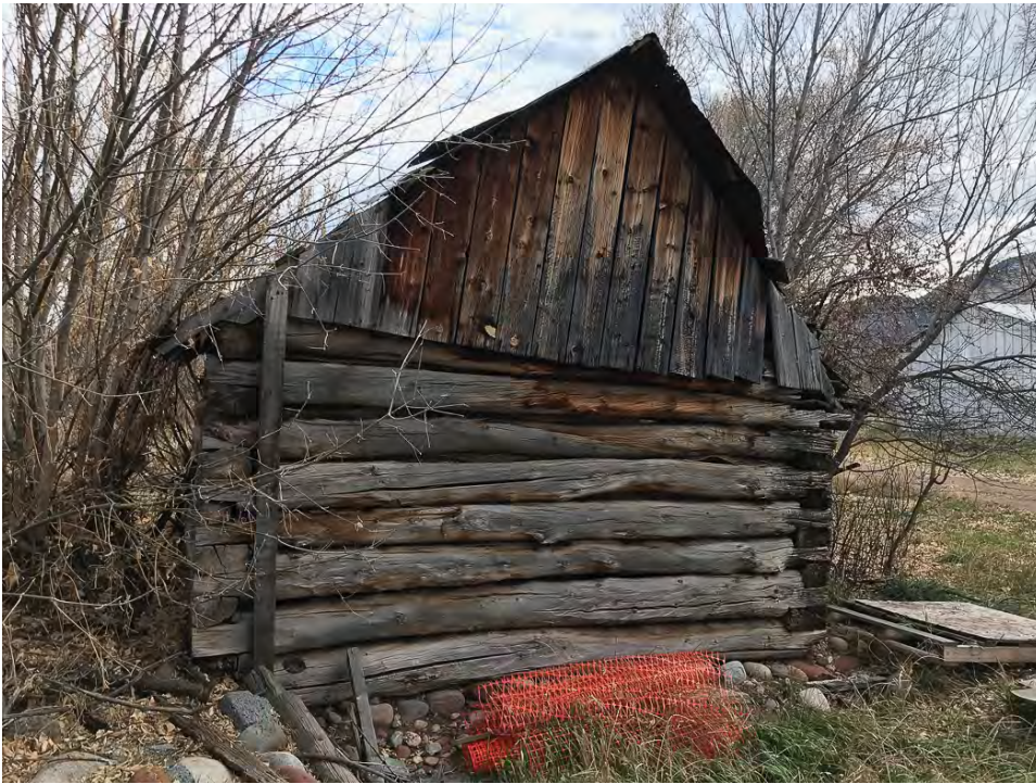
Photo 37 • Log building #1, west elevation. Looking east, November 2021
