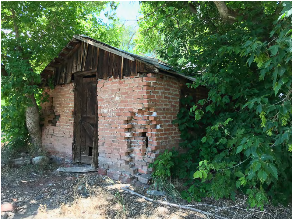
Photo 18 • Brick shed, aka chicken coop. Looking northwest, July 2022
