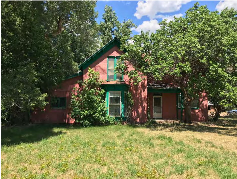
Photo 1 • Southwest (main) Facade, looking northeast. July 2022
