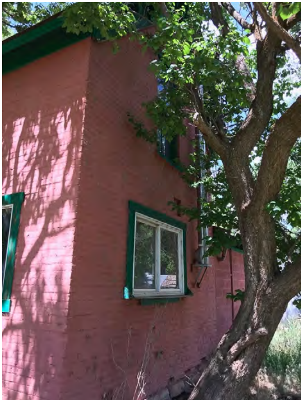
Photo 4 • Southeast facade, looking northwest. July 2022
