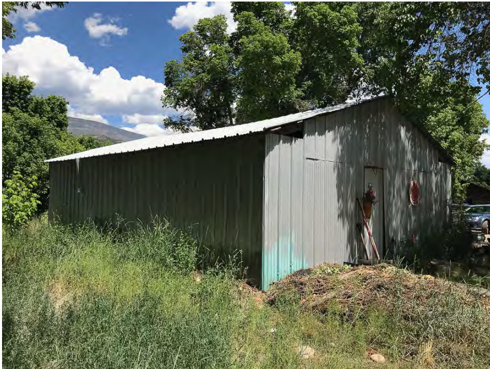
Photo 24 • Low barn, northwest facade. Looking northeast, July 2022
