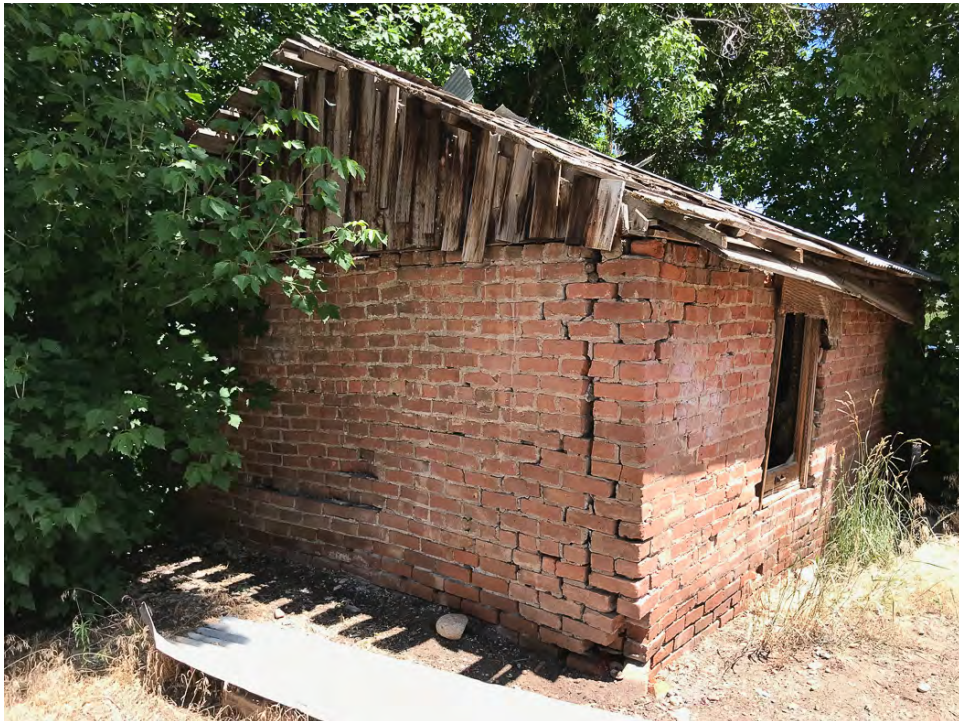
Photo 20 • Brick shed northwest facade, looking northeast. July 2022
