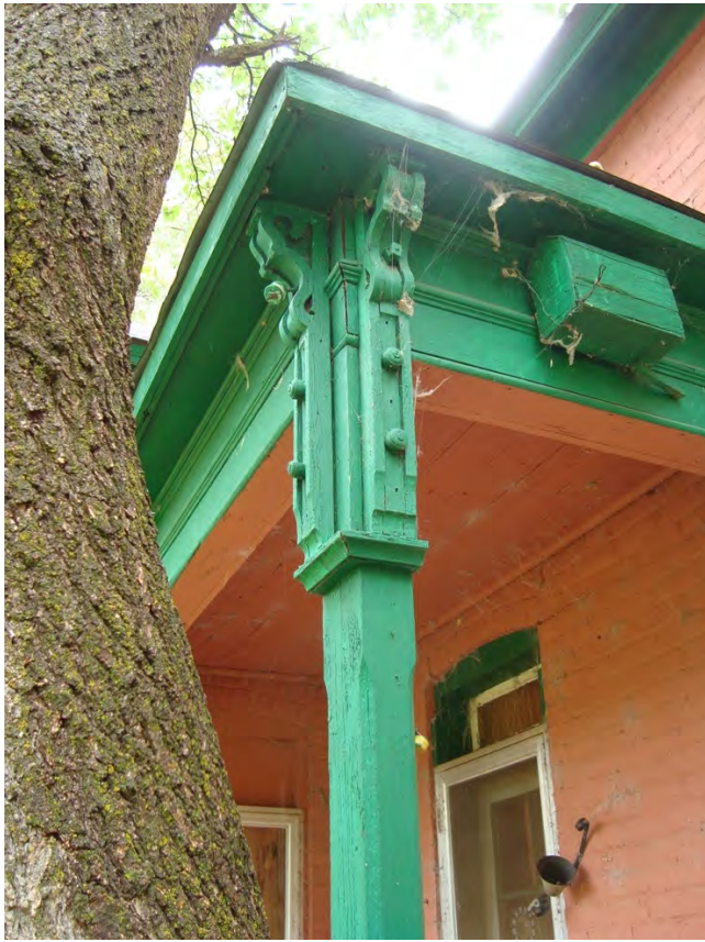
Photo 11 • Detail at southwest porch post & bracket. June 2017
