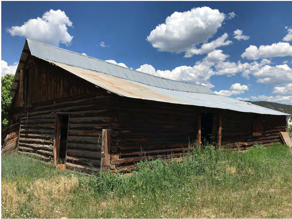
Photo 13 • Log Barn, looking northeast. July 2022
