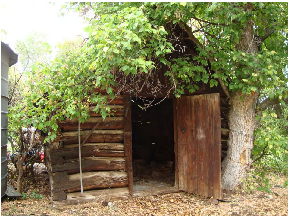
Photo 34 • Log building #1 forge remnants can be seen inside. Looking west, September 2015
