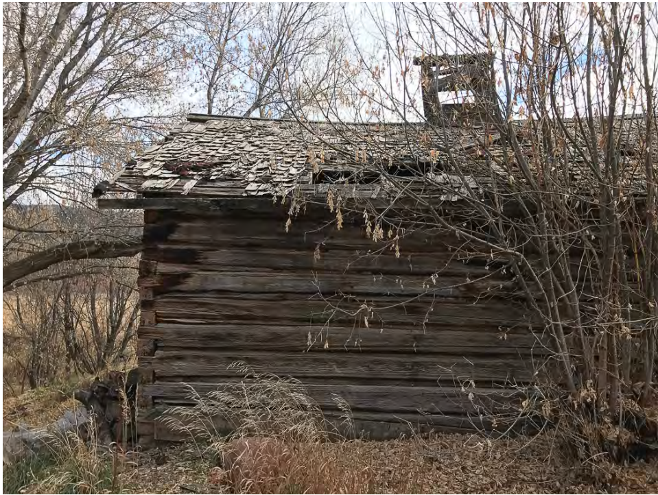
Photo 31 • Log building #2, west facade. Looking east, November 2021
