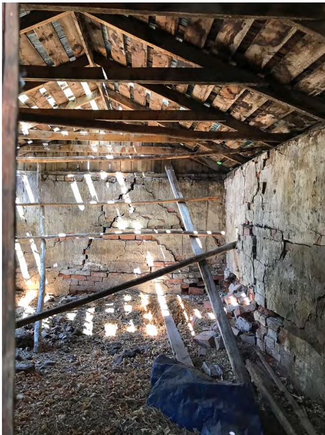
Photo 21 • Interior of brick shed, looking northwest. July 2022
