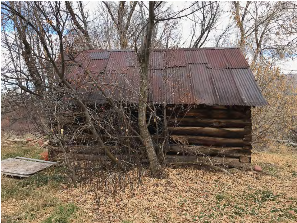
Photo 36 • Log building #1, south elevation. Looking north, November 2021
