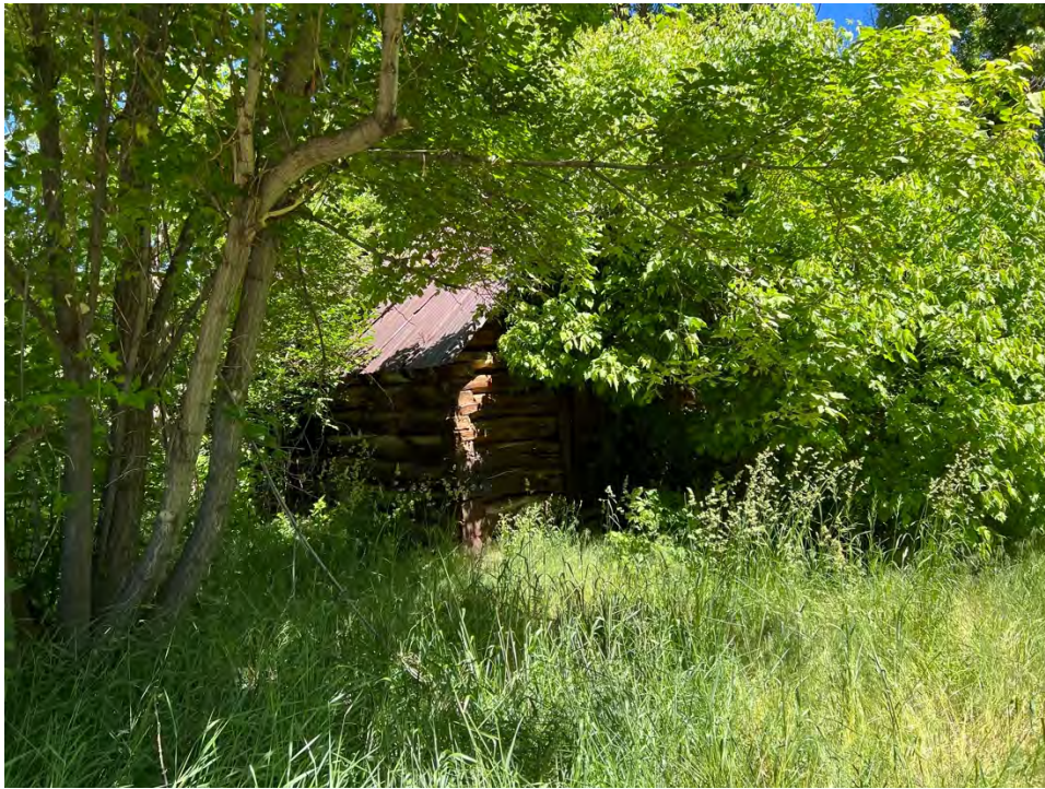
Photo 35 • Log Building #1, looking northwest. June 2023
