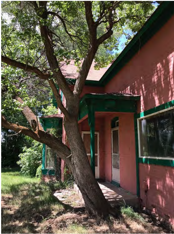
Photo 3 • Southwest Facade, looking west. July 2022
