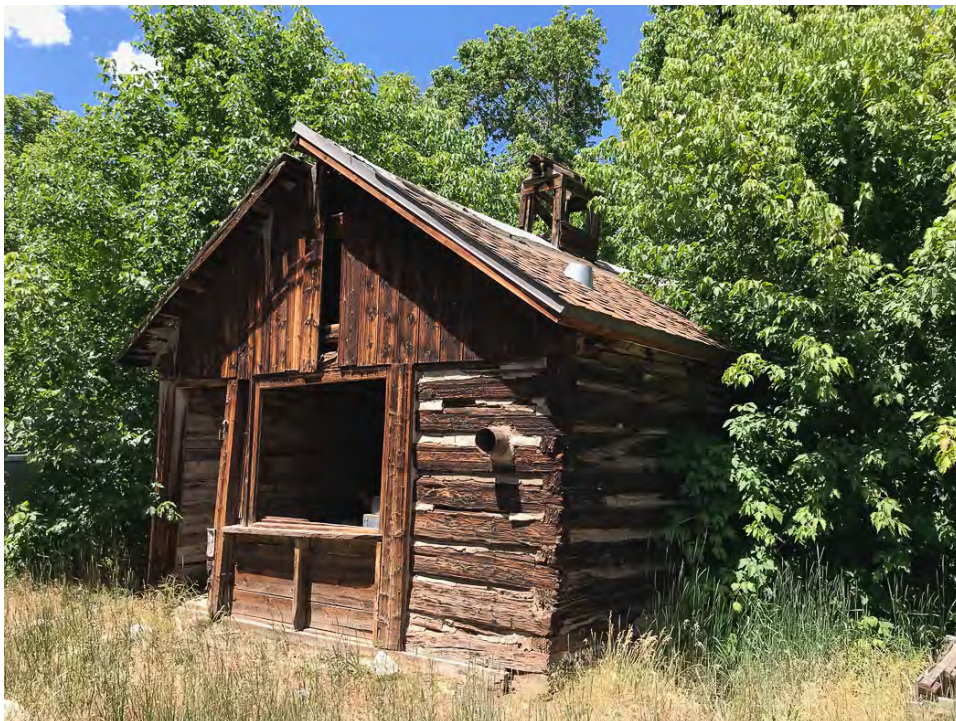
Photo 29 • Log building #2, aka Bunkhouse. South facade, looking north. July 2022
