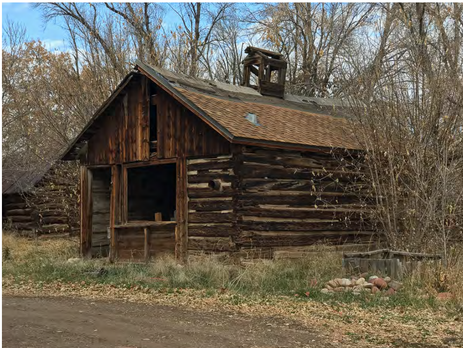
Photo 30 • Log building #2, looking north. November 2021
