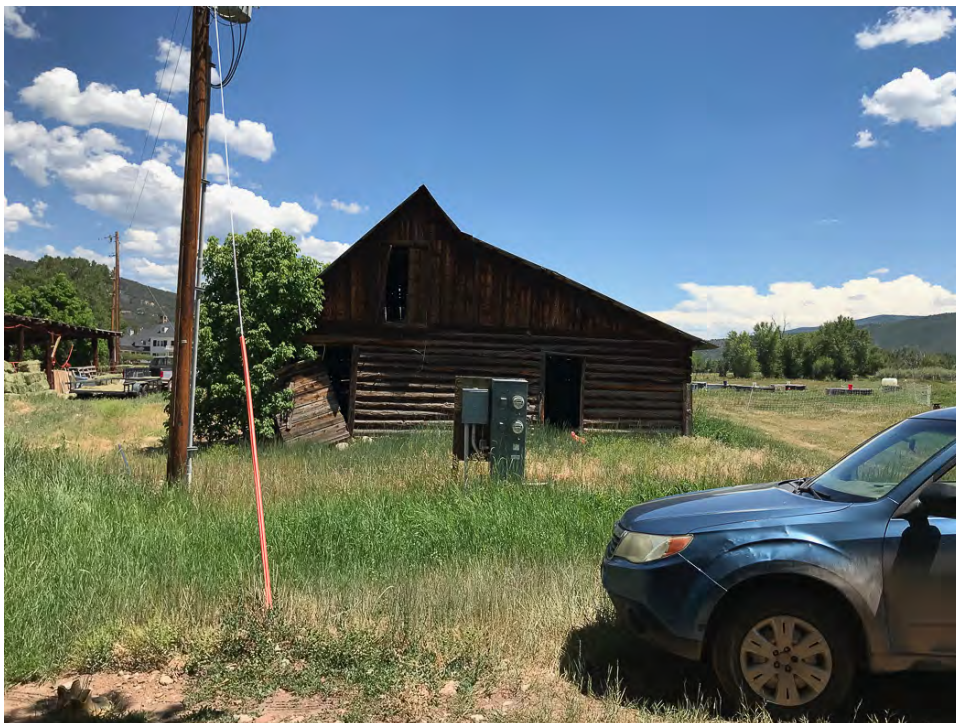
Photo 12 • Log Barn northwest facade (main) looking southeast. July 2022
