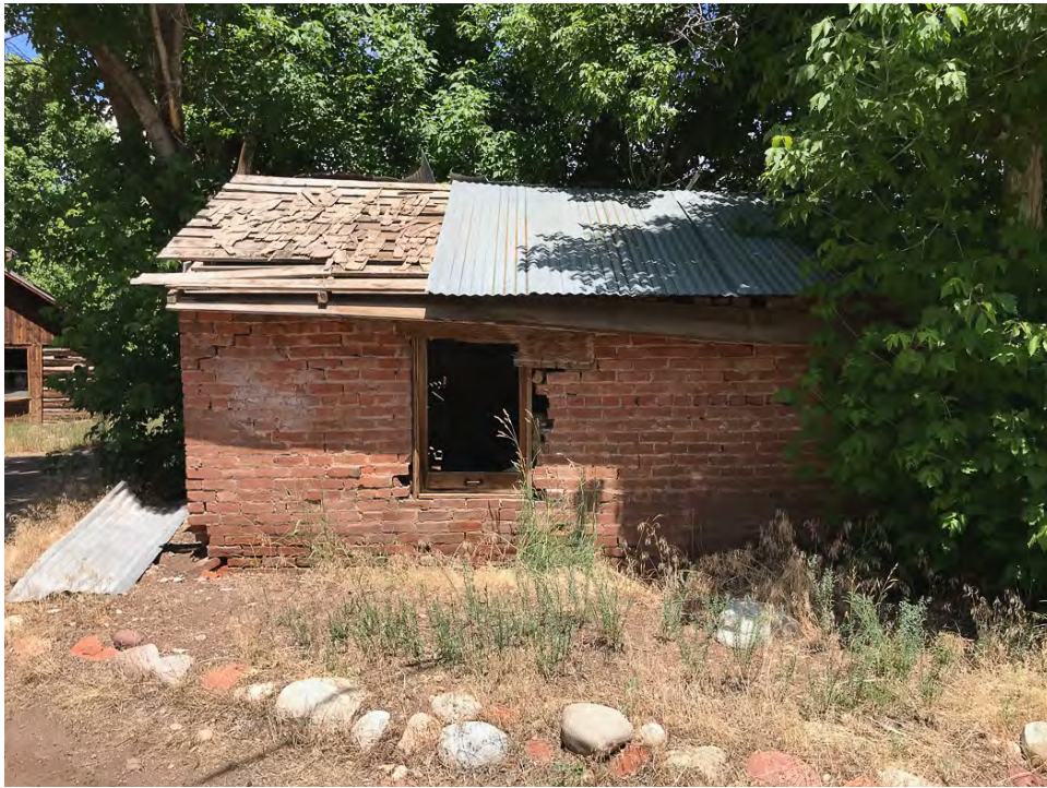
Photo 19 • Brick shed southwest facade, looking northeast. July 2022
