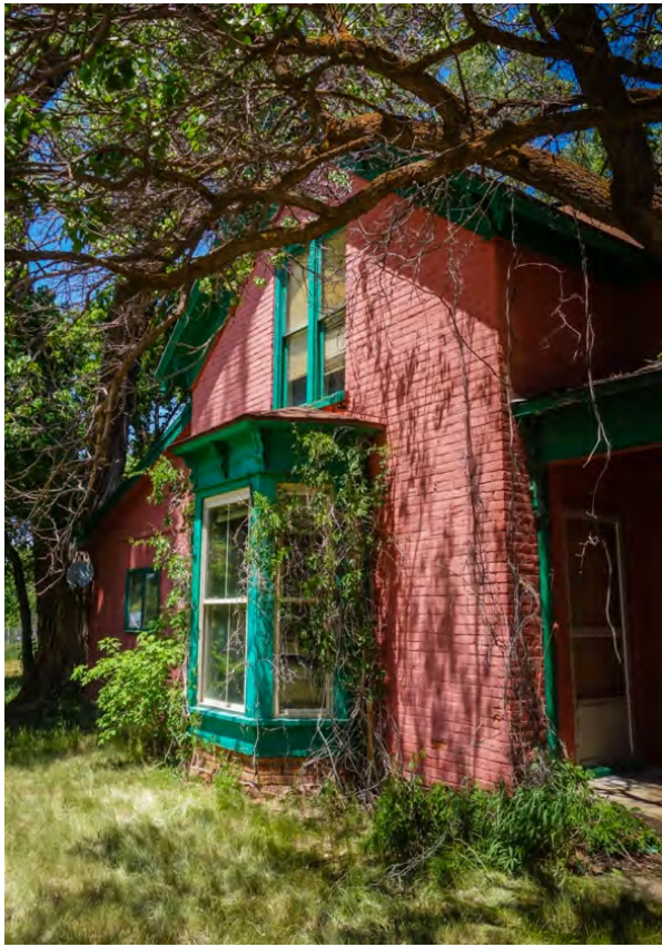
Photo 9 • Southwest Facade, detail of bay window. June 2017
