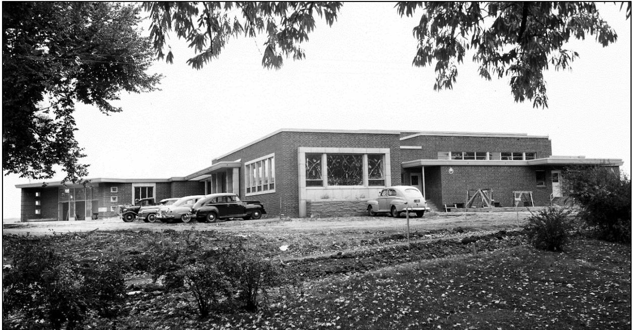
e. Machebeuf Hall east and northeast elevations, 1950, facing southwest, Sisters Dining Room at northeast corner (LHC).
