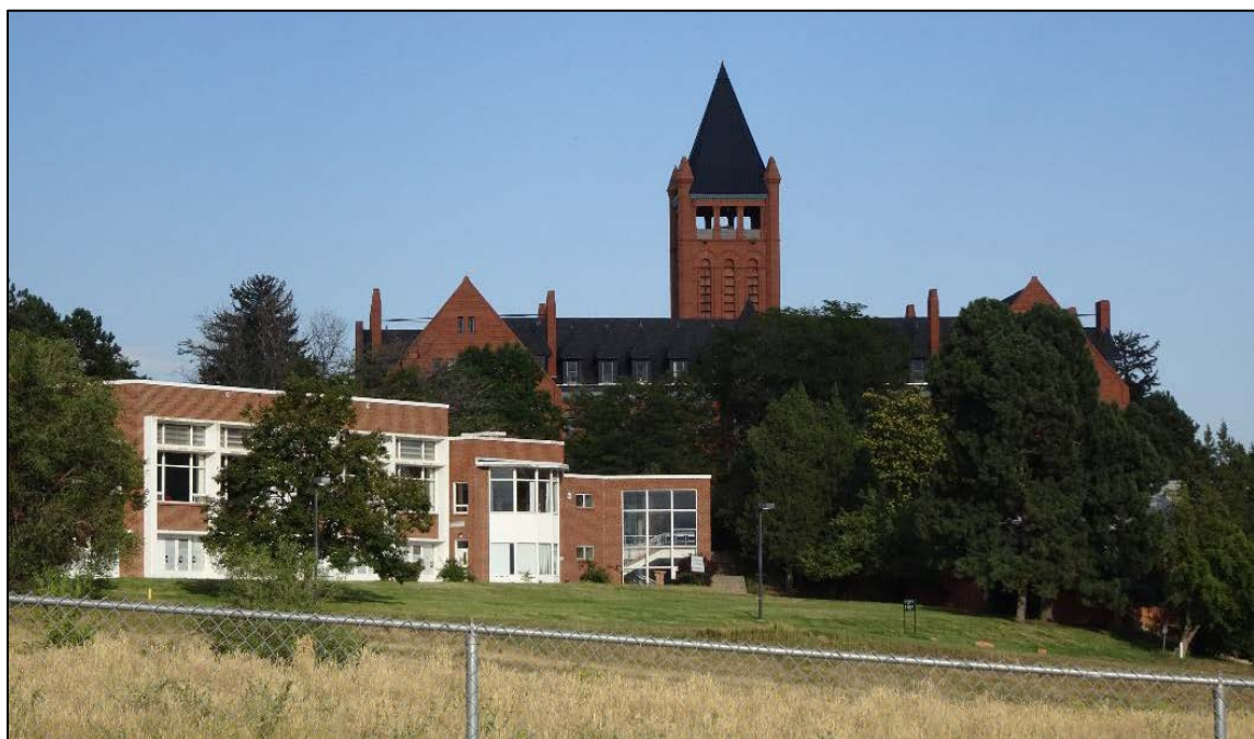
b. Machebeuf Hall southwest elevation, 2018, facing east, Ad. Building in background.
