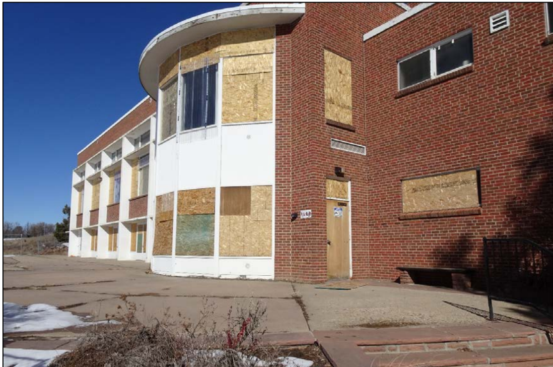
h. Machebeuf Hall southwest elevation, 2023, facing north-northwest.
