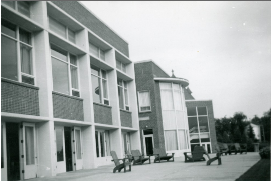
g. Machebeuf Hall southwest elevation, c. 1960, facing east (LHC).
