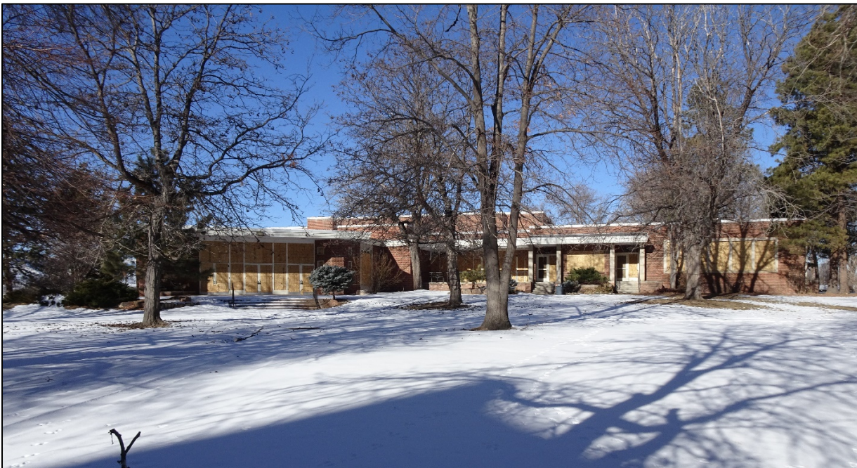
d. Machebeuf Hall east elevation, 2023, facing west, “Quad” landscape in foreground. Windows are protected by plywood—in all 2023 photographs—to secure the building during surrounding former-campus redevelopment.
