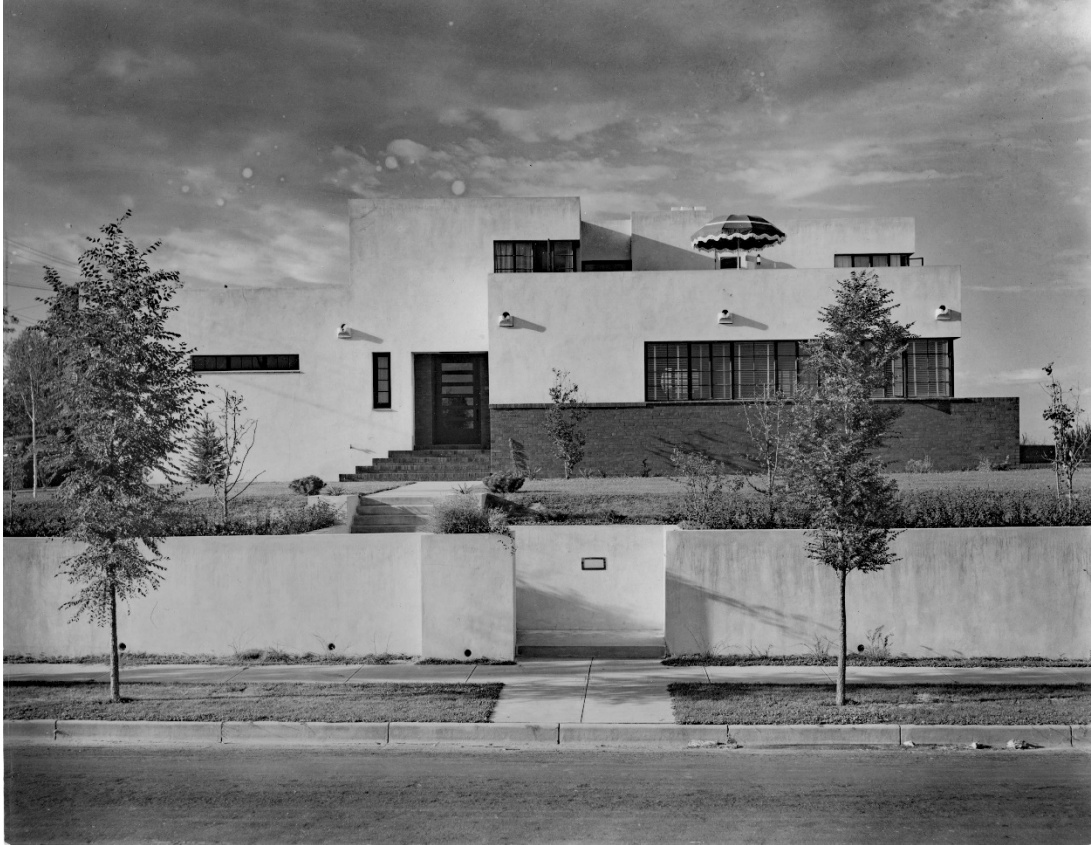
Figure 2. The front (south wall) of the completed house is shown in this circa 1936-37 photograph (view north). SOURCE: Frank Hegner photograph collection, on file Carol and Tom Amy, Denver, Colorado.
