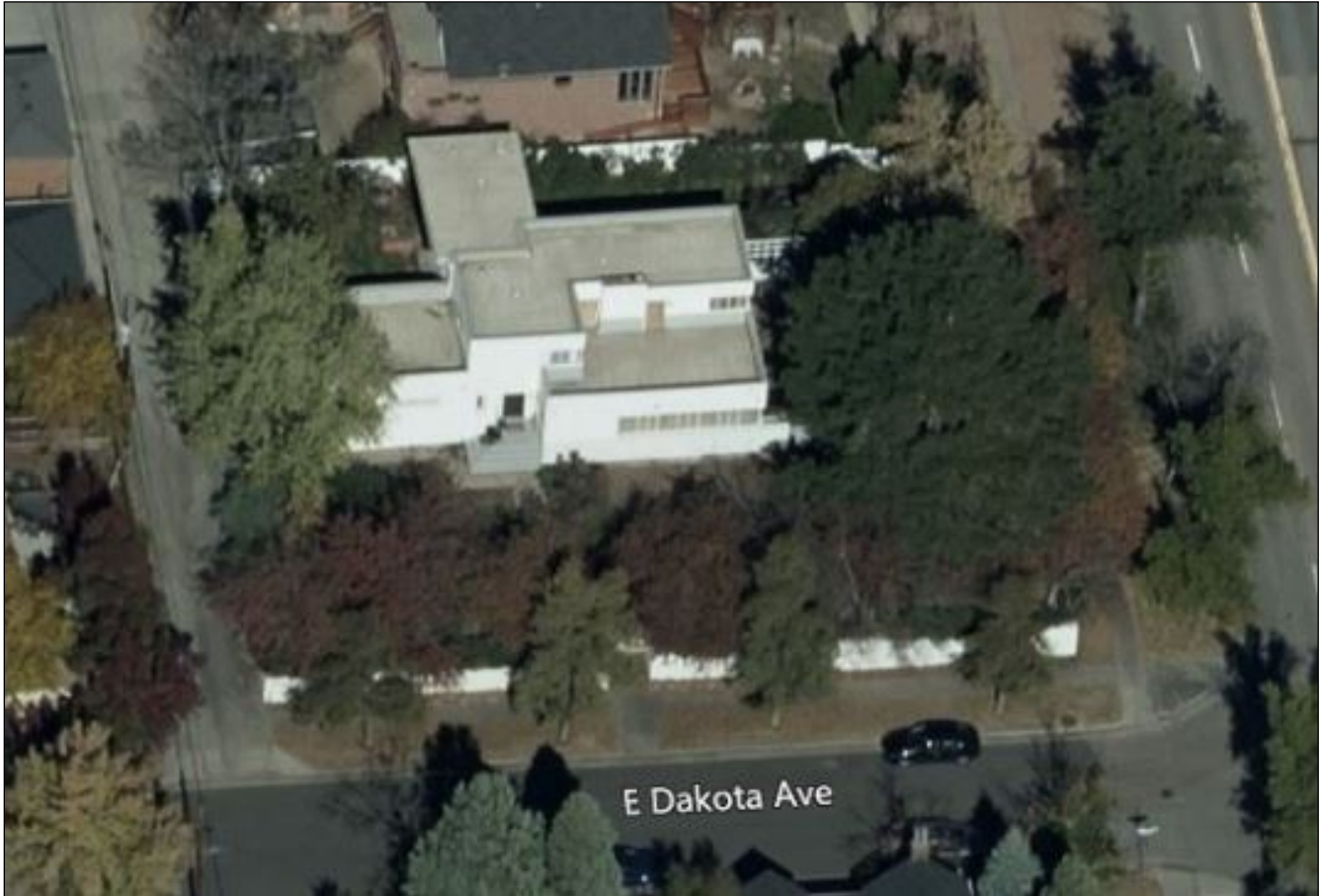
Figure 1. This oblique aerial photograph (view north-northeast) provides an overview of the parcel and the Hegner House plan. East Dakota Avenue is at the bottom, South University Boulevard is to the right, and the public alley is to the left. SOURCE: Bing Maps birds-eye-view photograph, undated, Denver, Colorado.
