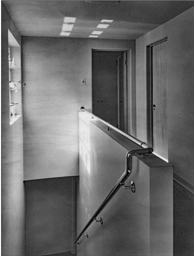
Figure 9. This ca. 1937 photograph (view west-northwest) shows the stairs to the second story with their stainless steel rail. This view appeared in Architectural Forum in April 1937. SOURCE: Frank Hegner photograph collection, on file Carol and Tom Amy, Denver, Colorado.
