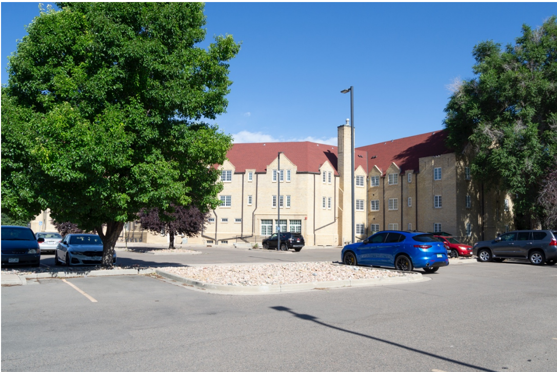
CO_Denver_CWC_0026: Porter Hall, southeast-east elevation, facing northwest
