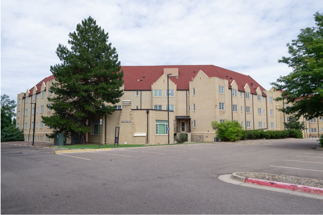
CO_Denver_CWC_0019: Curtis Hall, east elevation, facing west
