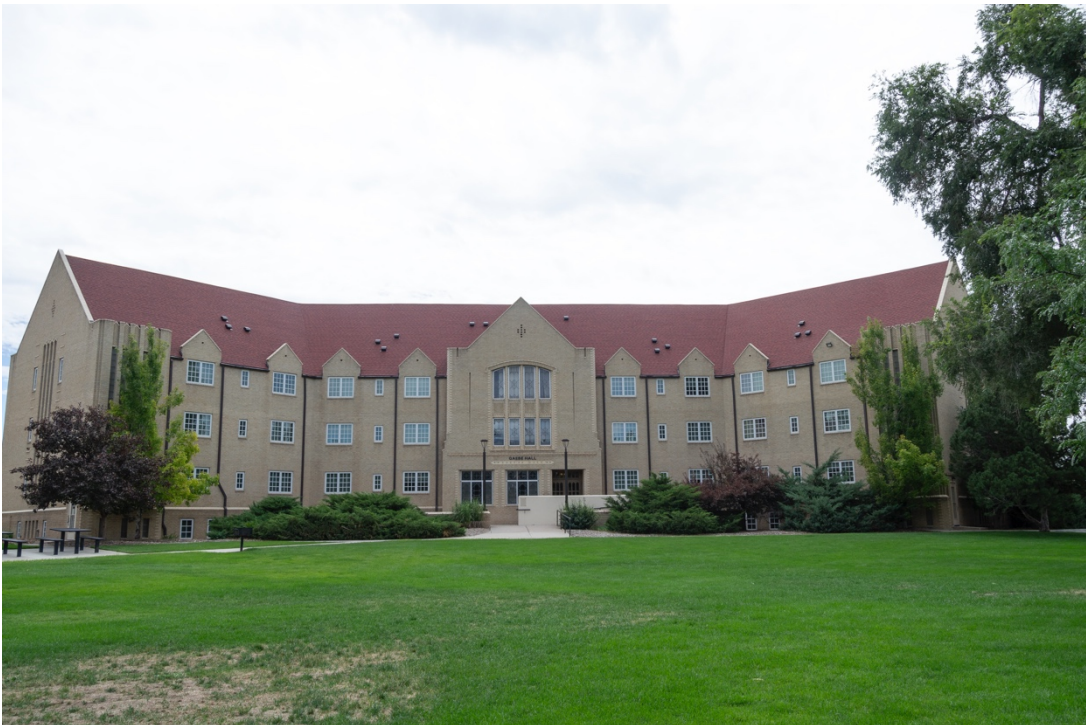
CO_Denver_CWC_0018: Curtis Hall, northwest elevation, facing southeast
