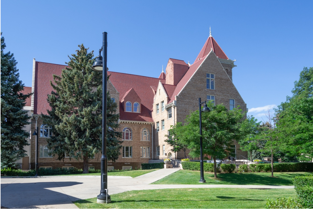
CO_Denver_CWC_0029: Treat Hall, northeast corner, facing southwest
