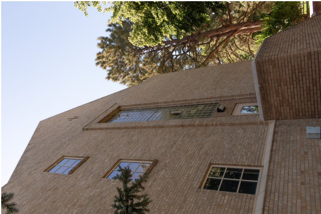
CO_Denver_CWC_0058: Pulliam Hall, west elevation, facing southeast
