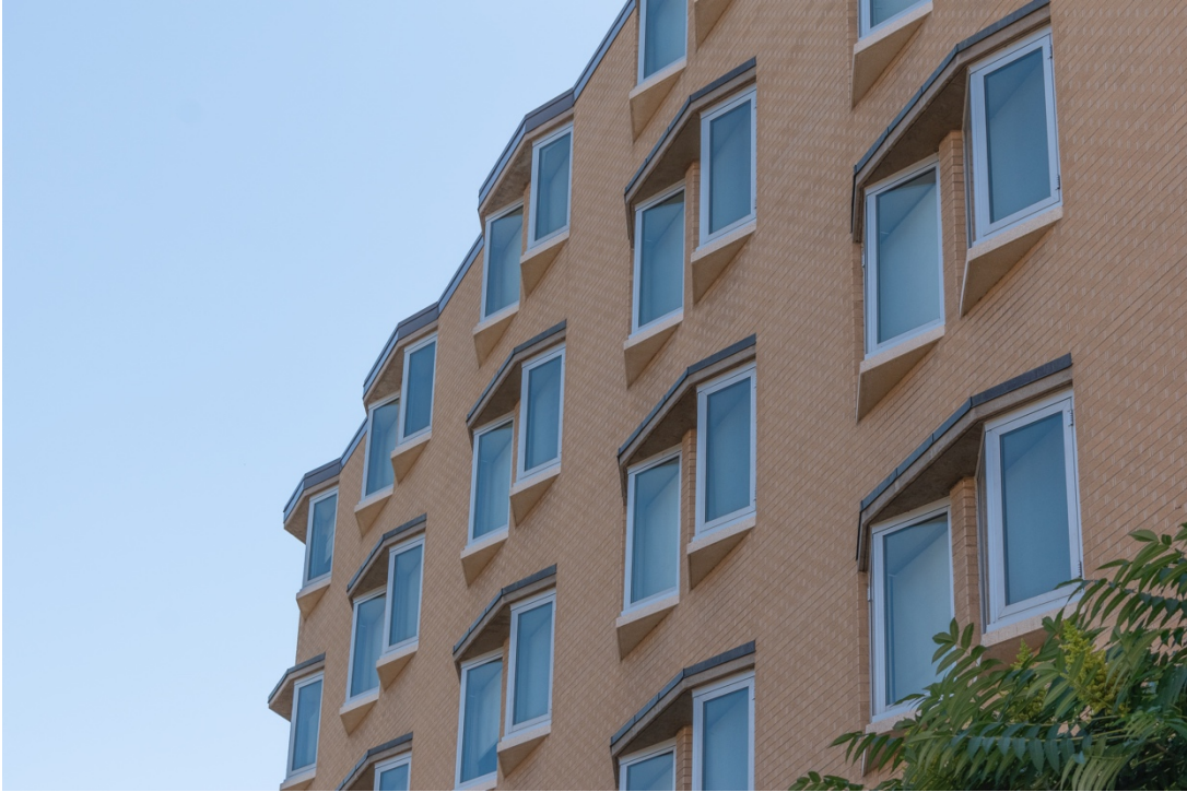
CO_Denver_CWC_0047: Dunklee Hall, northwest elevation window detail, facing northeast
