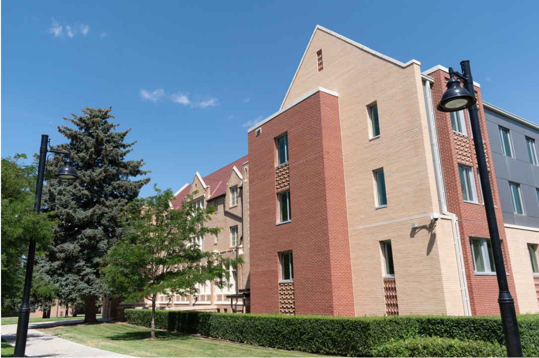
CO_Denver_CWC_0035: Foote Hall, southeast corner, facing northwest
