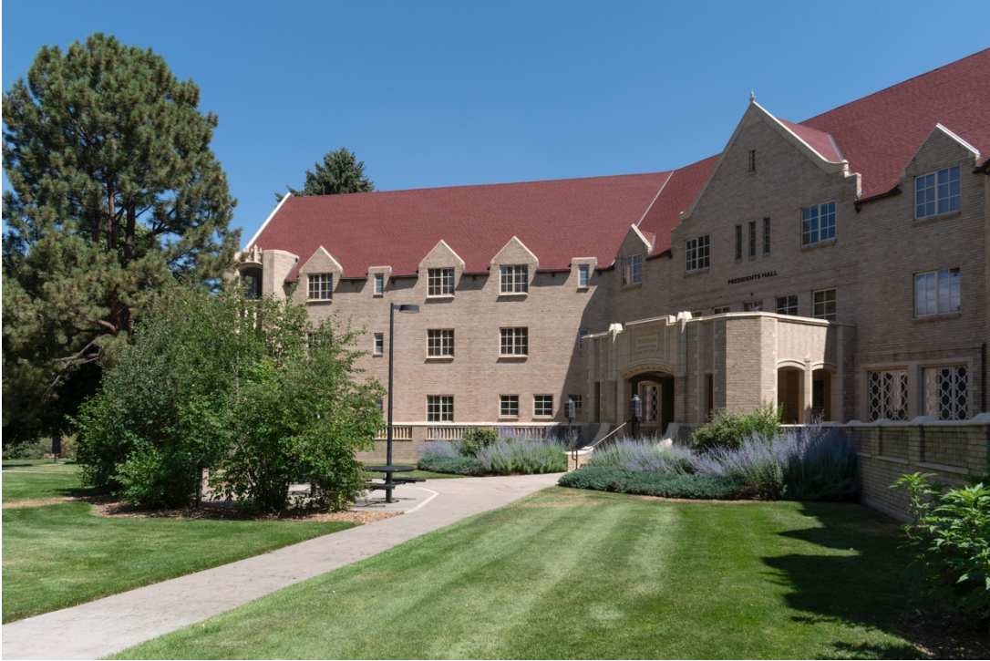
CO_Denver_CWC_0055: Pulliam Hall, south and southwest elevations, facing north
