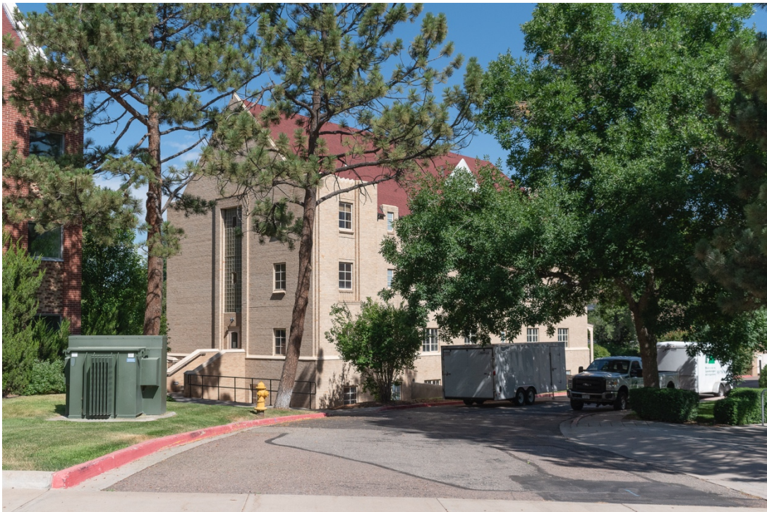
CO_Denver_CWC_0054: Pulliam Hall, south and east elevations, facing northwest
