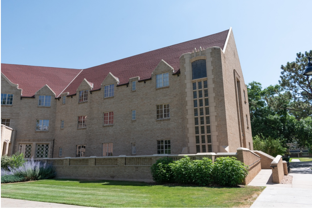
CO_Denver_CWC_0057: Pulliam Hall, west elevation, facing northeast
