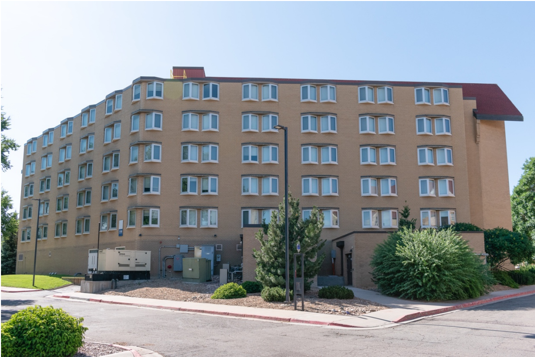
CO_Denver_CWC_0042: Dunklee Hall, north and northwest elevations, facing south
