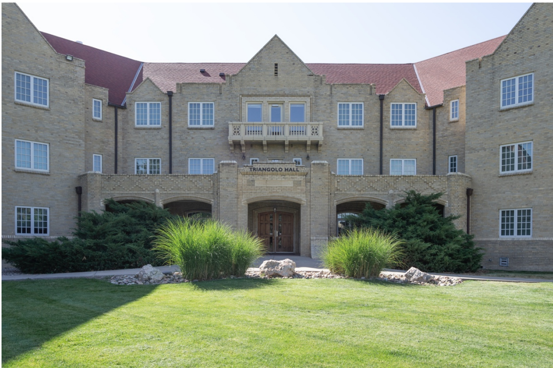
CO_Denver_CWC_0022: Porter Hall, main entrance on the northwest elevation, facing southeast
