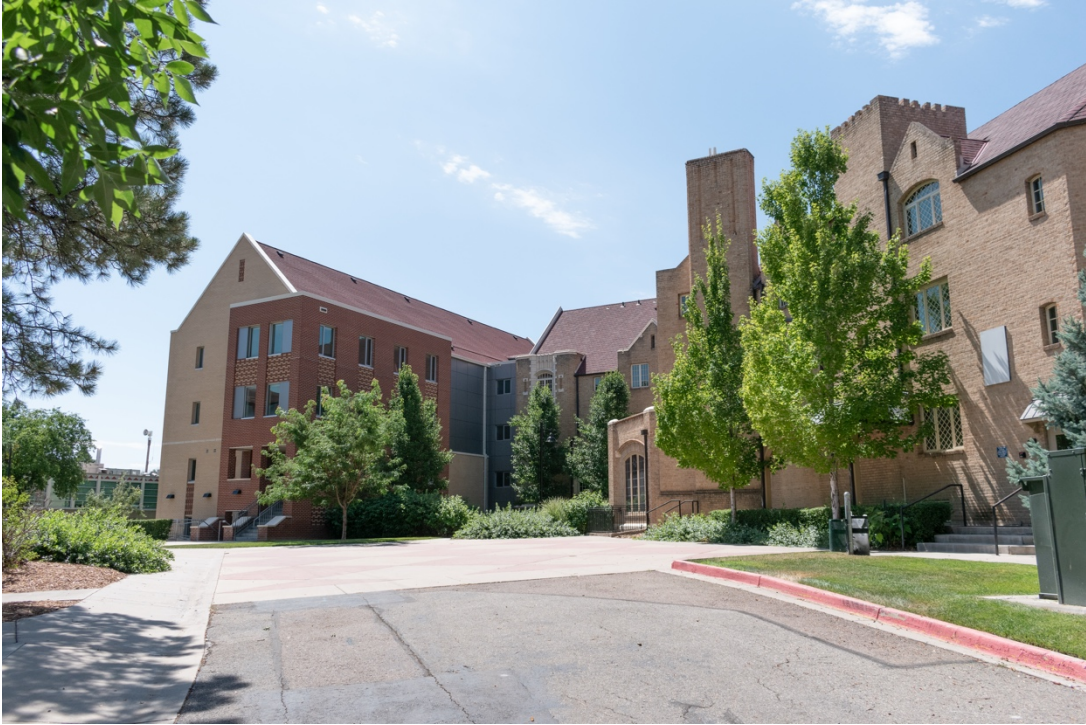
CO_Denver_CWC_0031: Foote Hall, north elevation, facing southeast
