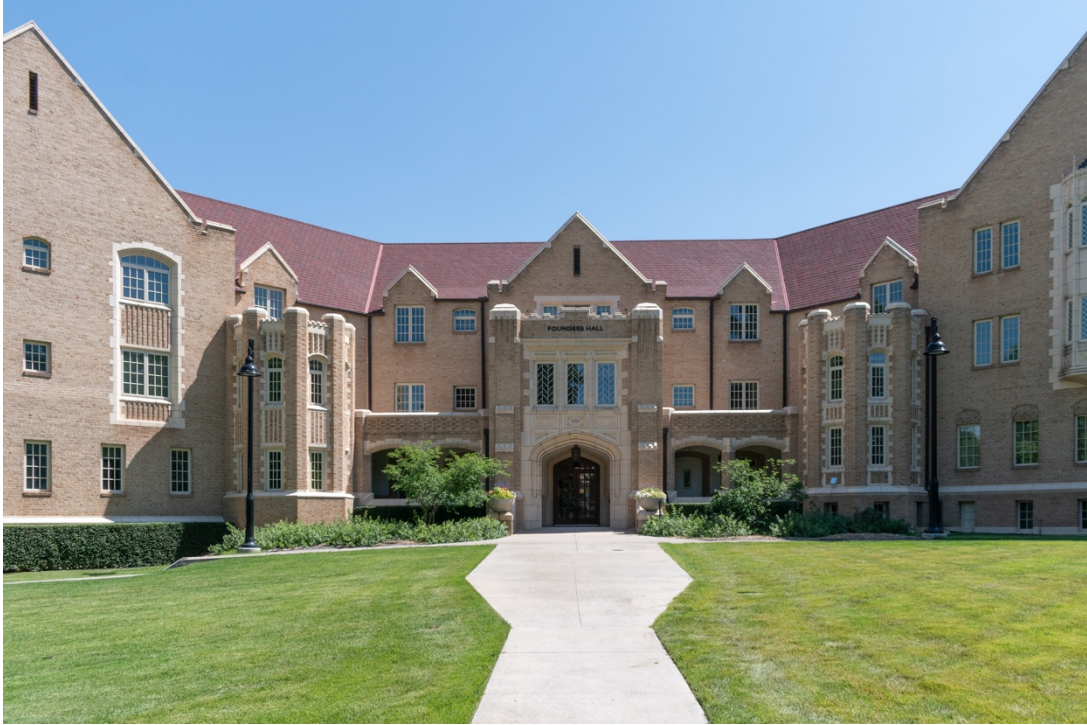
CO_Denver_CWC_0037: Foote Hall, southwest elevation, facing northeast
