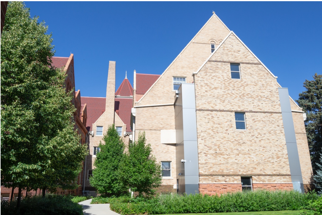
CO_Denver_CWC_0030: Treat Hall, east elevation, facing west
