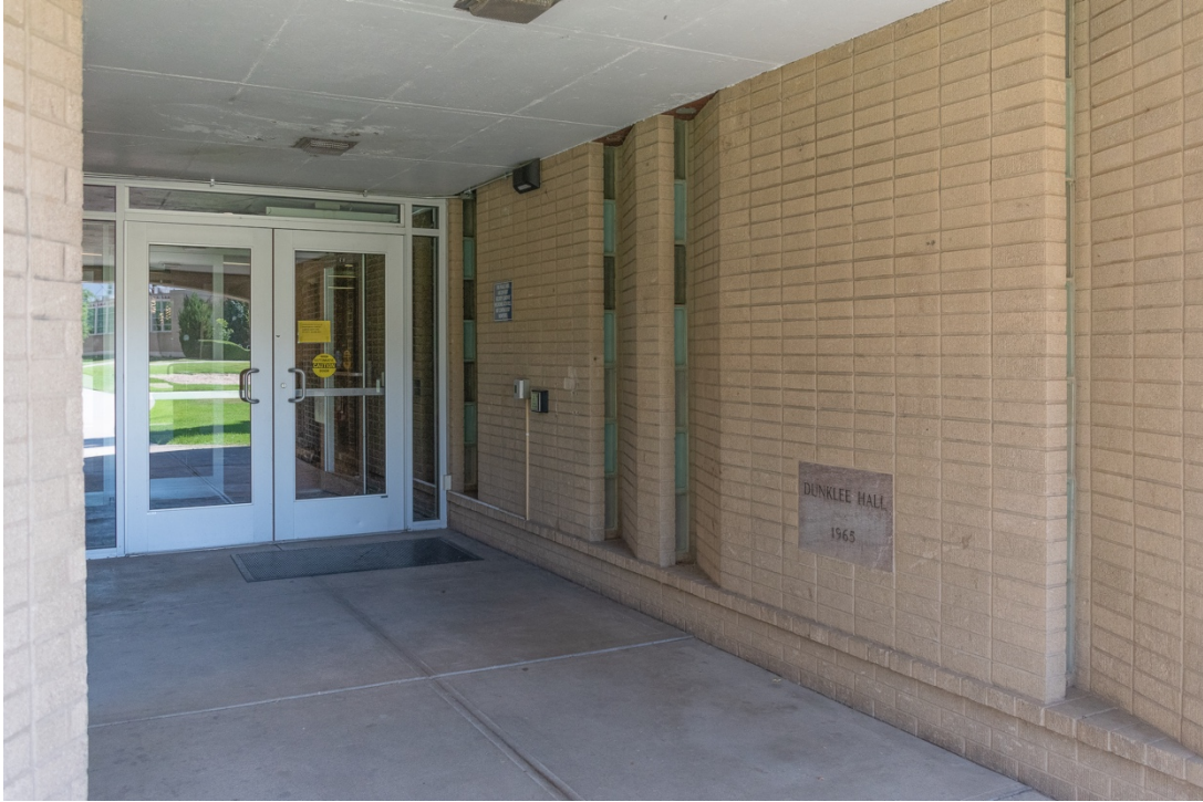
CO_Denver_CWC_0045: Dunklee Hall, entrance at west end of south elevation, facing northeast
