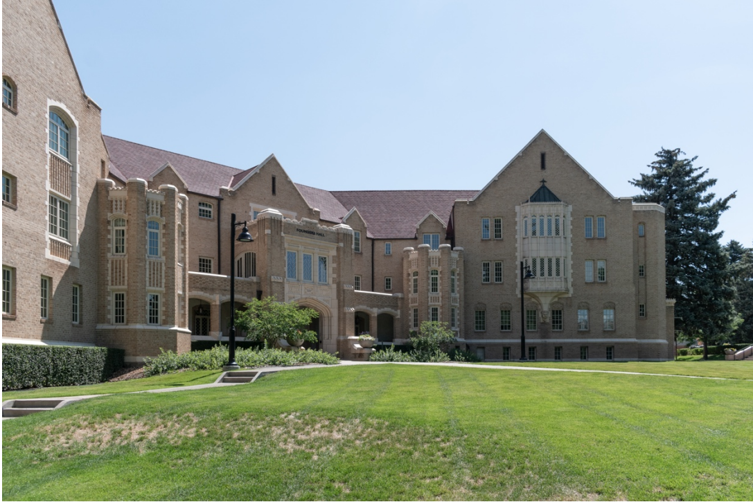
CO_Denver_CWC_0039: Foote Hall, west and southwest elevations, facing east
