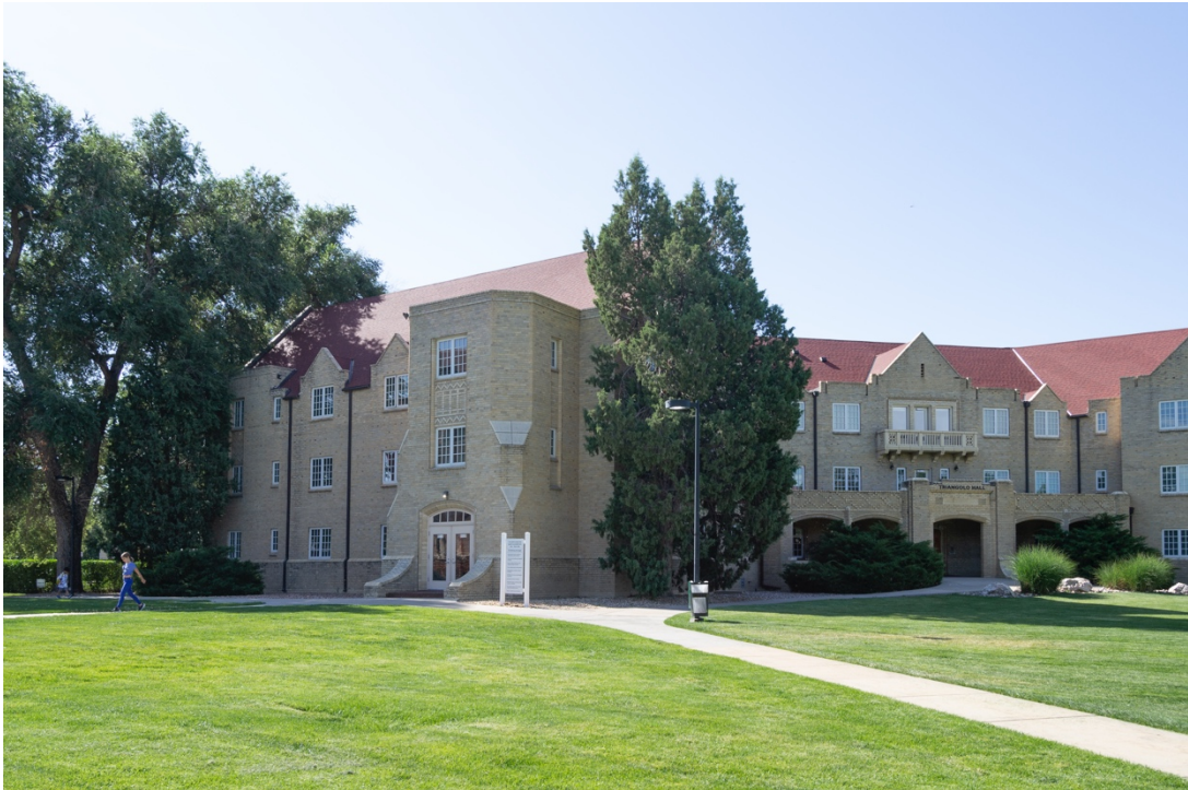
CO_Denver_CWC_0024: Porter Hall, northeast-east elevation, facing southwest
