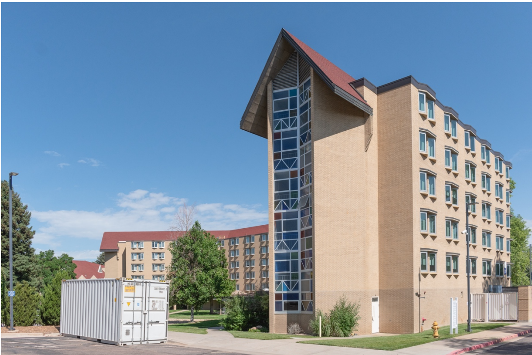
CO_Denver_CWC_0016: Southeast corner boundary near Dunton Hall, facing northwest
