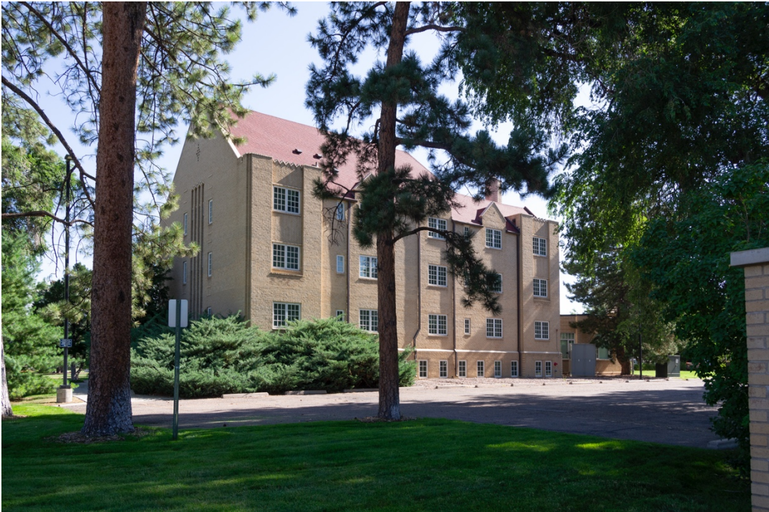
CO_Denver_CWC_0020: Curtis Hall, south elevation, facing north
