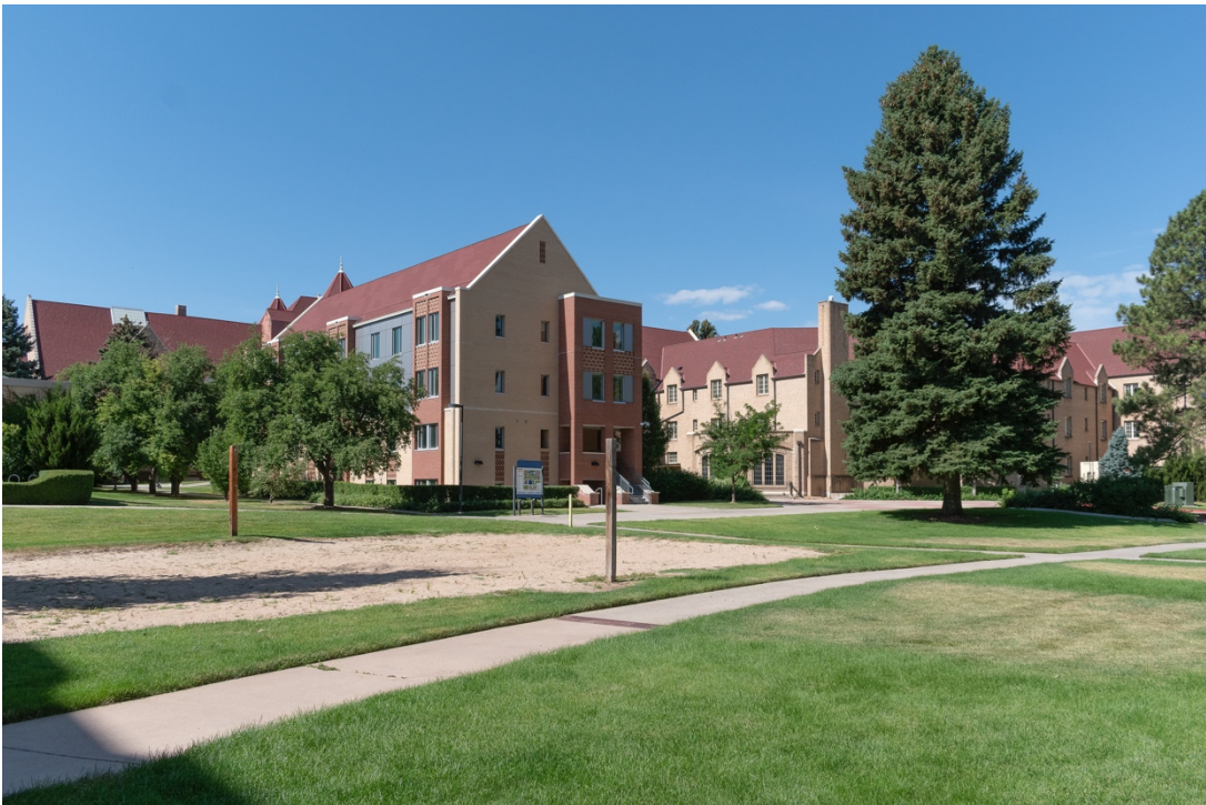
CO_Denver_CWC_0032: Foote Hall, north and east elevations, facing southwest
