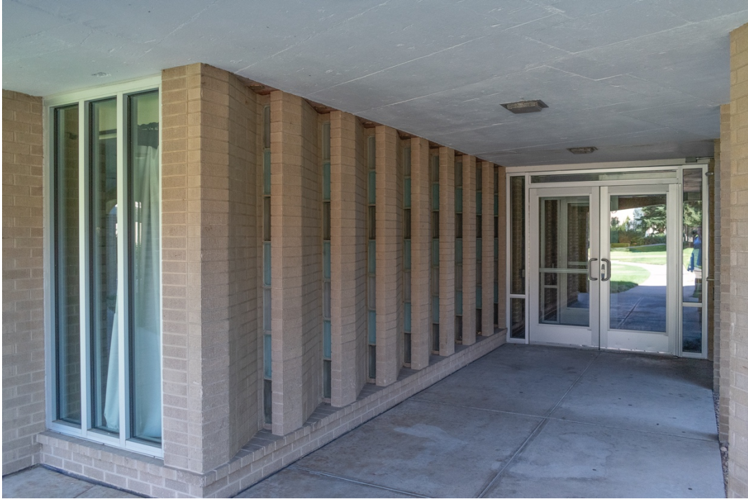
CO_Denver_CWC_0051: Dunton Hall, entrance on east elevation, windows detail
