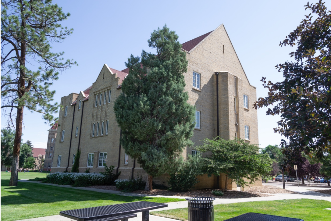
CO_Denver_CWC_0025: Porter Hall, west and south elevations, facing northeast
