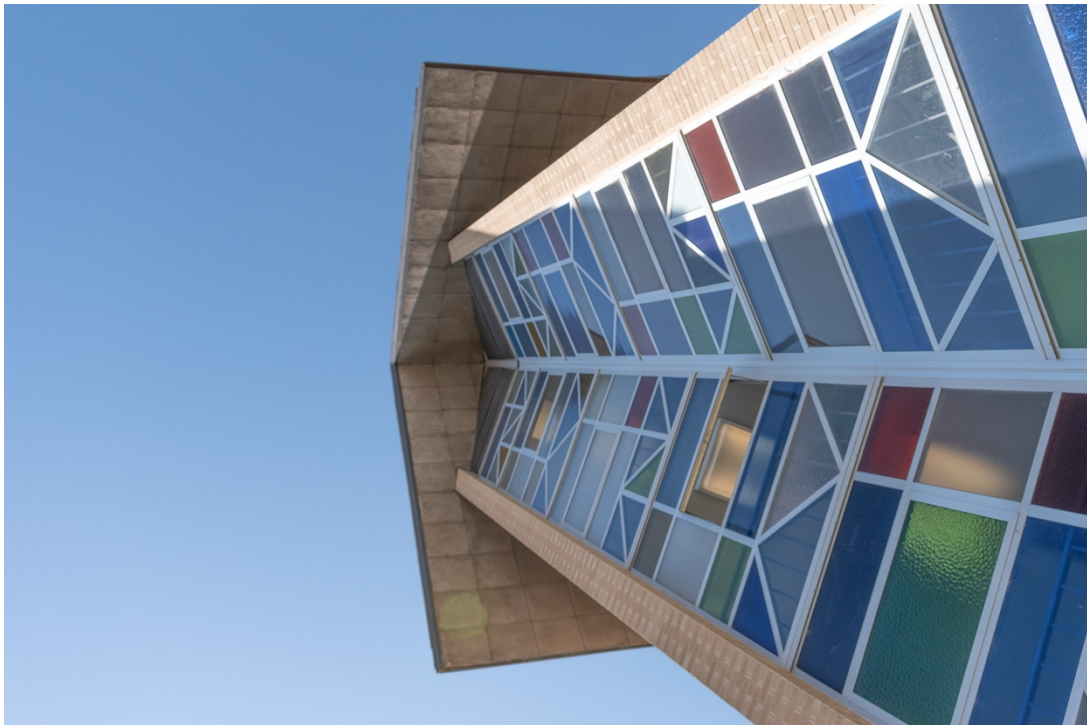
CO_Denver_CWC_0052: Dunton Hall, south stair tower detail
