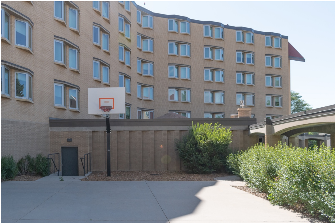
CO_Denver_CWC_0050: Dunton Hall, west and southwest elevations, facing southeast
