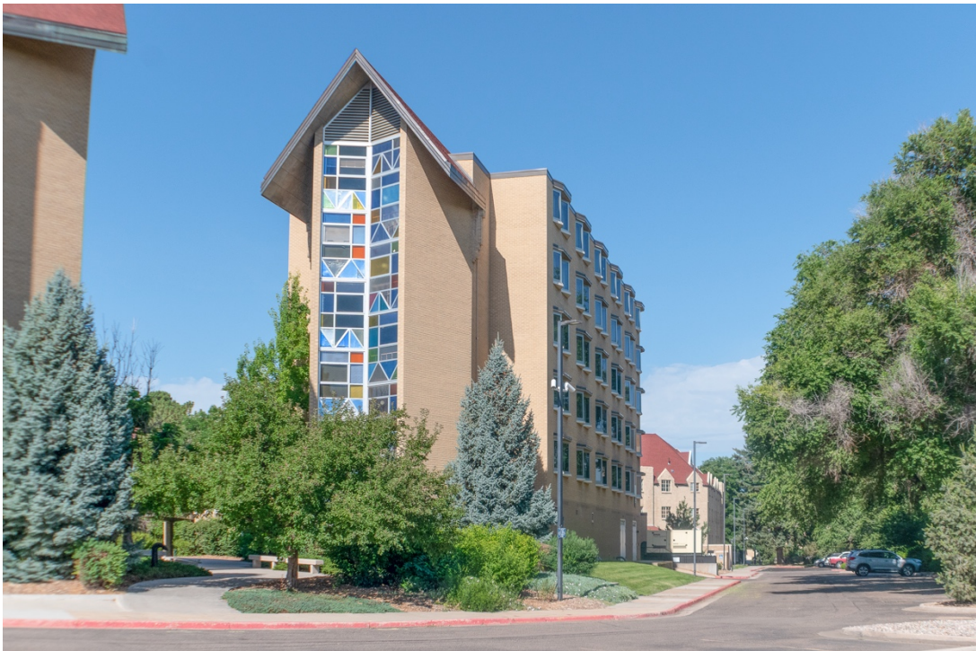
CO_Denver_CWC_0046: Dunklee Hall, north and east elevations
