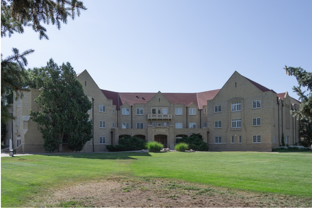
CO_Denver_CWC_0021: Porter Hall, northwest elevation, facing southeast
