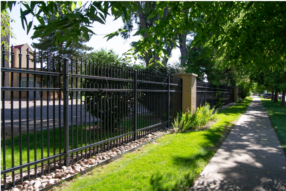
CO_Denver_CWC_0008: Fence (object) along south district boundary
