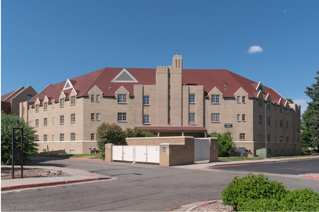
CO_Denver_CWC_0053: Pulliam Hall, east-northeast and north elevations, facing southwest
