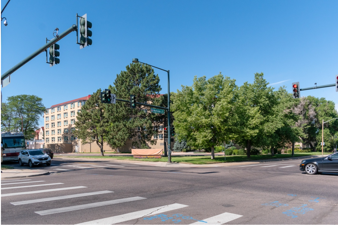
CO_Denver_CWC_0001: Northeast corner of campus, facing southwest
