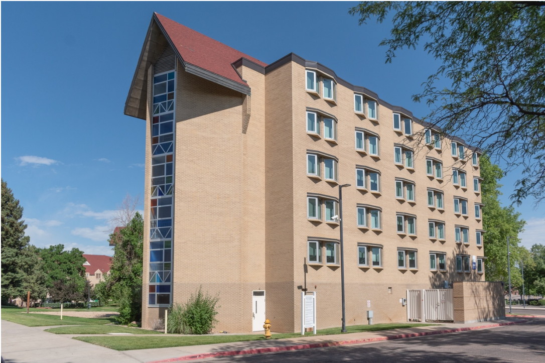
CO_Denver_CWC_0048: Dunton Hall, east and south elevations, facing northwest
