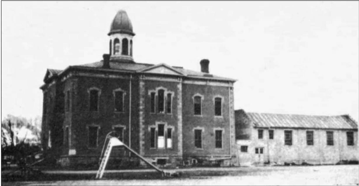
Figure 16. The east wall of the courthouse (left) and gymnasium (right) appear in this circa 1940s photograph. Note the playground equipment in the left foreground. SOURCE: Buena Vista High School, College Peaks Yearbook (1950).
