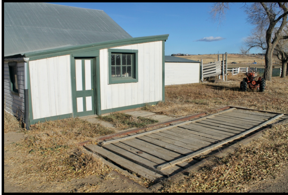
Photo 17 Scale House and Truck Scale. View to the Northeast.
