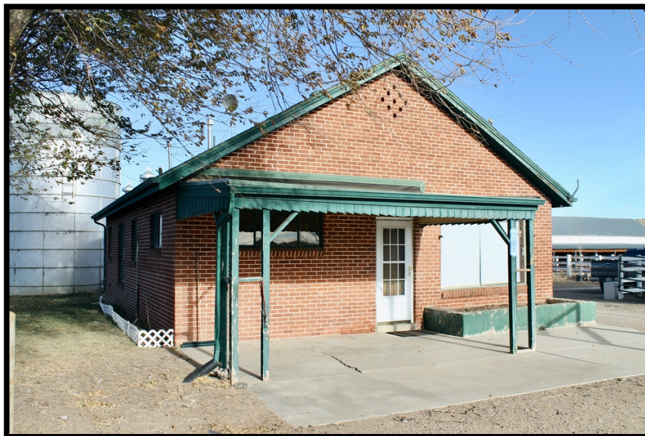
Photo 20 Milk Cooling House. View to the Northeast.
