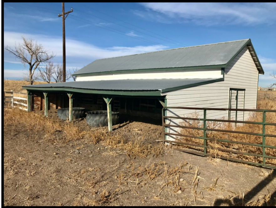
Photo 35 North Hay Barn and Loafing Shed. View to the North.
