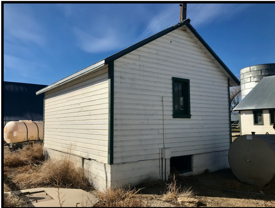
Photo 24 Water Pump House. View to the Southwest.
