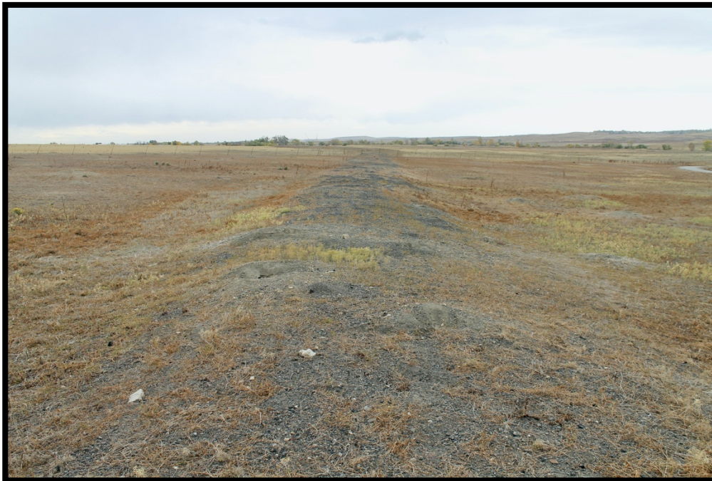
Photo 52 Colorado Central Railroad Segment. View to the Northeast.
