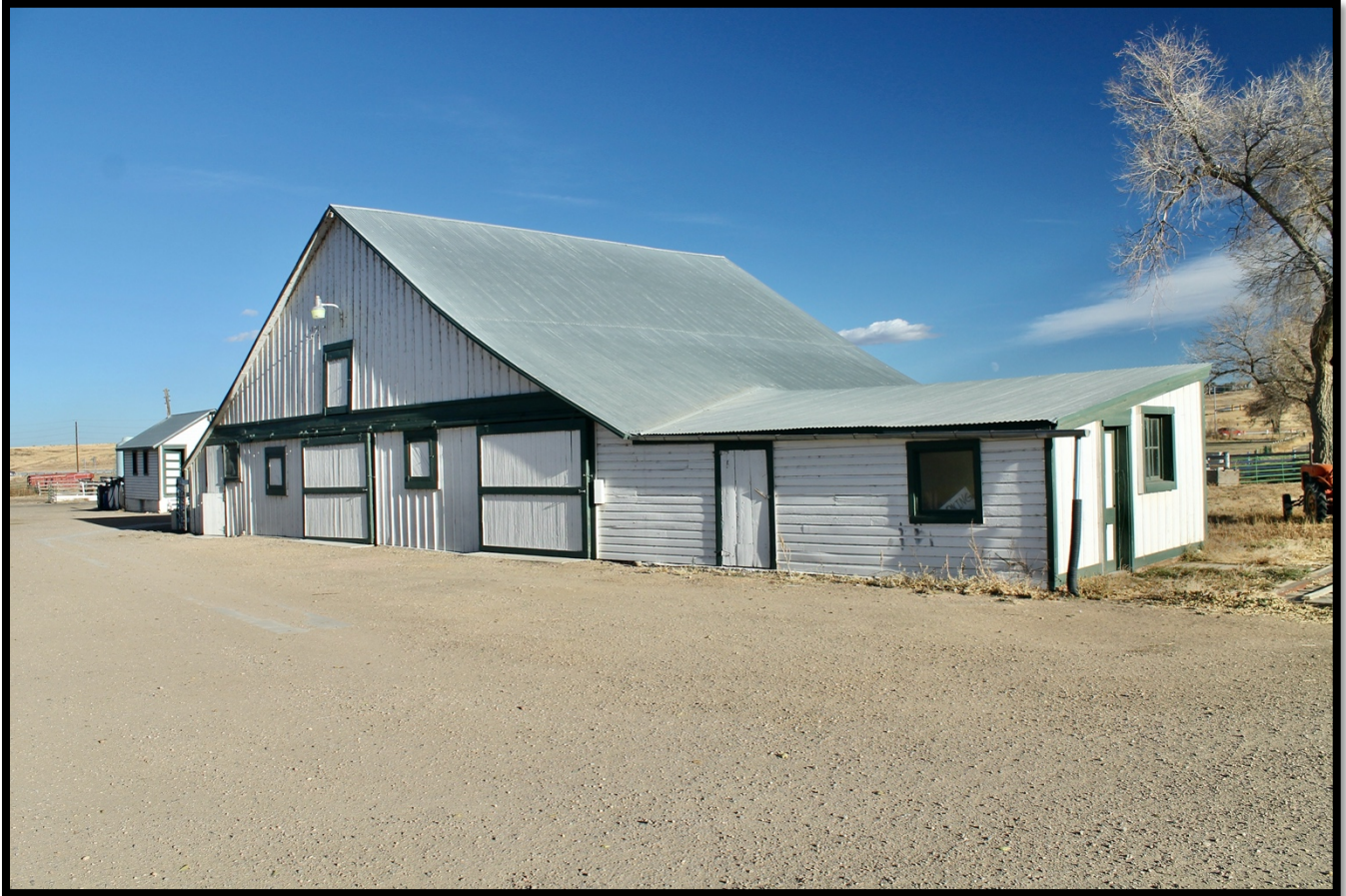
Photo 14 Horse Barn. View to the Northeast.
