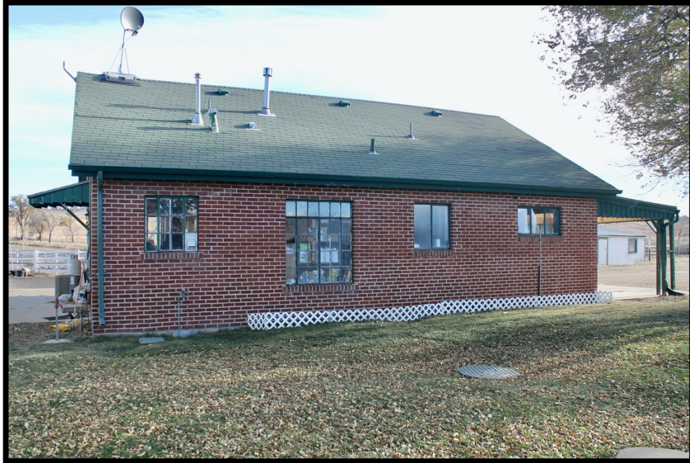
Photo 21 Milk Cooling House. View to the Southeast.
