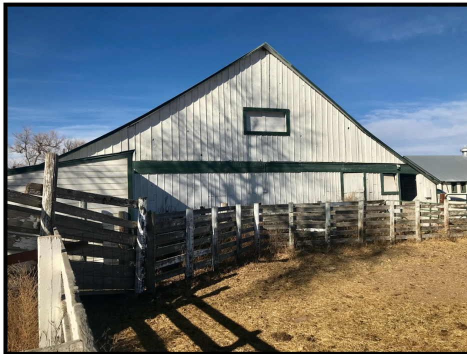
Photo 16 Horse Barn. View to the Northwest.
