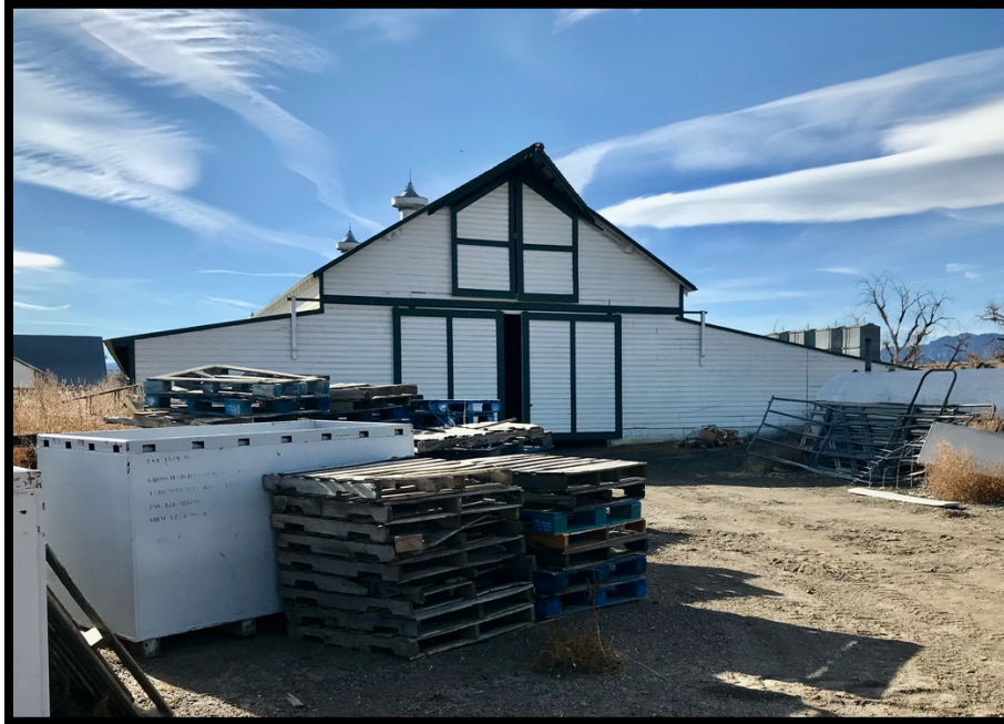
Photo 31 Feeding Barn. View to the Southwest.
