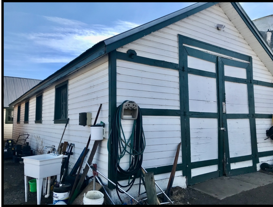
Photo 28 Milking Barn Annex. View to the Southeast.
