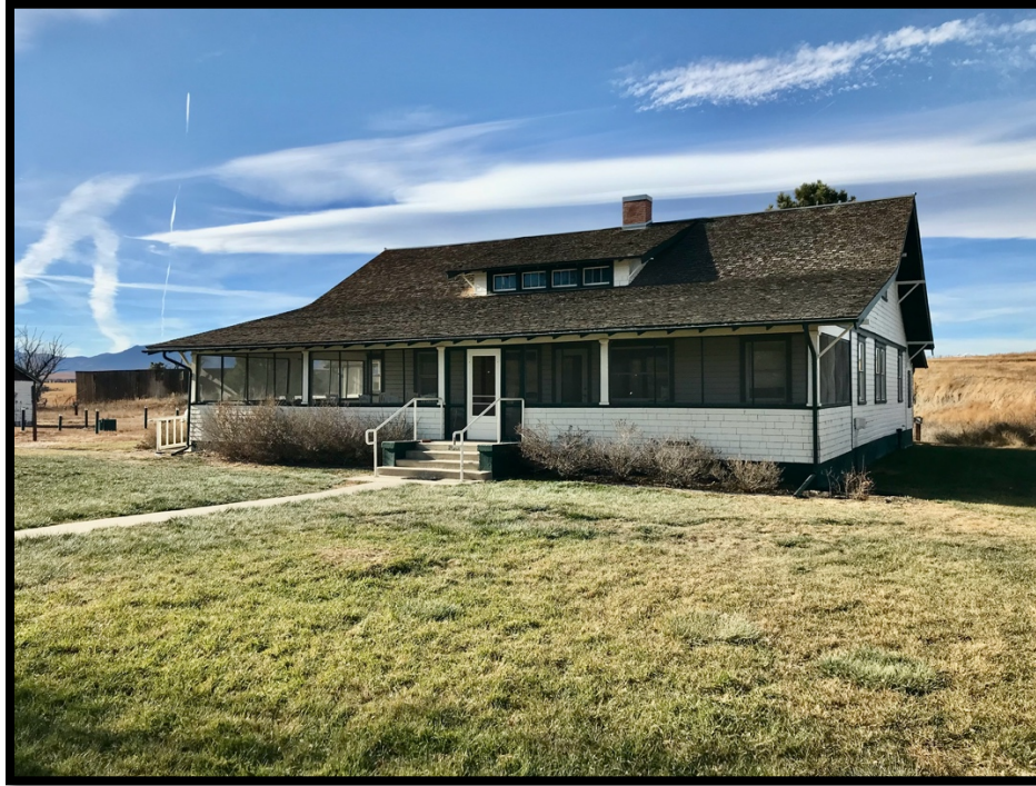
Photo 8 Goodhue House. View to the West.
