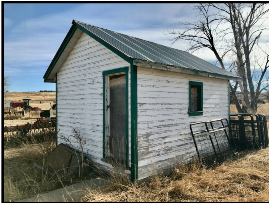
Photo 38 Old Well House. View to the Southeast.
