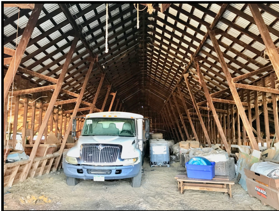
Photo 34 Feeding Barn Interior. View to the Southwest.
