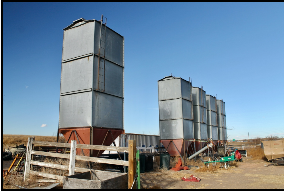
Photo 51 Cattle Feed Hoppers (Non-Contributing). View to the North.
