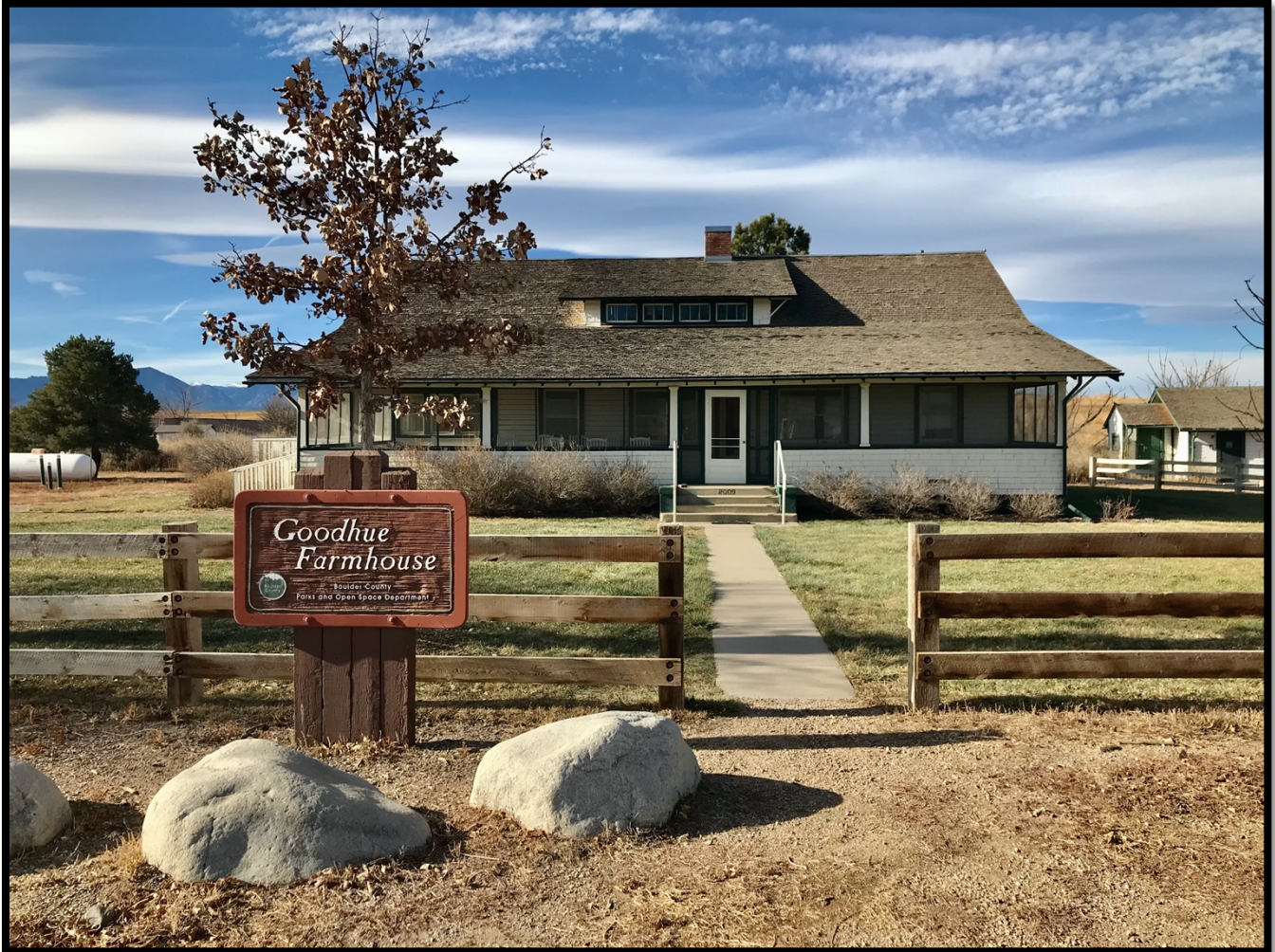
Photo 5 Goodhue Farmhouse. View to the Northwest.
