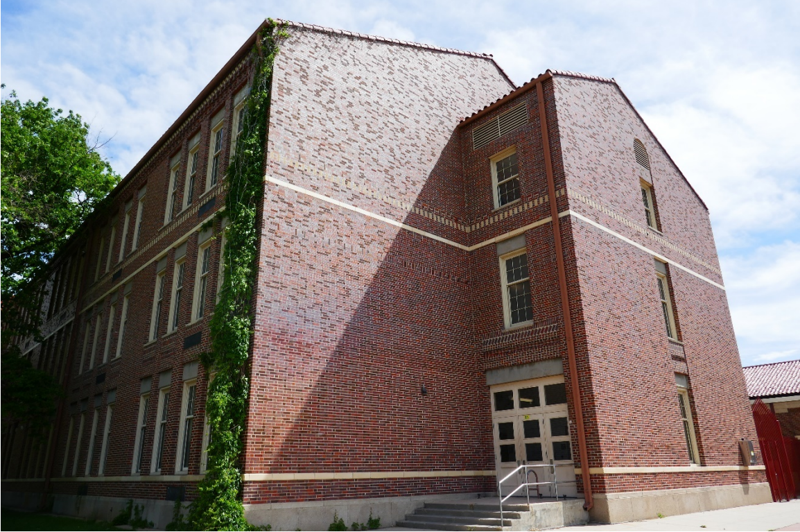
10 5/27/2022 Facing NNE Southwest corner of the south wing (1963 add.)
