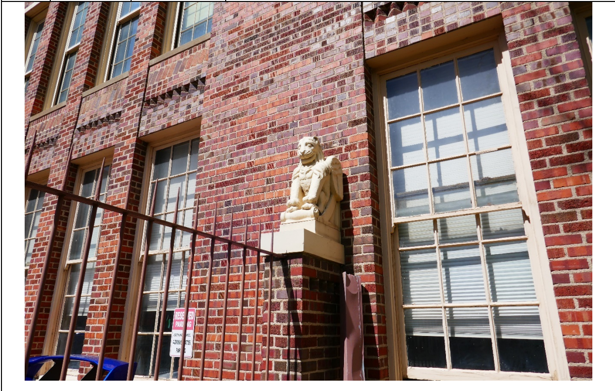
17 5/27/2022 Facing WSW Detail: Gargoyle at north parking lot fence
