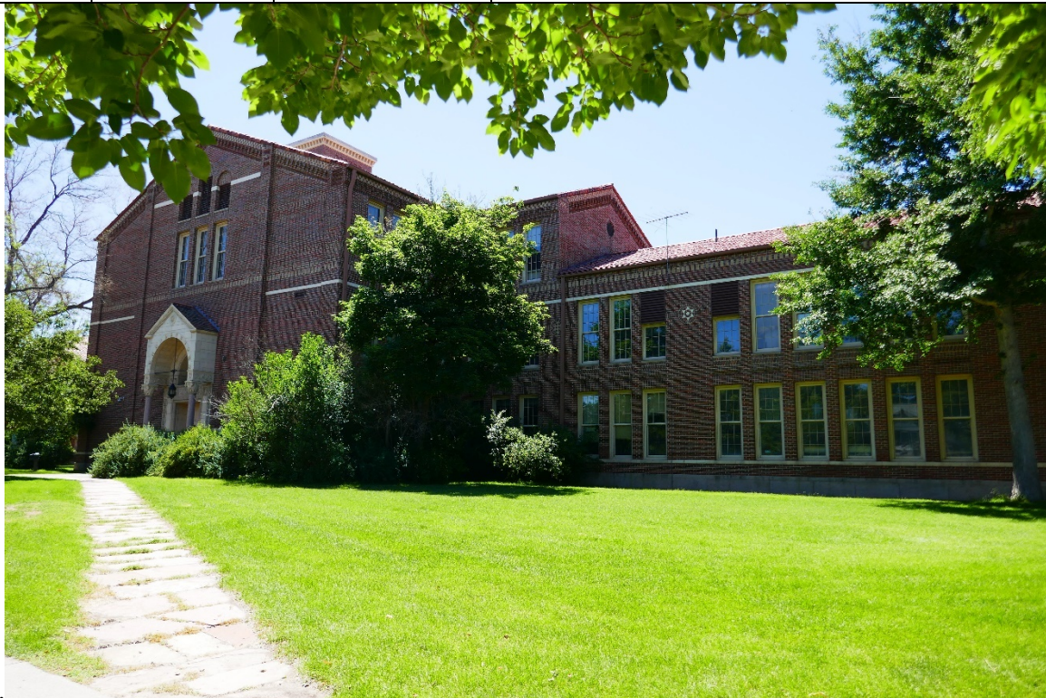
11 6/16/2022 Facing SW NW entrance and west end of north façade
