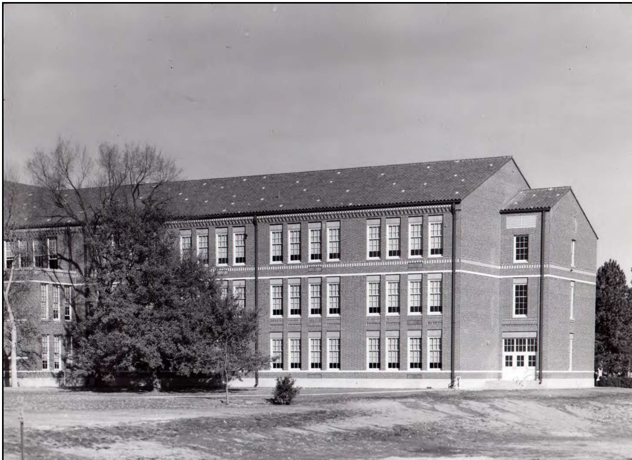
Figure 16. South addition to the high school, designed by Charles Gordon Lee and completed in 1963. Source: SHAFI collections. Charles Gordon Lee
