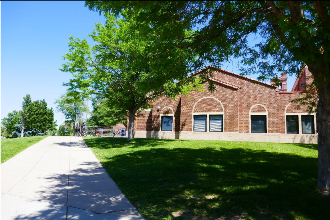
29 6/16/2022 Facing NW South façade of the 1989 Gym addition
