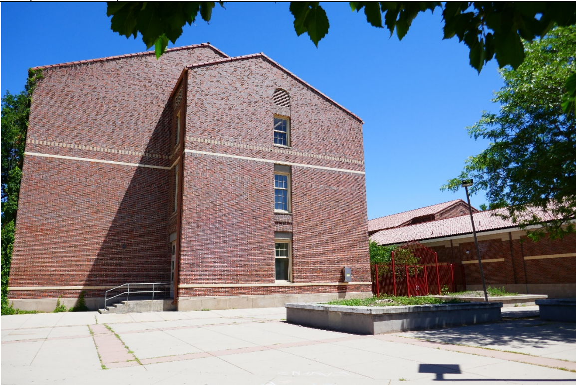
31 6/16/2022 Facing NE South façade of the 1963 addition and south gate to Senior Courtyard
