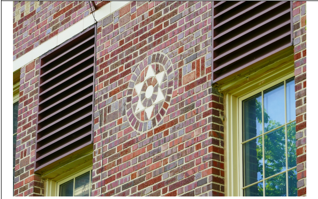
3 5/27/2022 Facing ENE Detail of brickwork, Star of David, north facade
