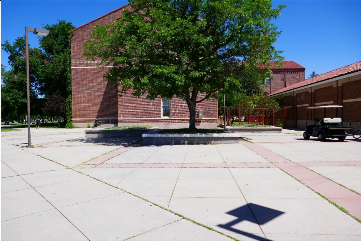
60 6/16/2022 Facing N Triangular landing area at the south end of the 1963 classroom addition, showing the three raised planters (noncontributing)
