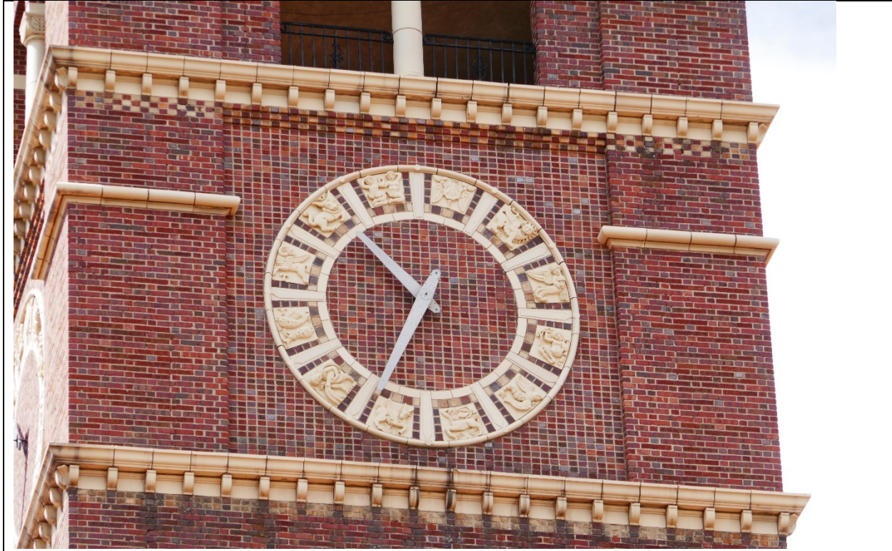
20 5/27/2022 Facing SSW Detail: Clock (north side of tower)
