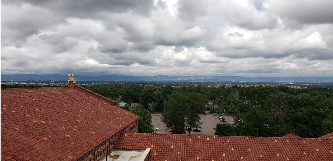
22 6/21/2021 Facing WSW View over the rooftop to the west from the clock tower
