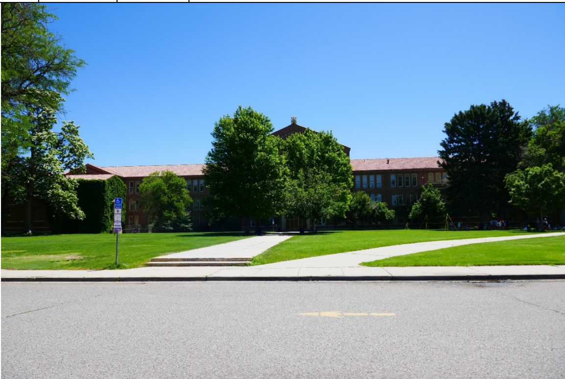
59 6/16/2022 Facing E West side of the resource boundary, showing wide walkway to main entrance from the west parking lot
