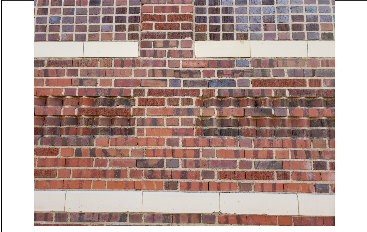
2 11/10/2020 Facing E Detail of brickwork, west facade
