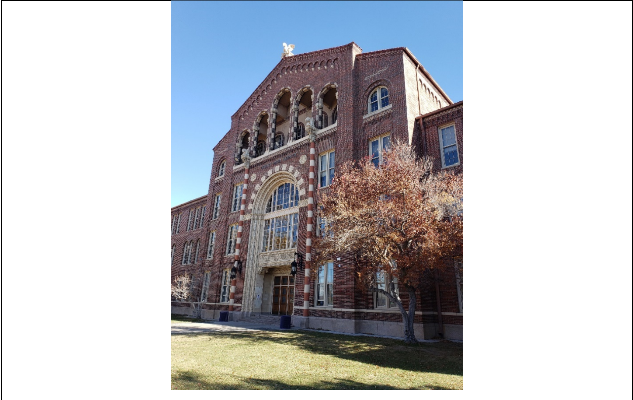
4 11/10/2021 Facing NE Primary façade and main entrance
