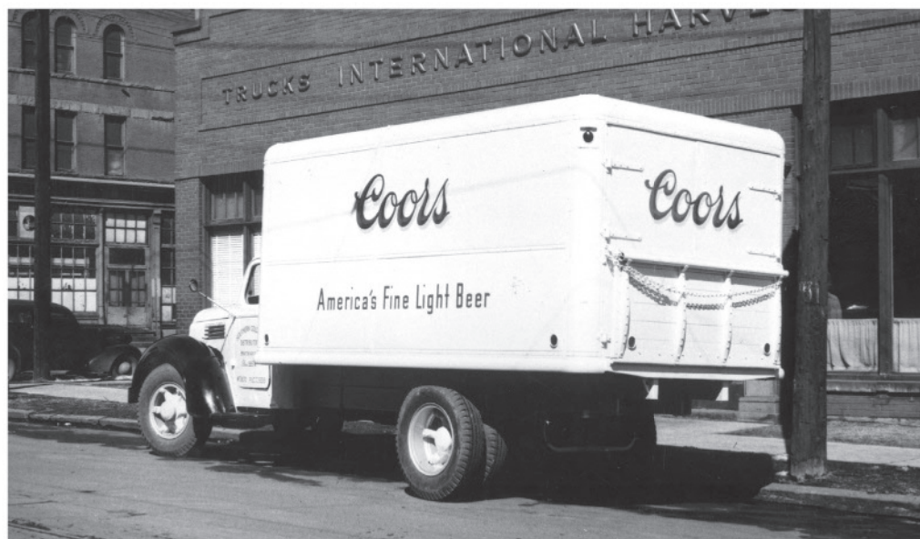
By the 1940s, Coors had invested in a fleet of refrigerated trucks like this one to ensure its unpasteurized beer stayed cold and fresh from brewery to backyard. Denver Public Library Special Collections. X-10018
