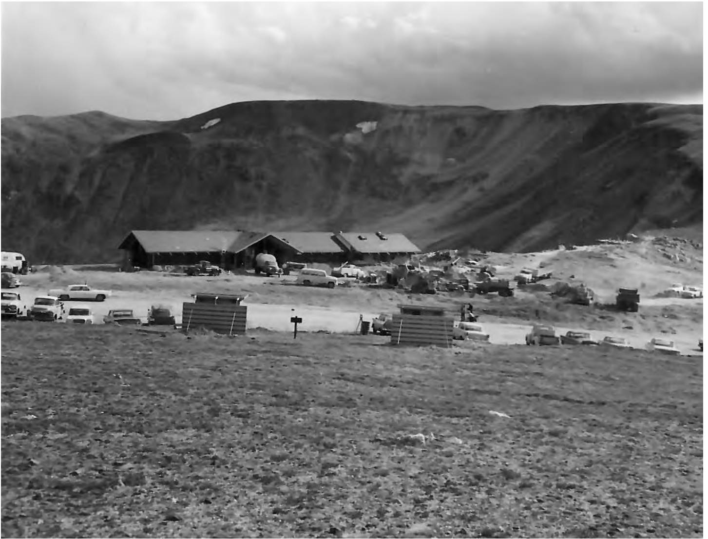
Figure 19 – Alpine Visitor Center under construction, September 1963 (Source: ROMO-11-Q-2-a, neg 4993)
