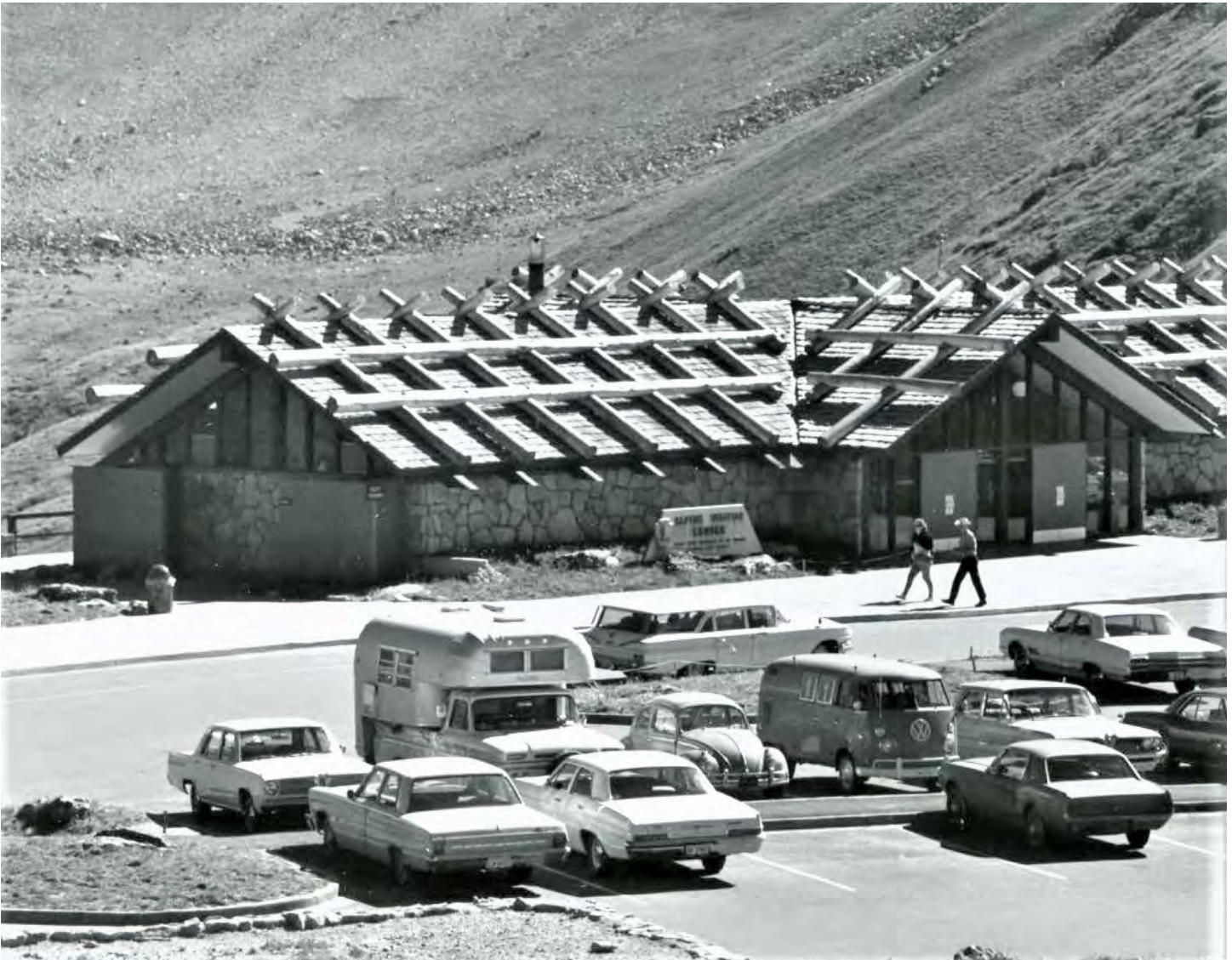
Figure 4 - Alpine Visitor Center Public Plaza c. 1970s (Source: ROMO_121_P7_ALPINE VISITOR CENTER) The photograph and architectural drawing (Figure 5) highlight one of the minor alterations to the Public Plaza. Both images show a small landscaped island with a few rocks and very low vegetation. It is not clear when the landscaped island at the corner of the Public Plaza was removed. However, it seems likely such formal landscaping proved difficult to maintain due to not only the large number of visitors but also the extreme weather conditions of the site.
