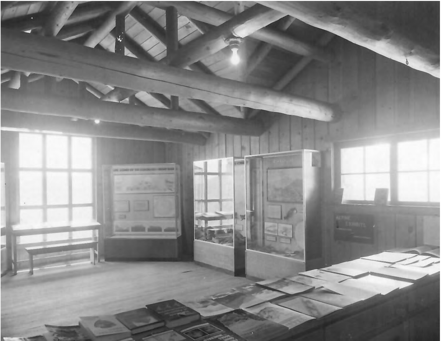
Figure 14 – Trail Ridge Store exhibits August 1958 (Source: ROMO-11-Q-2-a, neg 1122) After the Trail Ridge Store addition, exhibits were installed utilizing natural light. After the Alpine Visitor Center was constructed, the exhibits moved to that building, where they remain.
