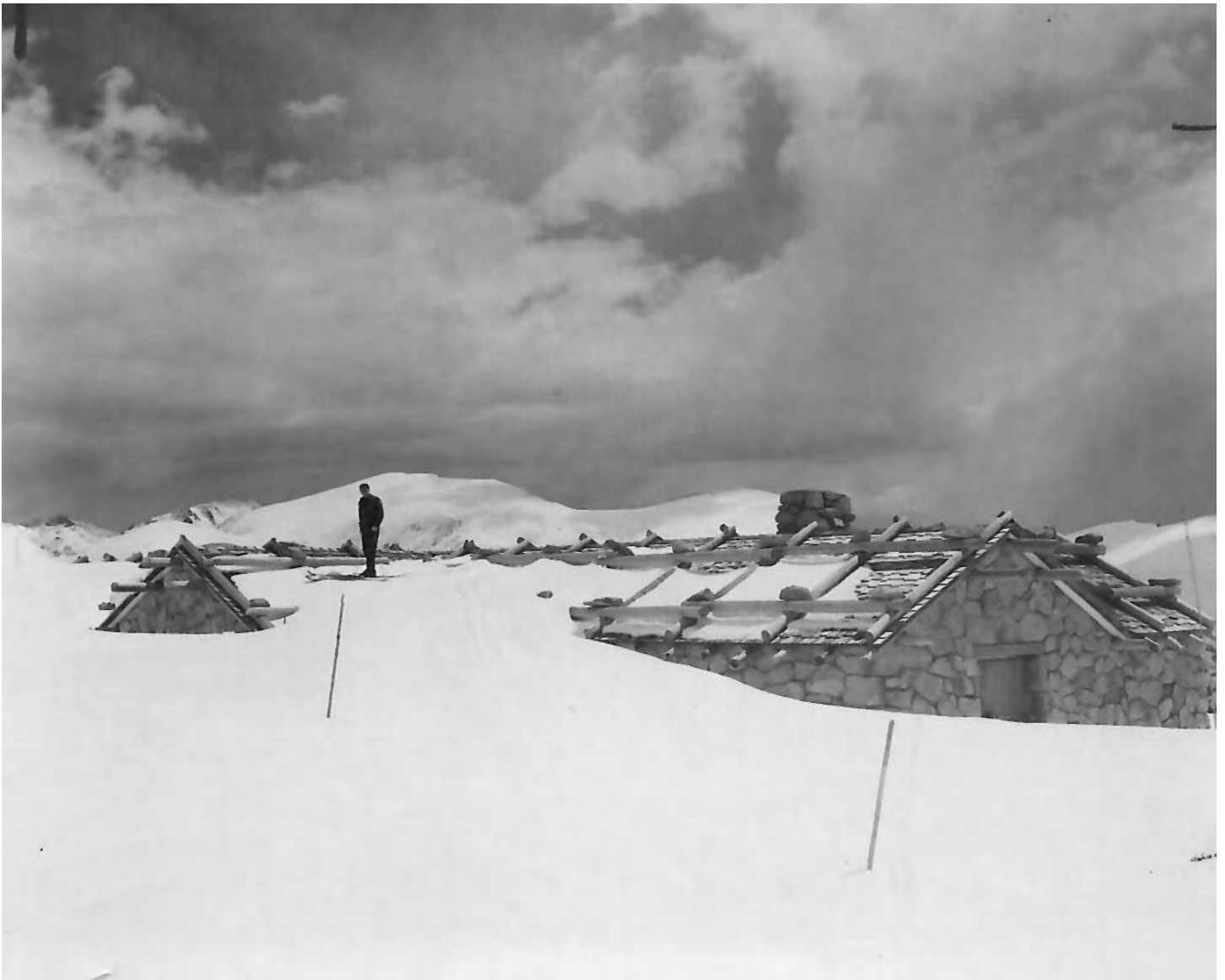
Figure 10 – Trail Ridge Store in May 1958 (Source: ROMO-11-Q-2-a, neg 5640)
