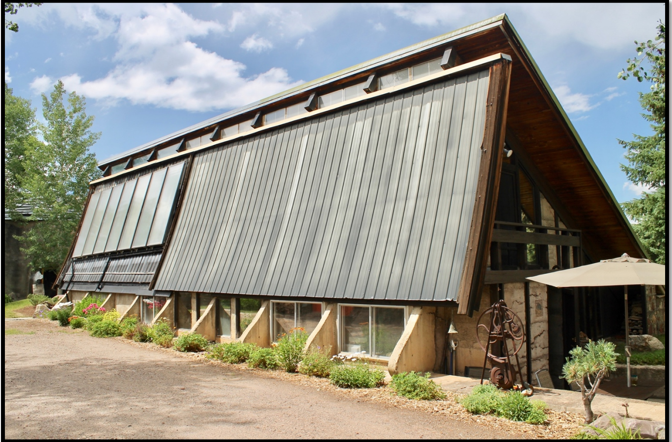
Photo 4: A-Frame Building, South Wall. View to the Northwest.
