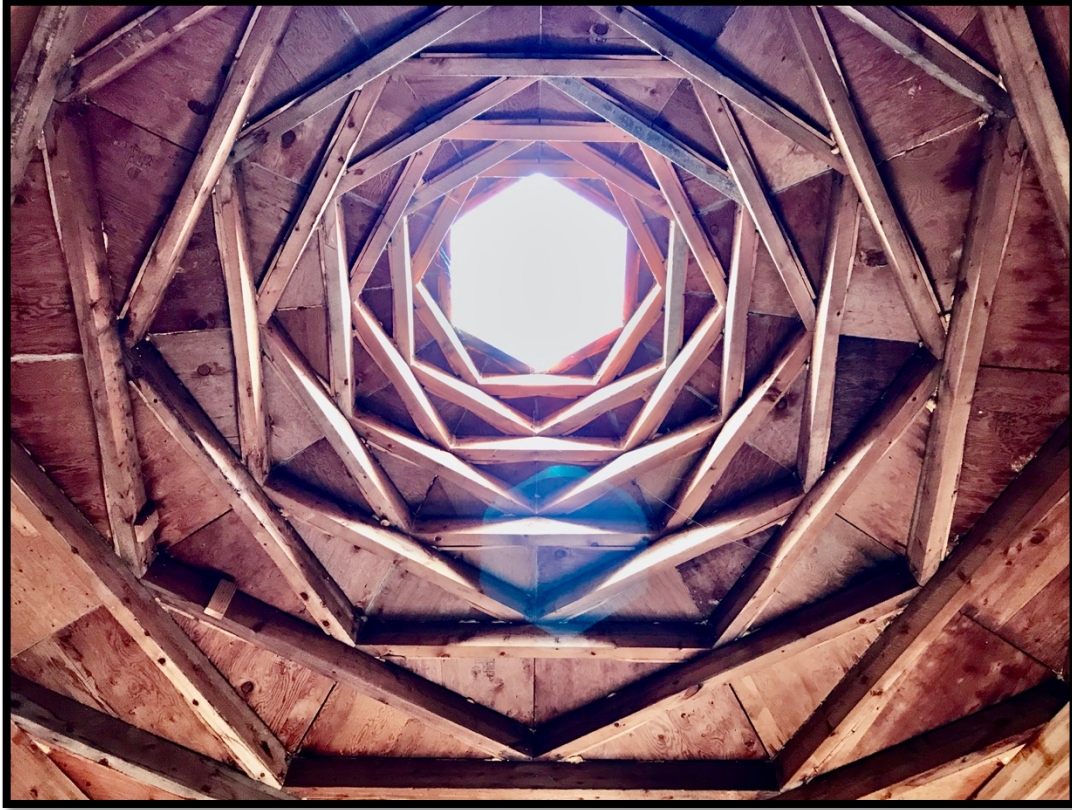
Photo 26: Round Building, Cribbed Roof Structure and Octagonal Skylight.
