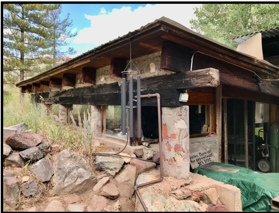
Photo 29: Studio Building, South Wall. View to the Northwest.
