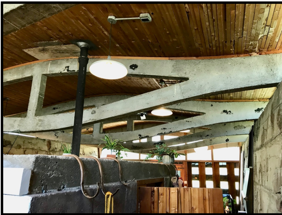
Photo 15: Orange Door Building, Interior Roof Structure. View to the South.
