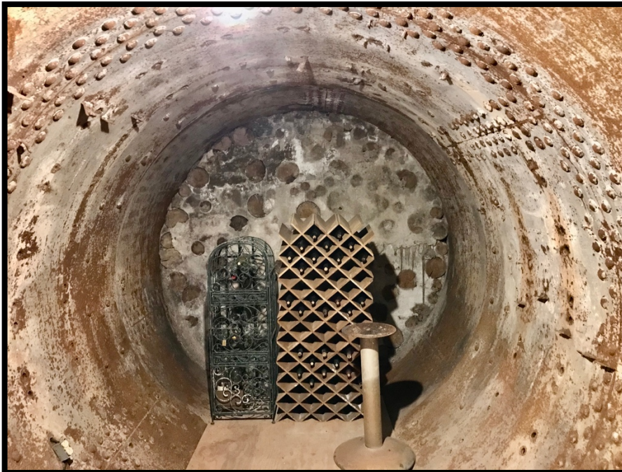
Photo 37: Wine Cellar, Lower Room (Lime Kiln Drum).
