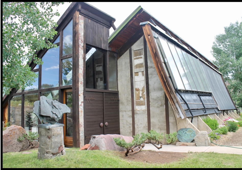
Photo 5: A-Frame Building, West Wall. View to the Northeast.
