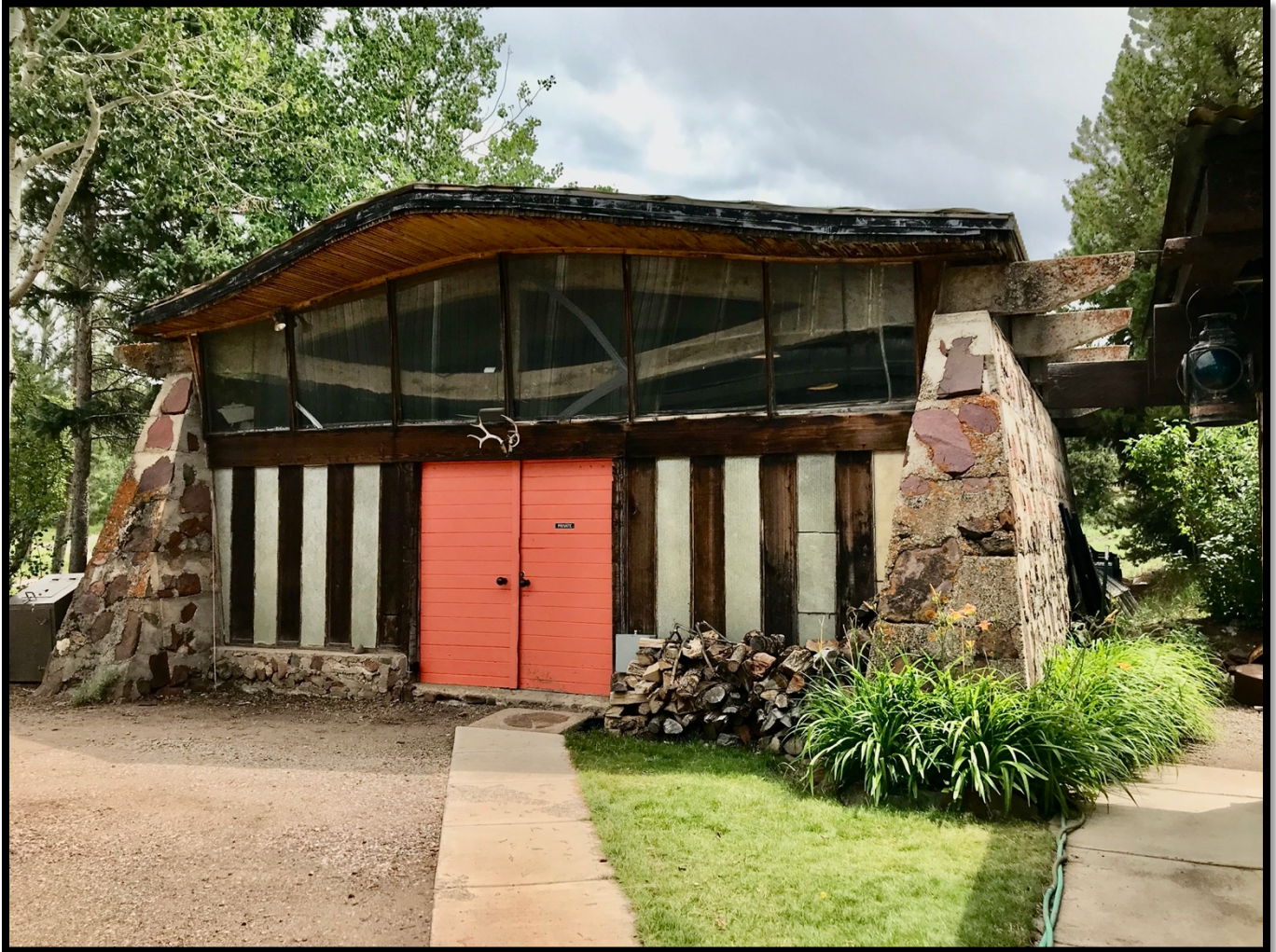
Photo 13: Orange Door Building, North Wall. View to the Southeast.
