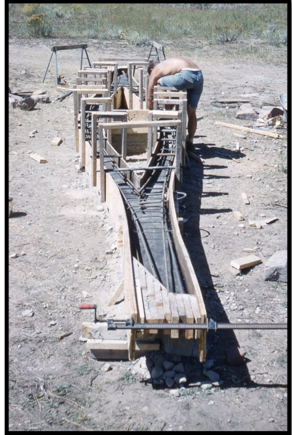
Photo 8 Orange Door Building Roof Truss Form 1958
