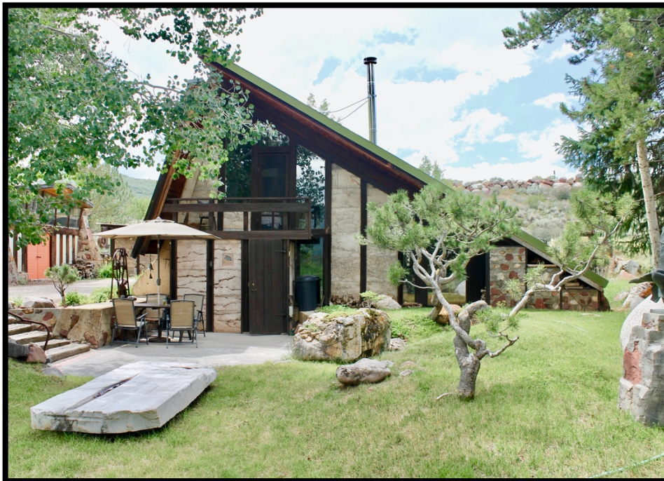
Photo 6: A-Frame Building, East Wall. View to the West.
