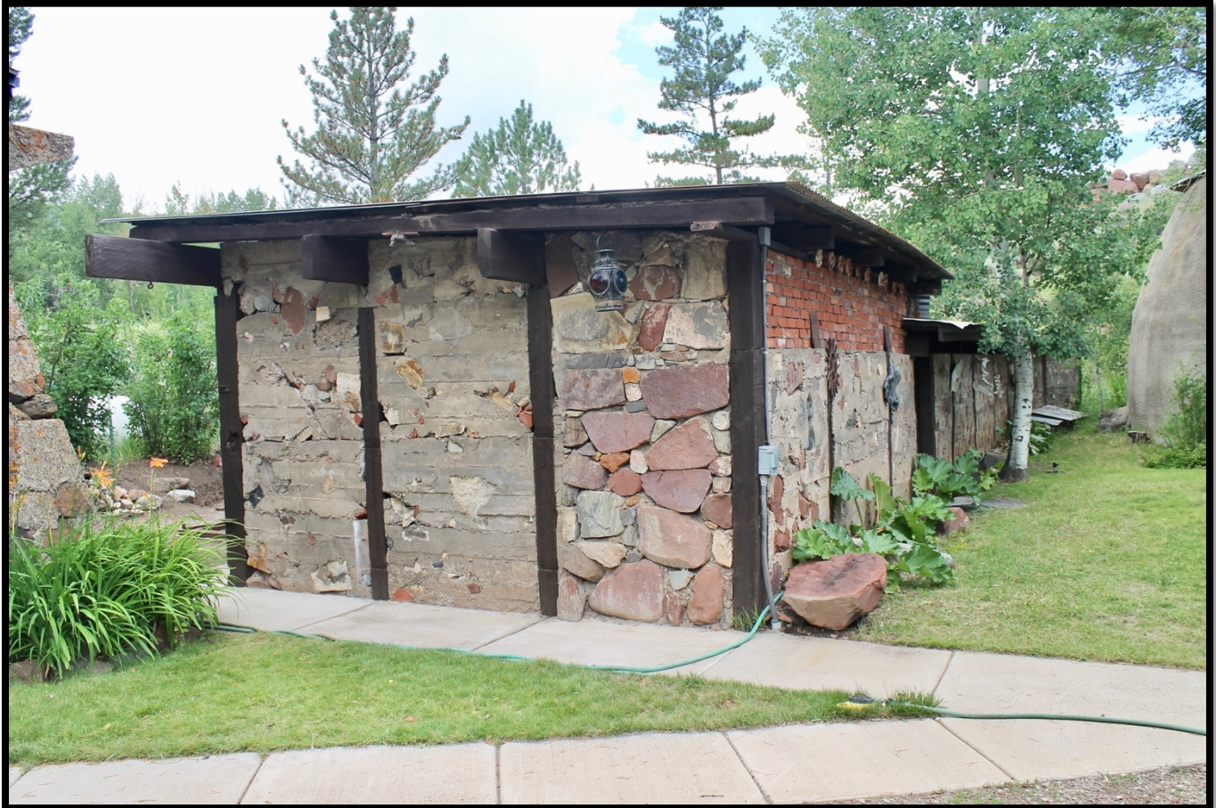
Photo 27: Studio Building, East Wall. View to the Southwest.
