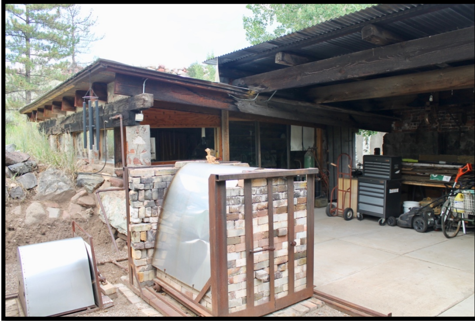
Photo 30: Studio Building, Outdoor Workshop with Kilns. View to the Northwest.
