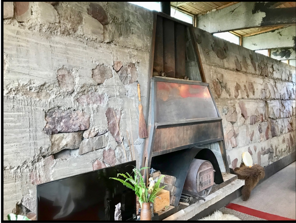
Photo 18: Orange Door Building, West Wall with Fireplace. View to the Northwest.
