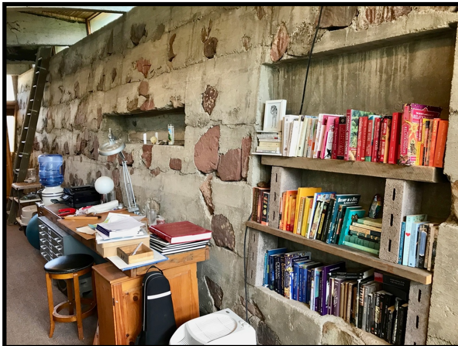
Photo 17: Orange Door Building, East Wall. View to the Northeast.
