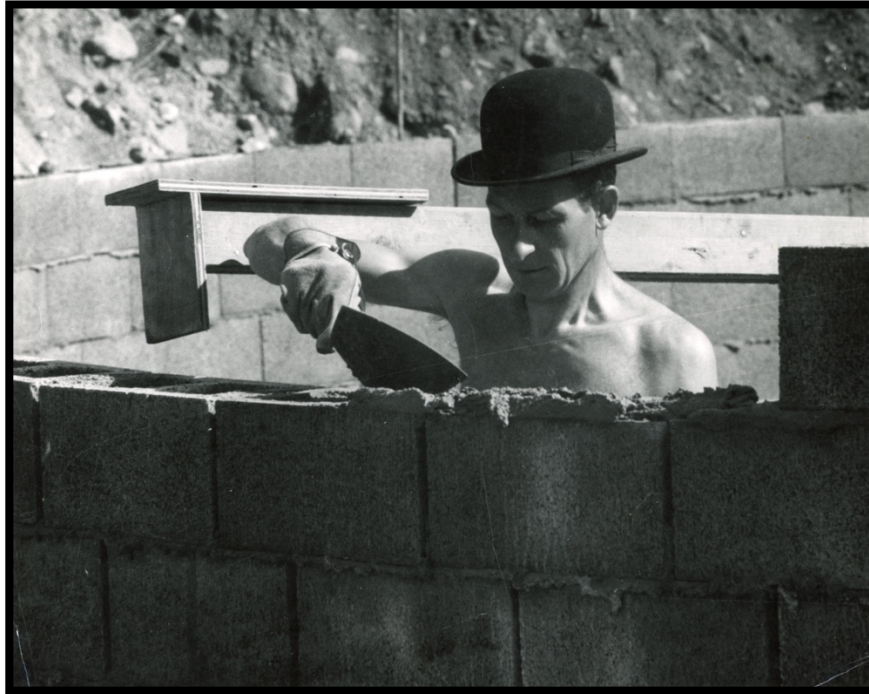
Photo 15: Paul Soldner Laying Concrete Blocks for the Round Building, circa 1966. From the Collection of the Soldner Family Partnership LLLP.
