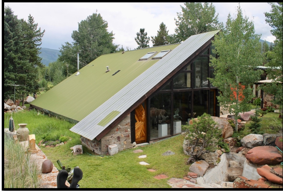
Photo 7: A-Frame Building, North Roof and West Wall. View to the Southeast.
