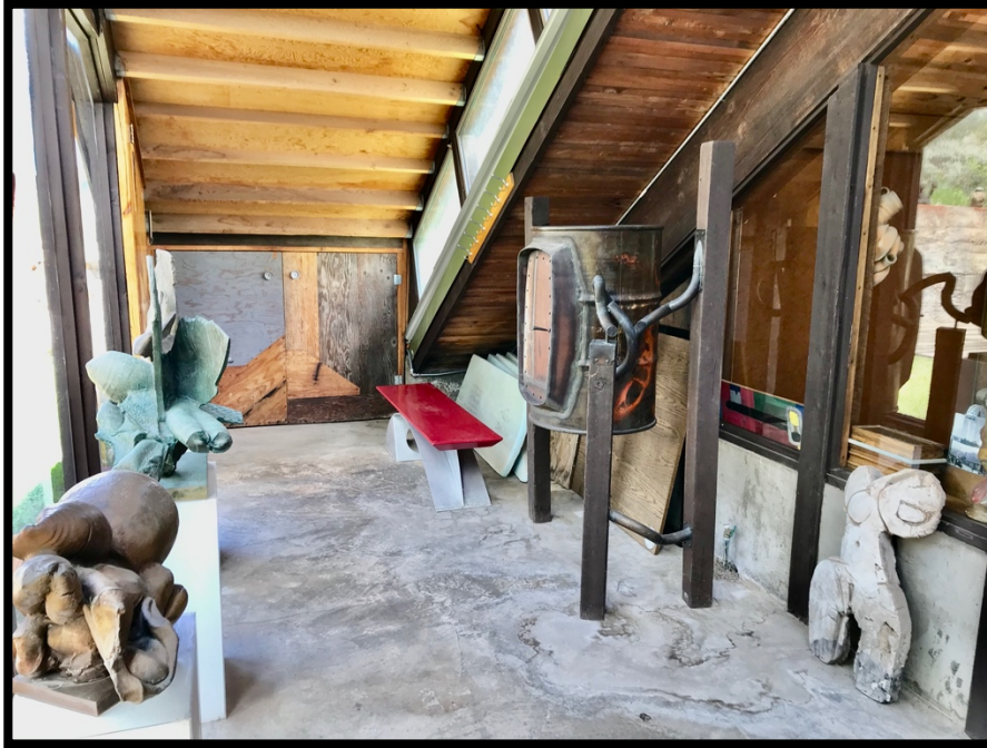
Photo 11: A-Frame Building, West Addition. View to the North.
