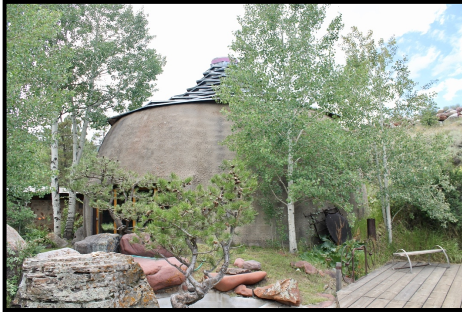
Photo 20: Round Building. View to the Southwest.
