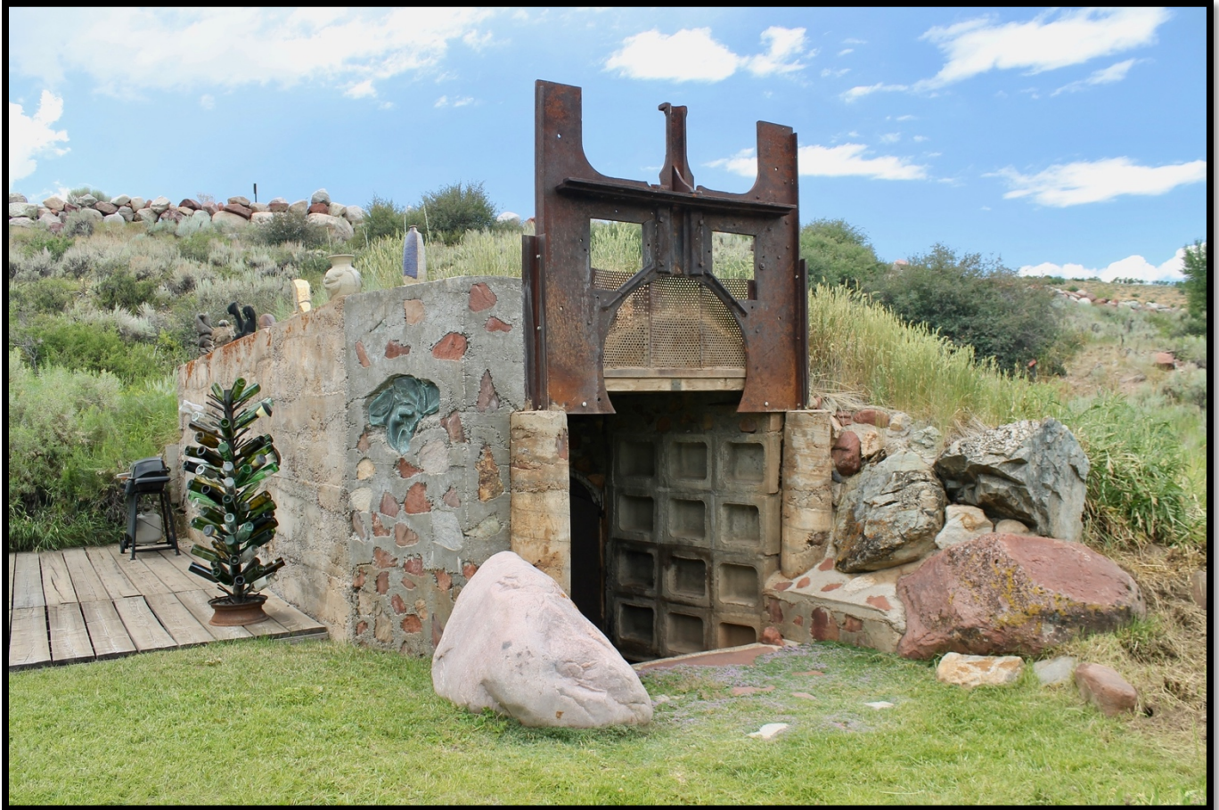
Photo 35: Wine Cellar, East Entrance. View to the Northwest.
