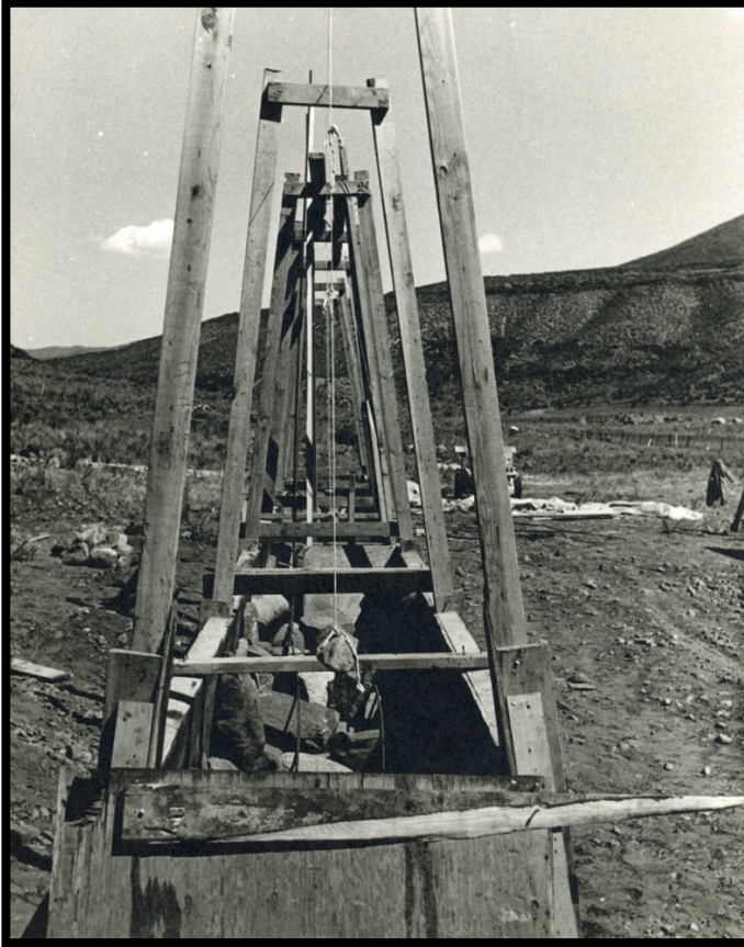
Photo 7 Orange Door Building Slip-Form Concrete Wall Frame 1957
