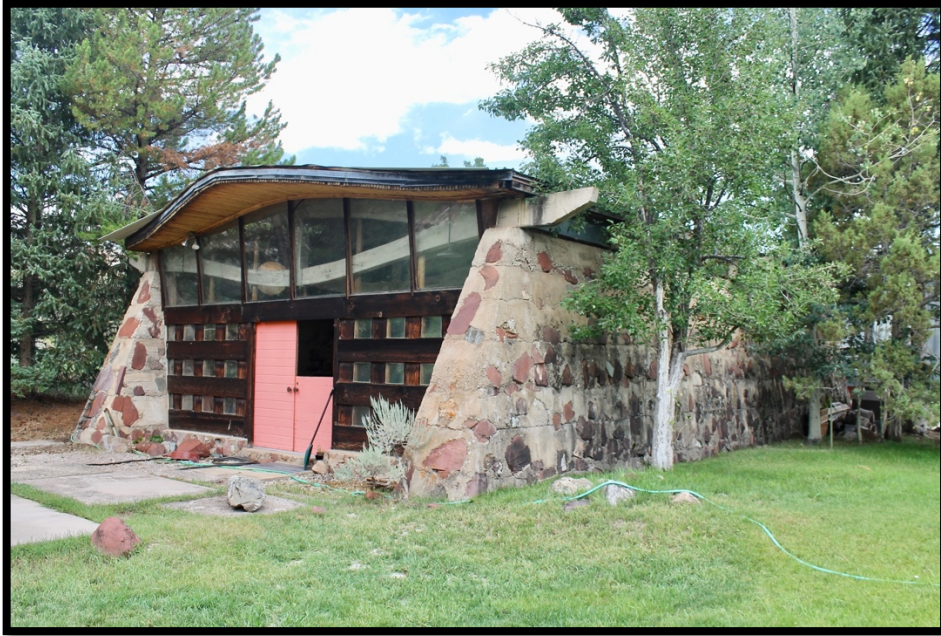
Photo 14: Orange Door Building, South Wall. View to the Northwest.
