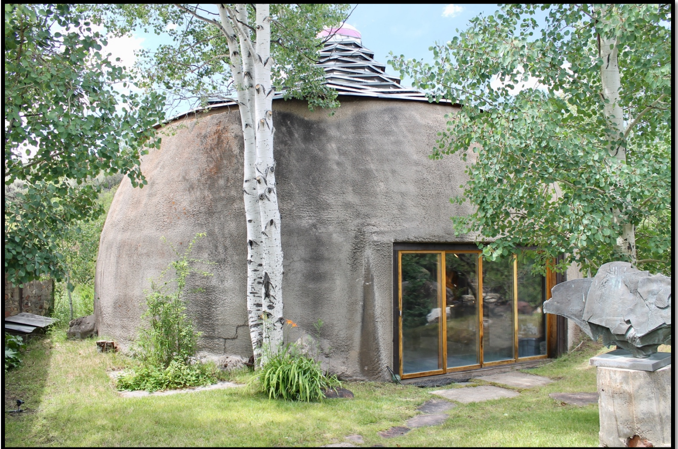
Photo 19: Round Building. View to the Northwest.
