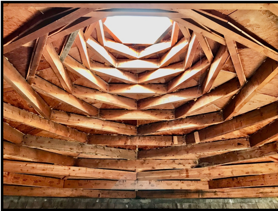
Photo 25: Round Building, Roof Structure.
