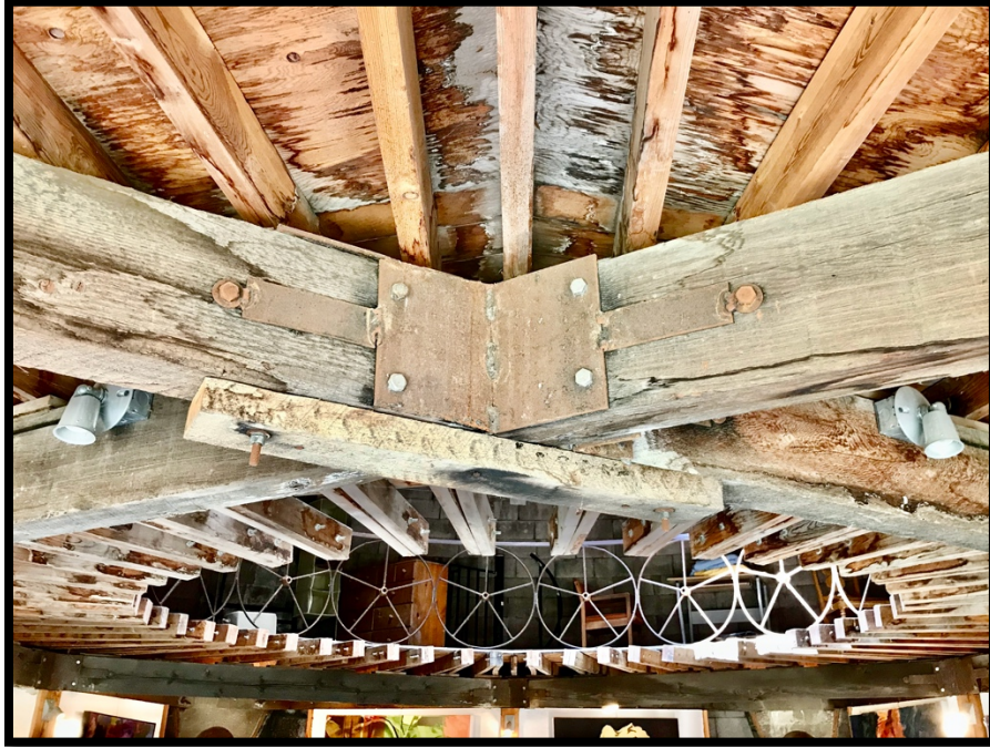
Photo 24: Round Building, Cantilevered Loft Structure from Below.
