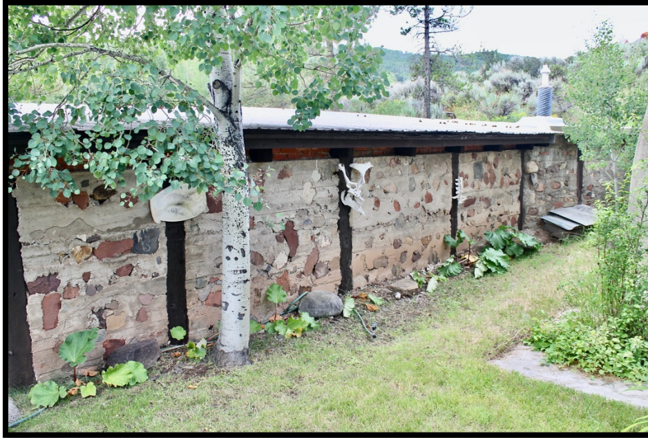
Photo 28: Studio Building, North Wall. View to the Southwest.
