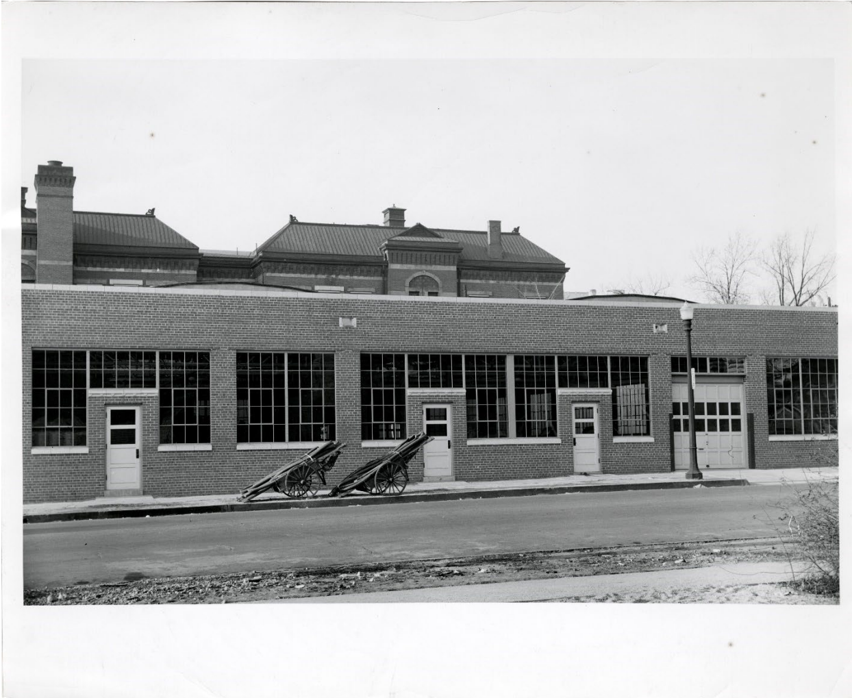
Historic Photo 4: 1941 photograph of the exterior of the Emily Griffith Opportunity School Shop building built in 1941.
