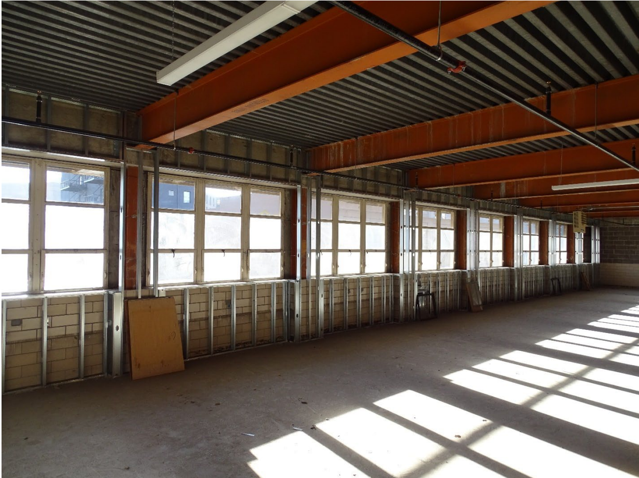
Photo 21: 1956 KRMA building Interior (Second Floor) – South Facing. 21 of 32 .
