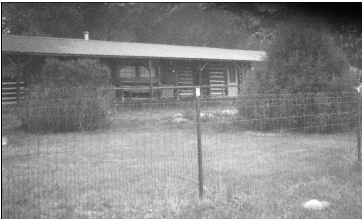
Figure 4. The east wall of the bunkhouse is pictured in this ca. 1980s assessor appraisal card image (view west). SOURCE: Chaffee County Assessor, Salida, Colorado.
