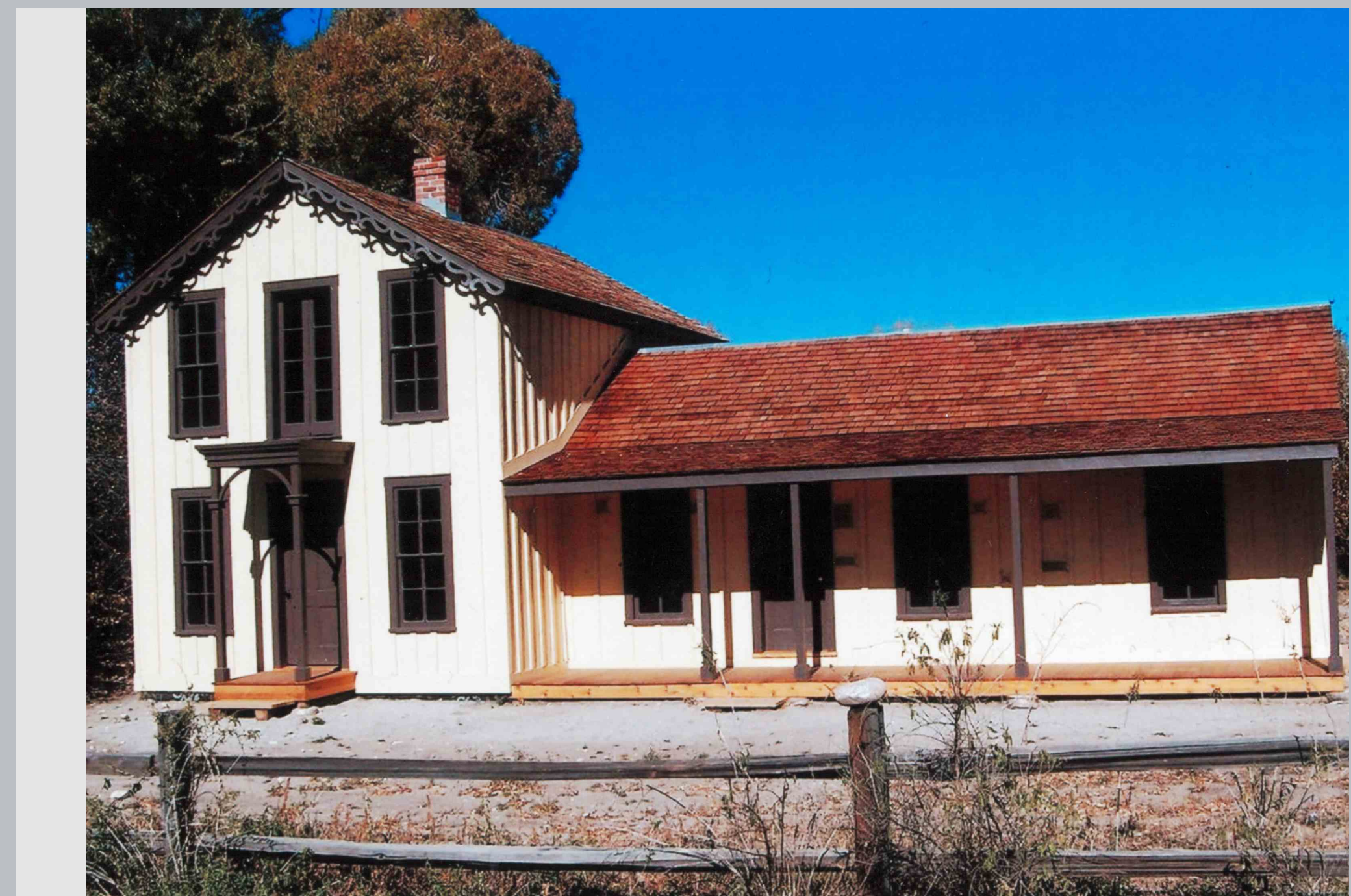
Photos: Top New interpretive panel Bottom, Rehabilitated homestead (2013)
