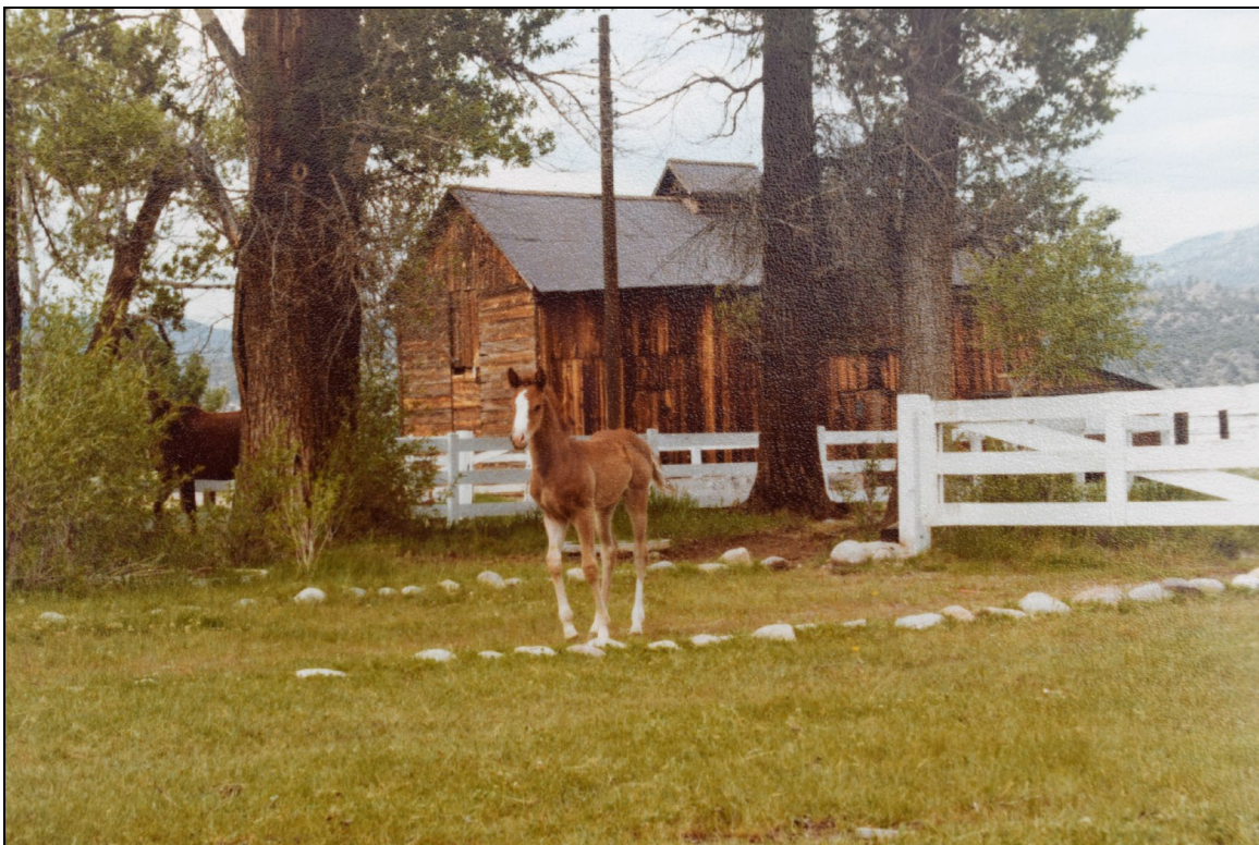
Figure 2. The front and west walls of the barn are visible in this ca. 1980s photograph (view northeast) taken from the pasture to the southwest. SOURCE: Nancy Roberts, Nathrop, Colorado.
