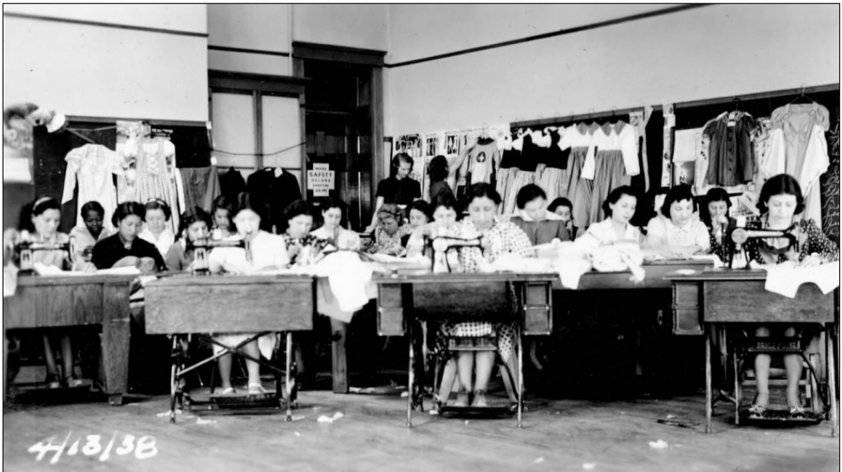
Figure 9. During the Great Depression, the Works Projects Administration and National Youth Administration conducted projects in the building. This 1938 photograph shows sewing participants engaged in making costumes for theater plays. SOURCE: image number PH-AAA-0034, April 13, 1938, Pueblo City-County Library, Pueblo, Colorado.
