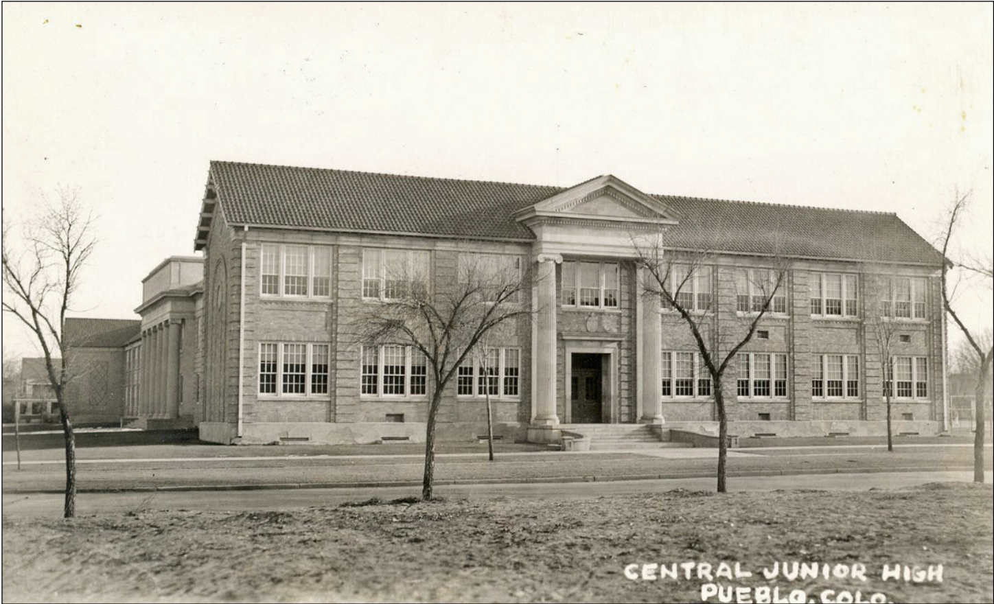
Figure 8. This ca. early to mid-1930s view shows the west wall of the school with the front to the left. SOURCE: N/A.
