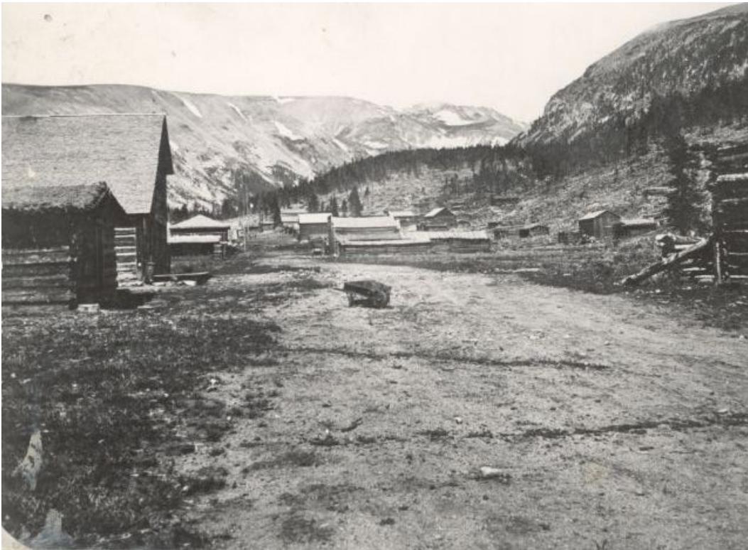
Figure 1: An 1864 photograph of Buckskin Joe, the first Euro-American settlement in the Alma area, which flourished in the 1860s before its abandonment ca. 1868, documents several representative examples of Pioneer Log buildings of various size and form.
