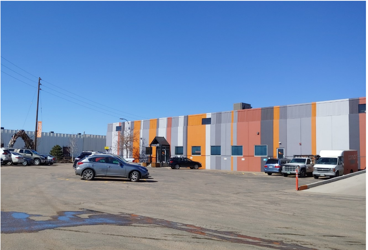
Figure 5. Photograph (February 2020) showing southwest corner of warehouse additions to CB&Q Shops machine shop building. Camera facing northwest.
