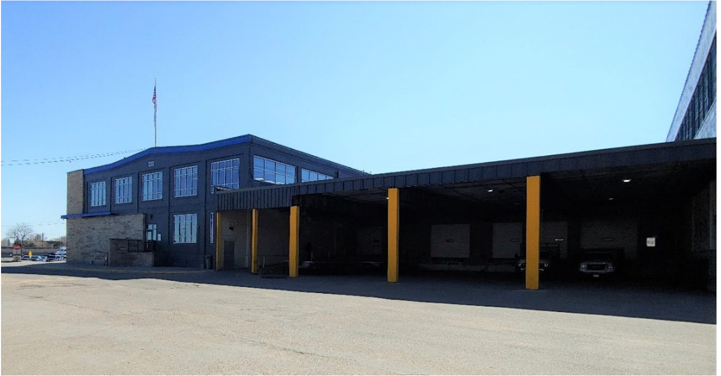
Figure 7. Photograph (February 2020) showing former Office and Storehouse (at left) and addition connecting to Machine Shop (at right). Camera facing south/southeast.
