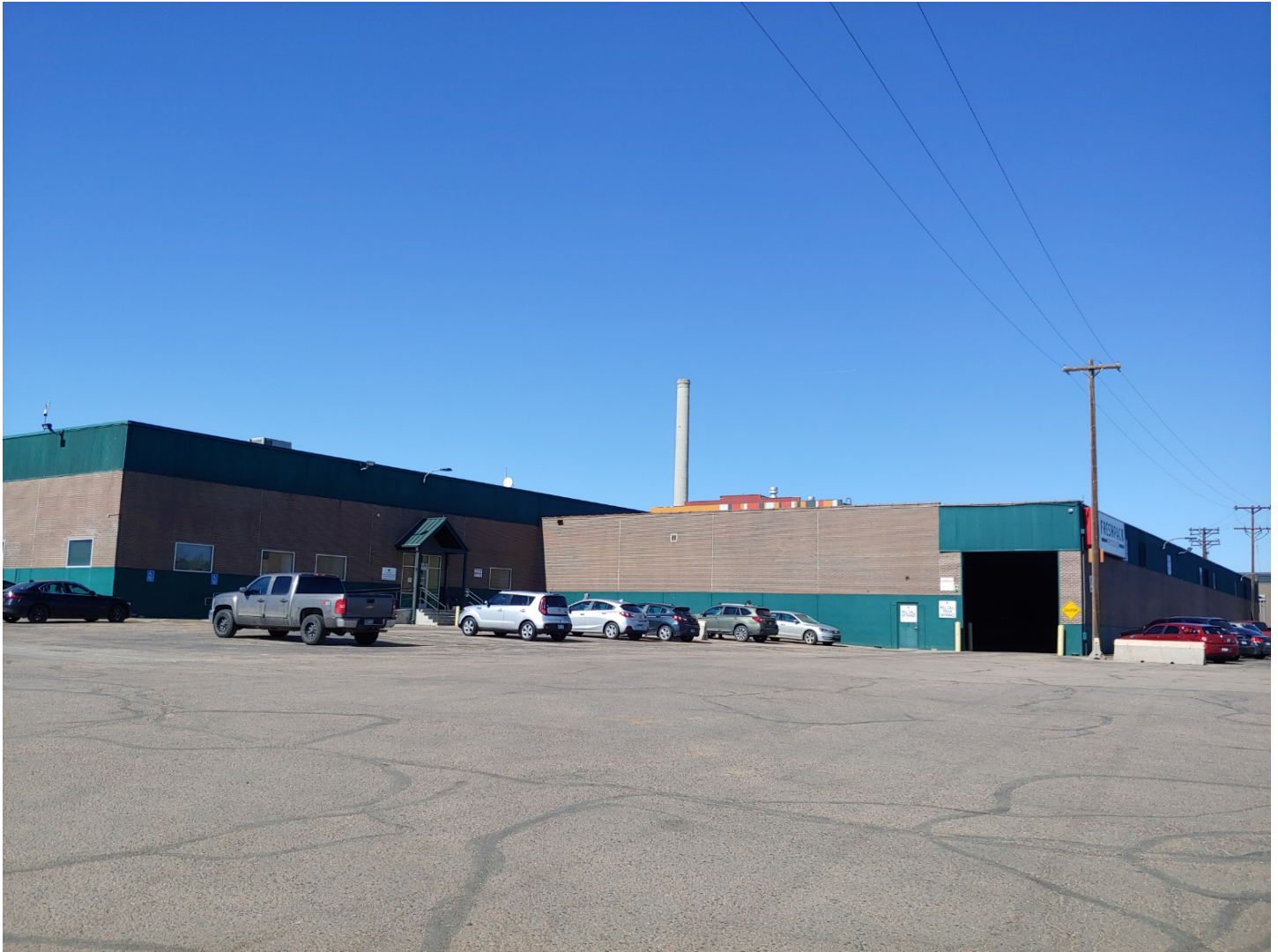
Figure 4. Photograph (February 2020) showing southeast corner of warehouse additions to CB&Q Shops office and machine shop buildings. Note concrete Chimney of Powerhouse beyond. Camera facing north/northwest.
