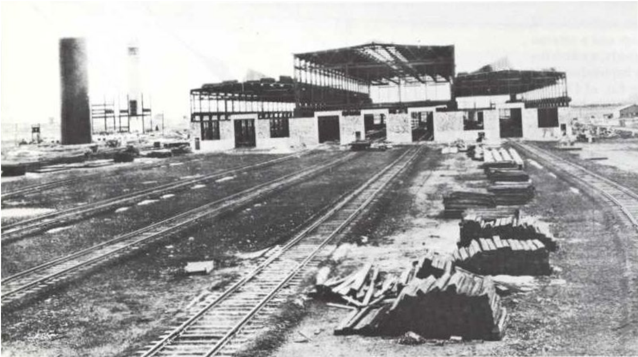
Historic Photo 3. Construction of Machine and Erecting Shop (center) and Powerhouse (left), late 1922, looking north. Reproduced in "Denver Locomotive Shops" Burlington Bulletin (July 1982) by F. Hol Wagner, Jr., with credit given to Denver Public Library Western History Department (unable to confirm call number).
