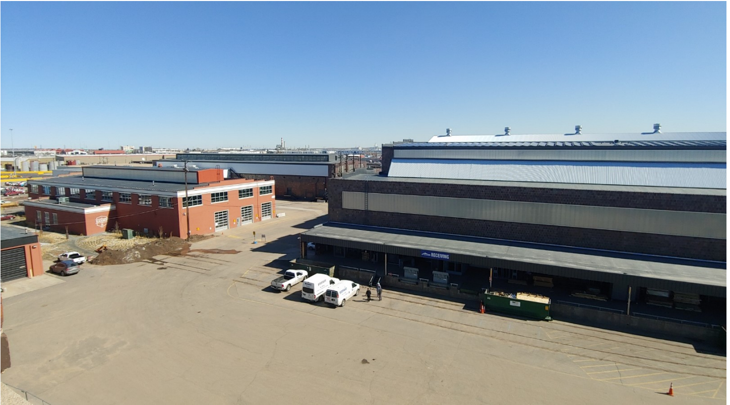
Figure 6. Photograph (February 2020) showing former Machine Shop (at right) and Blacksmith building (at left). East additions to Boiler Shop beyond (center background). Camera facing northeast.
