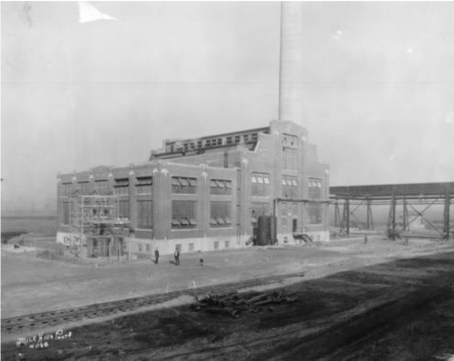
Historic Photo 6. CB&Q Denver Shops Powerhouse, looking northwest, ca. 1923, by Mile High Photo Company. Courtesy Denver Public Library Western History and Genealogy Department (call number Z-6016).
