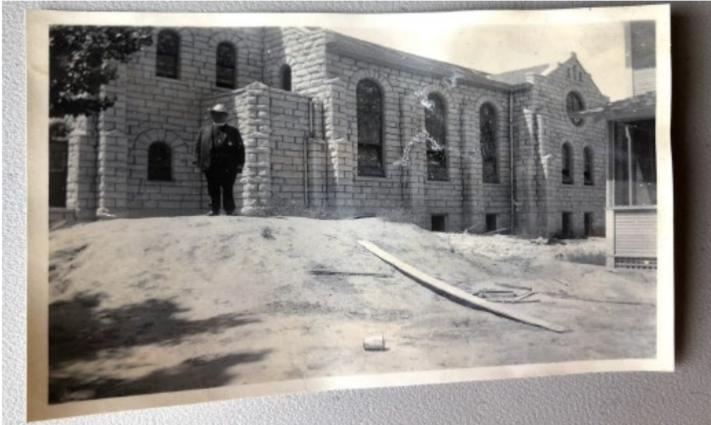
Photo H1. Sacred Heart Church as seen from SE corner of building, ca. 1922
