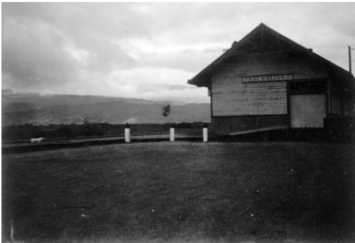
Figure 10: West wall of depot ca. 1940s. (Denver Public Library, X-11044).
