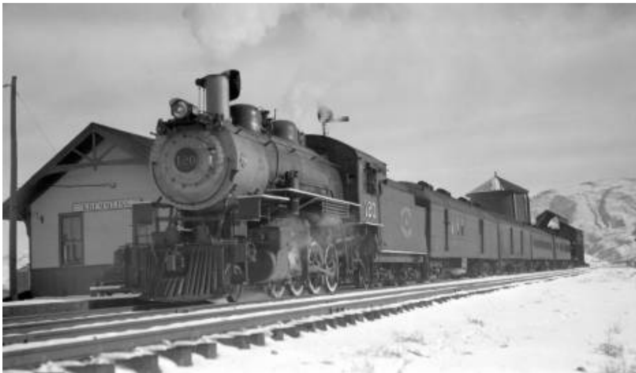
Figure 9: East wall of depot in 1933. (Denver Public Library, OP-11243)
