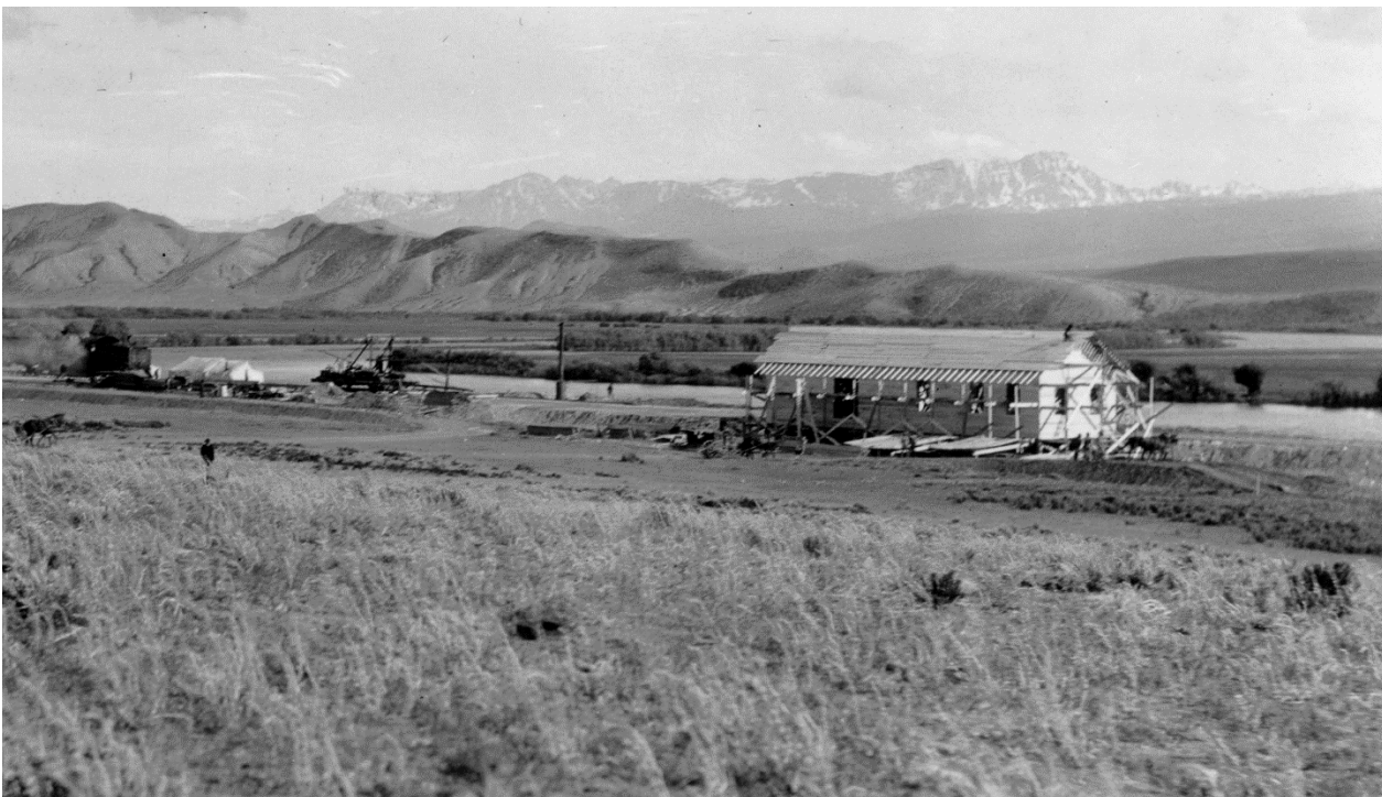
Figure 2: Depot under construction in 1906. (Denver Public Library, Z-5693)
