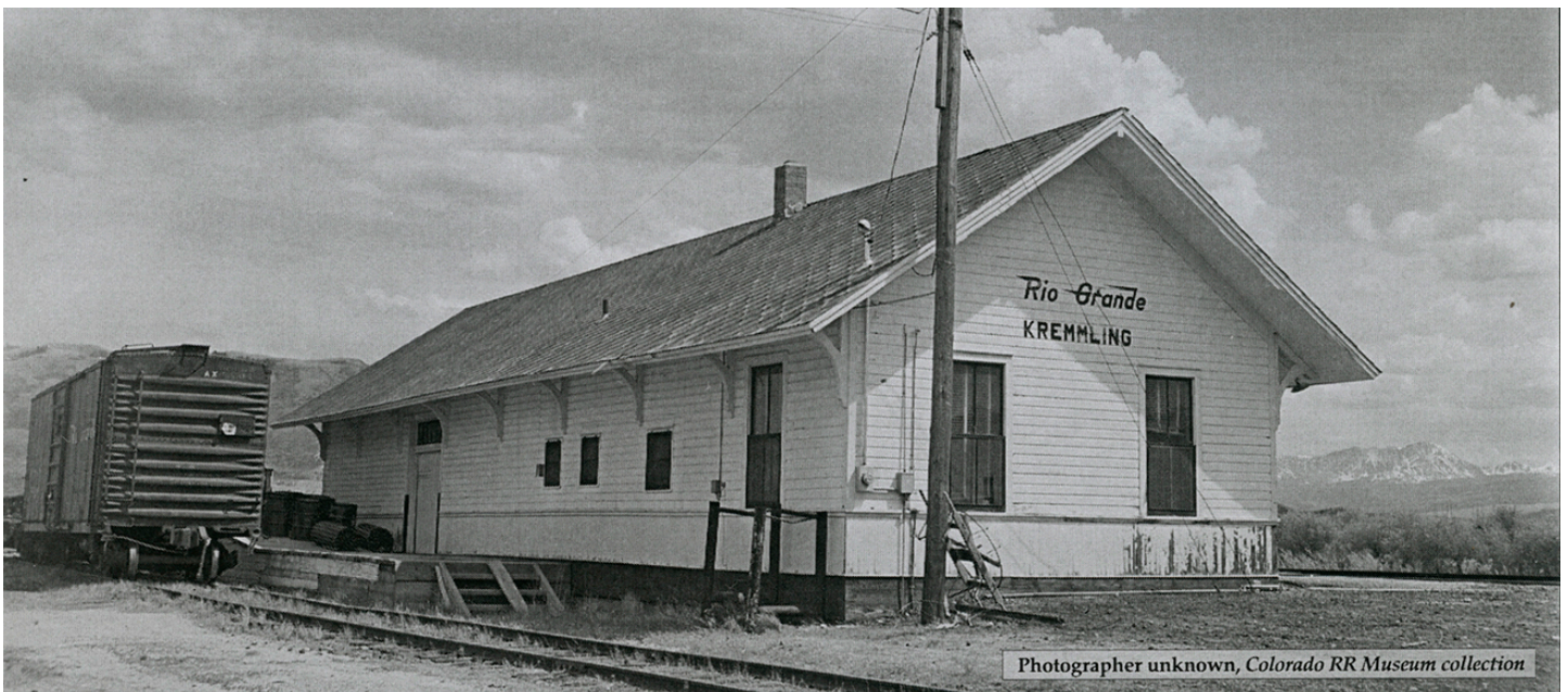
Figure 12: South and east sides after the 1954 renovation. Note changes to fenestration on south wall. (Colorado Railroad Museum Collection/ Corona Telegraph , Vol. 10, No. 2).
