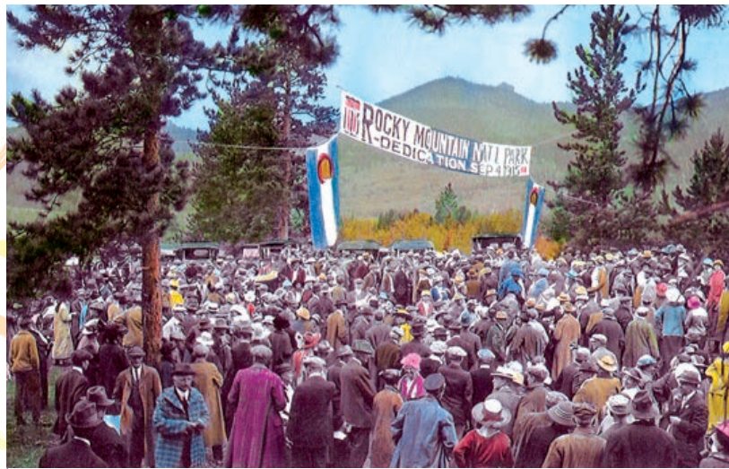
Photo courtesy Jim Pickering
